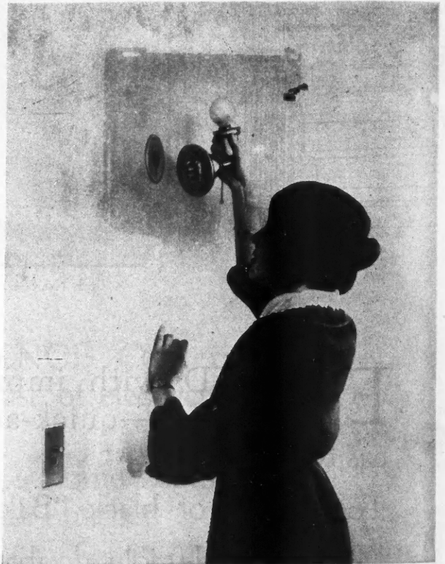
Fig. 3. With the Elexit Outlet the Lighting Unit Can Be Removed at Will.
