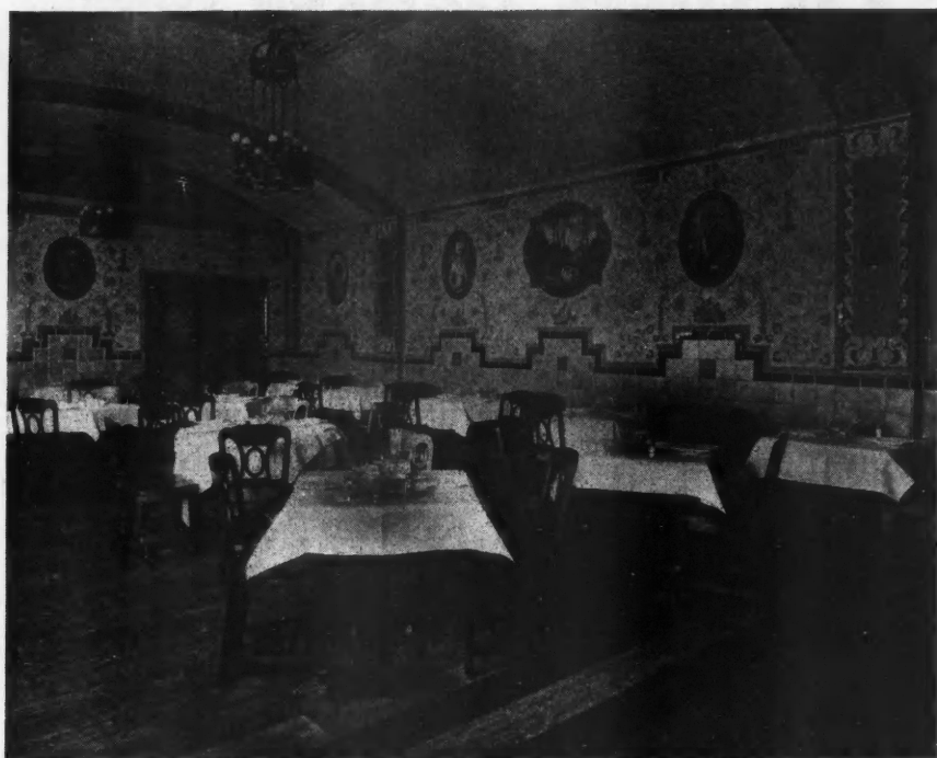
The Cement Base Paint Applied to the Walls and Ceiling, Overtone with Oil Colors, Pershing Square Cafe, New York, John J. Petit, Architect.
