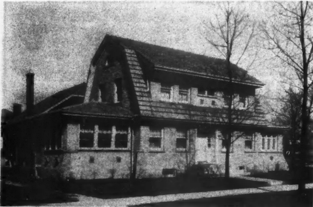
Demand for a Colorful Fireproof and Permanent Roofing Material Has Led to the Development of Concrete Tile for This Purpose, Used on the Home Shown Here. Recent improvements in machinery for making this product indicate that its manufacture is a coming enterprise.
