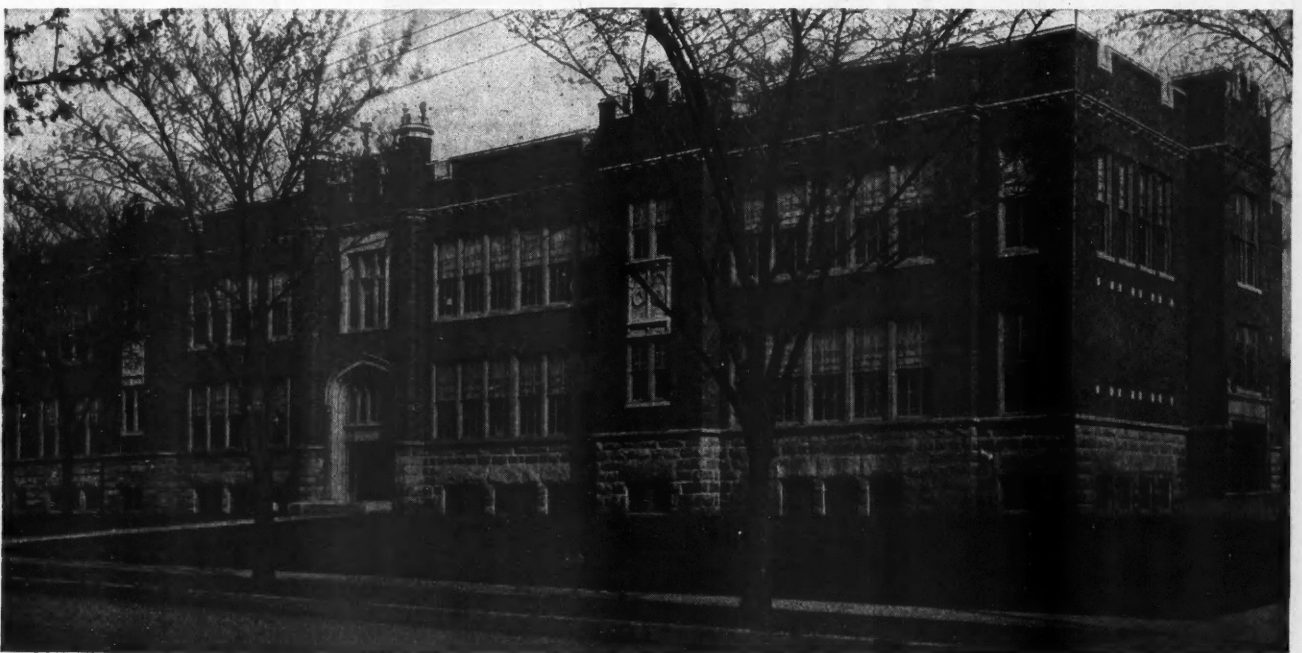
The Wright School, Rockford, Ill., is Typical of Modern School Construction in the United States. The exterior is veneered with a rough texture face brick and trimmed with terra cotta. Peterson and Johnson, Architects.
