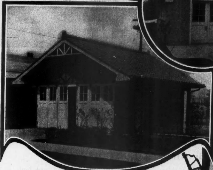
The Tile Roof of This Brick and Stucco Garage Will Strike a Common Note with the House for Which It Is Built.
