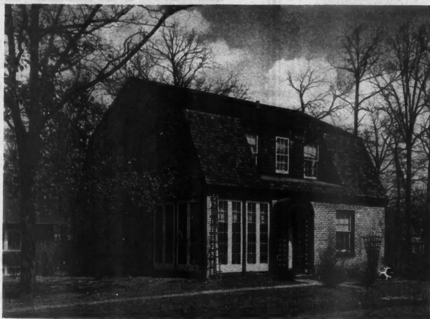
Common Brick Has Attained a Widespread Popularity as a Building Material in Many of Chicago's Residential Suburbs. Often the homes are painted with paints made especially for brick. The H. W. Branigar residence, 421 Oakwood avenue, Highland Park, Ill., was designed by C. Reinhardt, architect.
