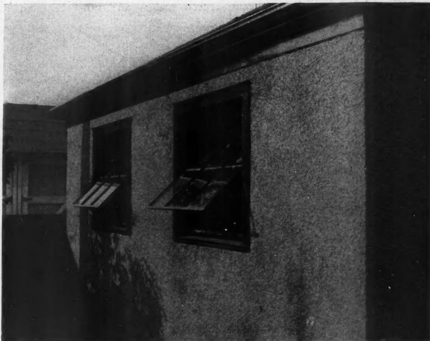
A Good Example of Stucco Work on This Garage.
