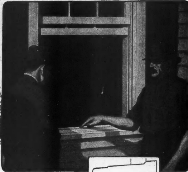
The double shoulder on the sill makes the Andersen Frame waterproof and windproof.
