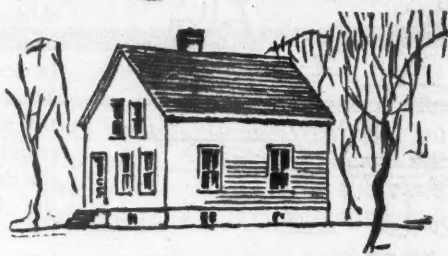
Front and Right Side of Old House.
