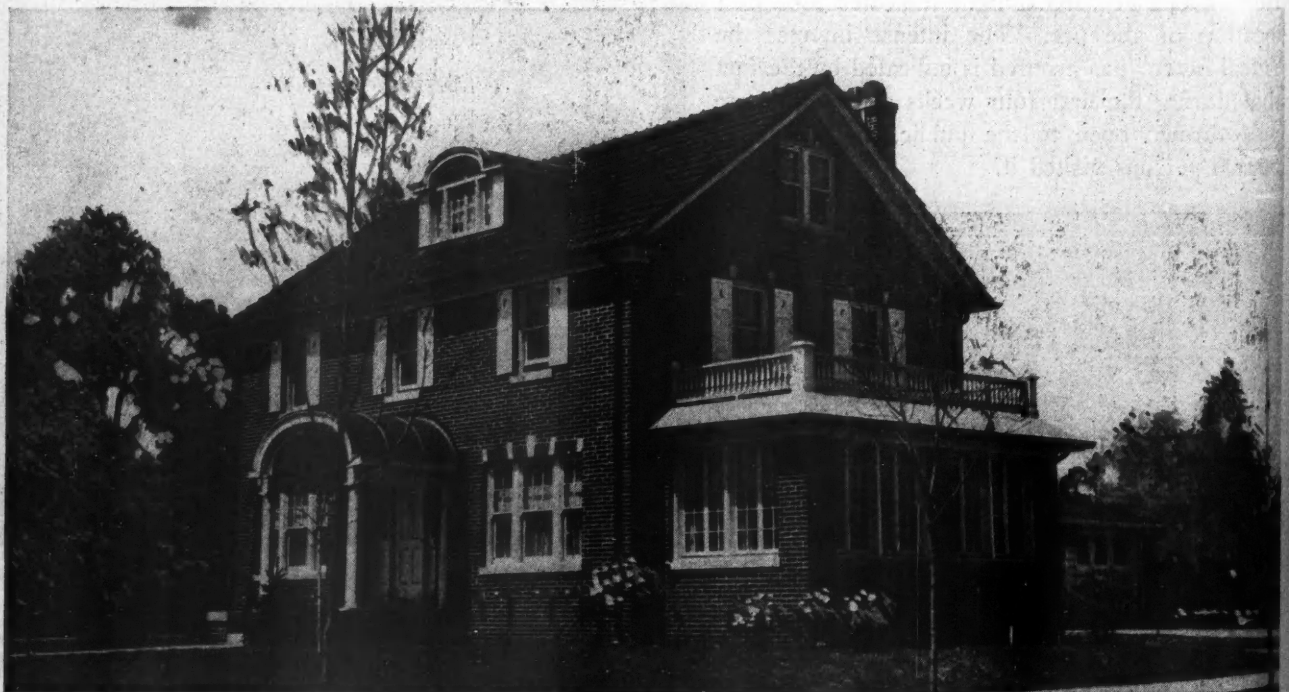
Care Was Expended to Make This Colonial Home Perfect in Its Construction Details. The exterior is of wire cut face brick, with a tile roof. Note the generous number of bathrooms in the floor plans, which show the convenience of the home.
