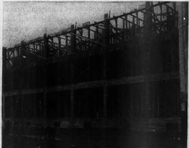
Ordinary Construction, Showing Multiplicity of Wood Supports.
