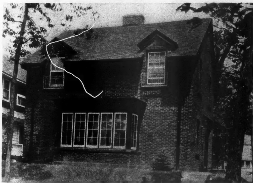
A Modern Home of Brick Is of Such a Permanent Nature That It Is Almost Impossible to Tell Whether It Is Five or Twenty-five Years Old. If the design is right, age will add the beauty of dignity to the residence. Where homes represent the savings of a lifetime, this quality of permanence is especially desirable.
