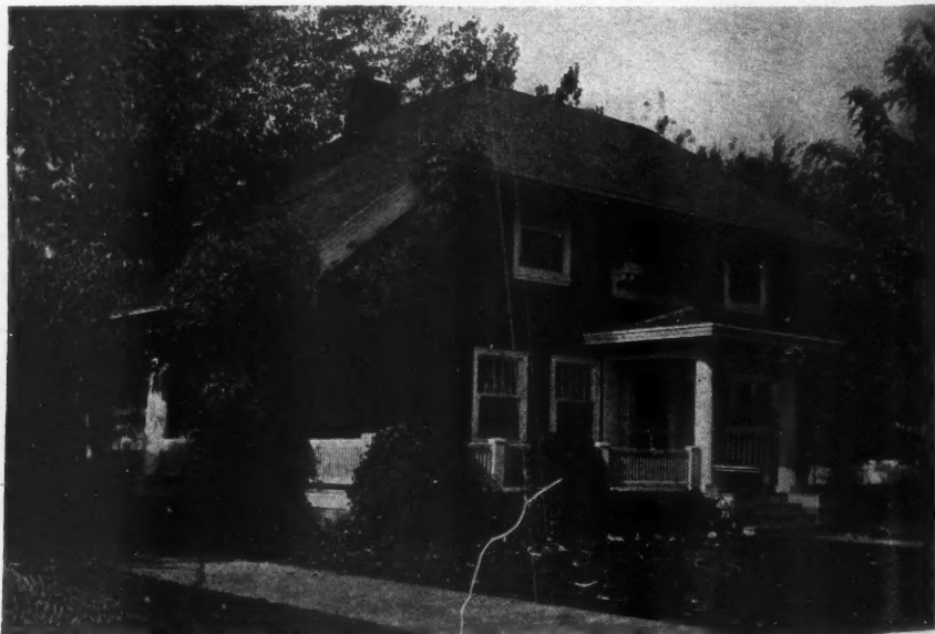
The Attractive Shingle Covered Frame House Shown Here Was Designed by E. Crawford, of Walla Walla, Wash.
