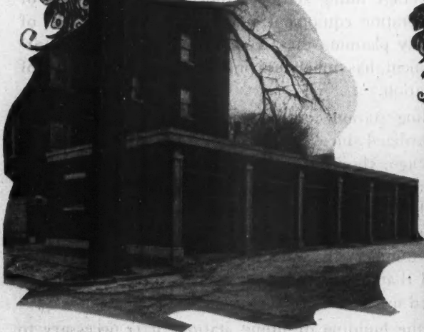
Shelter for the Automobiles of Apartment Dwellers Often Presents a Difficult Problem. A practical, convenient and attractive solution is shown above.
