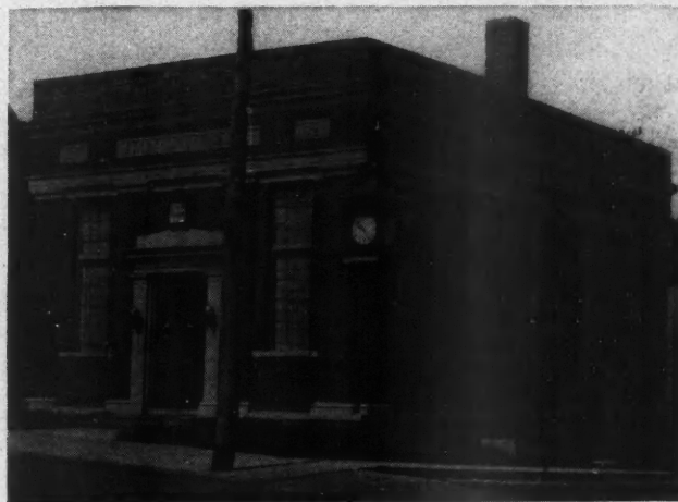
The Exterior of the First National Bank of Coopersburg, Pa., Is Pleasing in Its Dignified Simplicity. The exterior is of rough, red, face brick, laid in white mortar. The trim is of cast stone.
