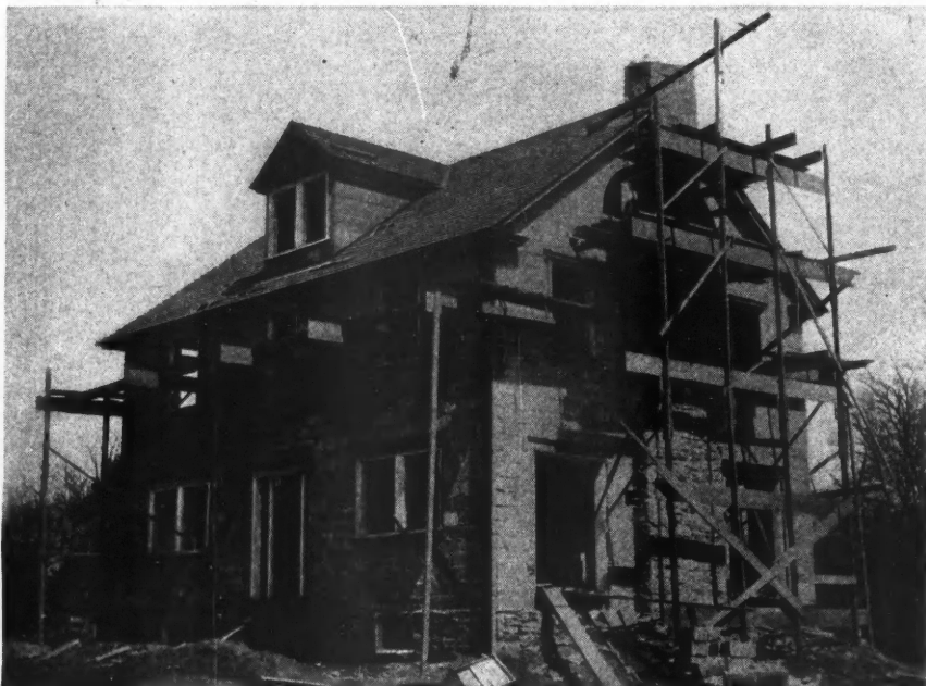
Concrete Blocks Ready for Stucco Finish.
