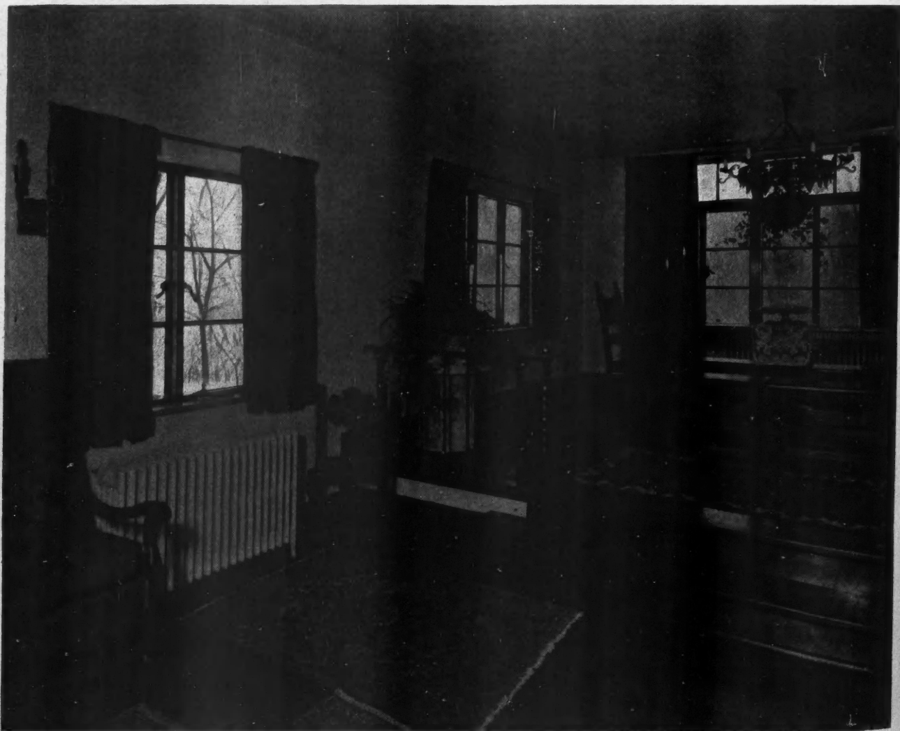
The Living Room and the Dining Room of the Home Are Enclosed in the Same Four Walls, the Portion Used for the Dining Room Being Raised Two Steps Above the Living Room Level as Is Shown in This Illustration. Broad plastered surfaces in sand finish are practical when metal lath is used to prevent cracks and avoid dust marks.
