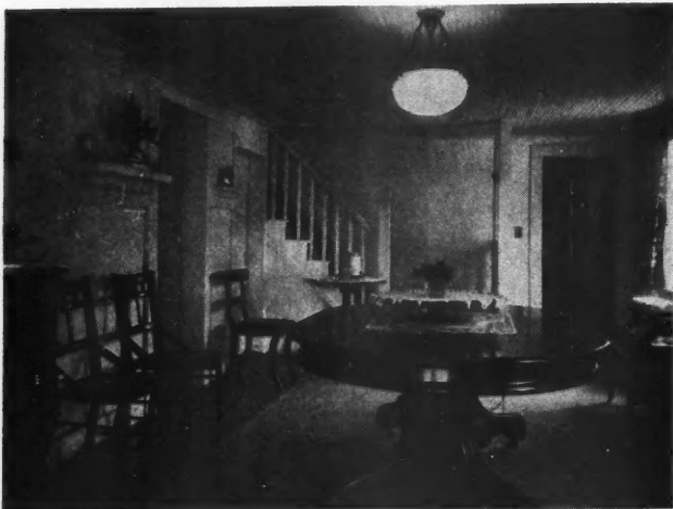
Fig. 4. The Small Bowl with Narrow Top Opening Hung Close to the Ceiling Is Not an Efficient Unit.
