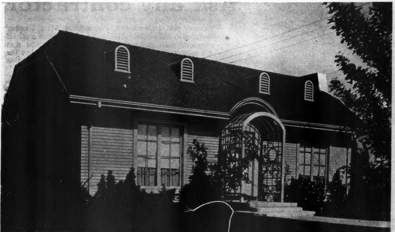
Nowhere Is Proper Wiring More Important Than in Small But Attractive Homes Like the One Shown Here. Full details of proper wiring for this bungalow will be found on page 144.
