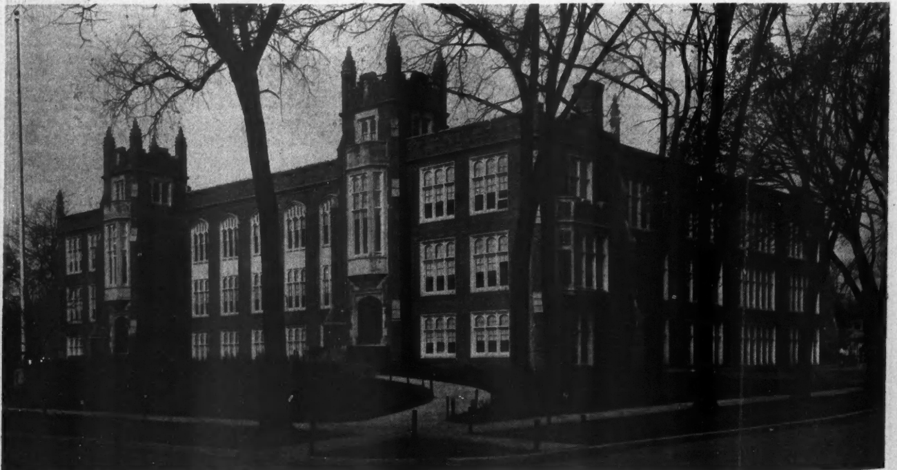
The Cossitt Avenue School, La Grange, Ill., Has Been Called the "Finest Grade School in America." The building is of reinforced concrete with the exterior of varicolored face brick. The architecture is Tudor Gothic. Childs and Smith, architects.
