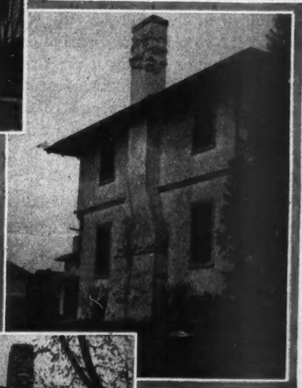
Protruding Rock, Placed at Random Near the Base and the Top of the Stucco Chimney Adds to Its Attractiveness.
