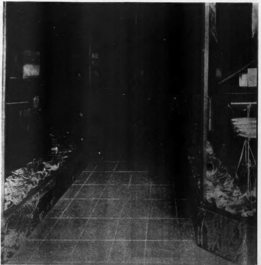
Flooring Material in Which an Abrasive Is Incorporated Finds an Increasing Use for Store Fronts, Public Places and All Purposes Where a Firm Footing and High Resistance to Wear Is Important.
