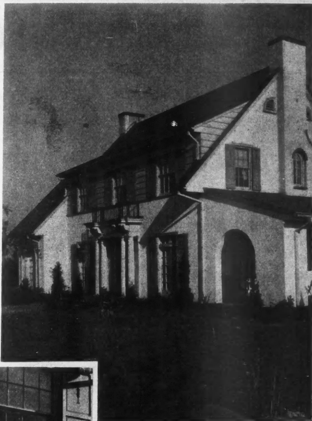
Balance Without Monotony Is Achieved Through the Projecting Sun Porch at One End of the J. P. Brady Home and the Open Porch on the Other.
