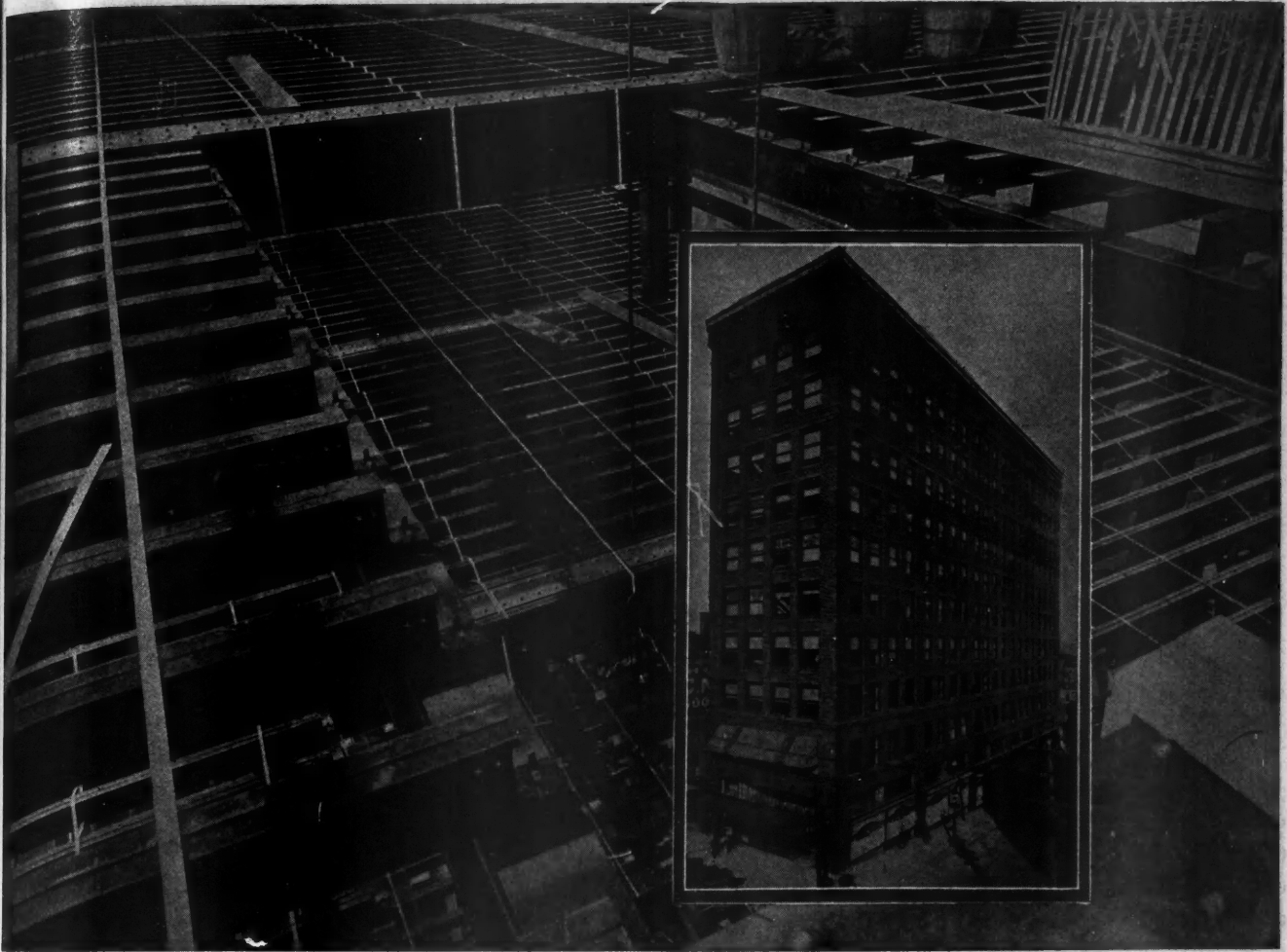
Berloy Metal Lumber in eleven floors and roof of Renkert Building, Canton, O. Architects Walker and Weeks, Cleveland, O. Contractors, Conley Construction Co.
