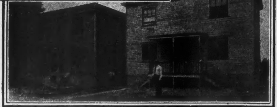
These two attractive, four-apartment, brick buildings vividly show what a little remodeling and Face Brick veneer accomplished for the two old frame buildings shown at the right, in a row, seen above, on Rhode Island Street, Gary, Indiana. Contractor and Builder, Marcello Gerometto.
