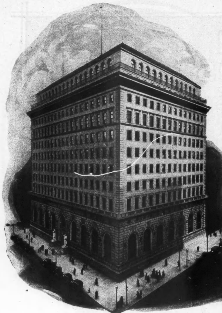
FEDERAL RESERVE BANK OF CLEVELAND Atlas White Portland Cement mortar used for setting, backing and pointing the stone.
