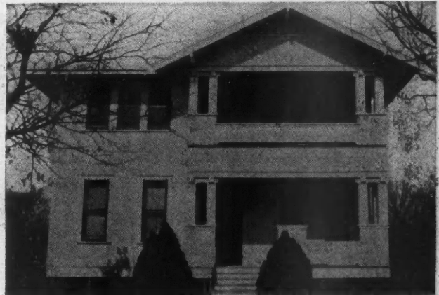
Another Home Erected by Robert Felsing, of Seguin, Texas, Sent to the Correspondence Department as Typical of Texas Residence Construction.
