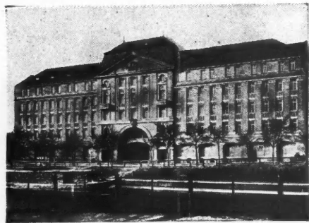
Sales Department of a Furniture Factory: In which Terranova has been used throughout; first as a beautiful wall surface that is as perfect as natural stone and again in the decorations which were cast in the same material to harmonize with the architecture of the building.
