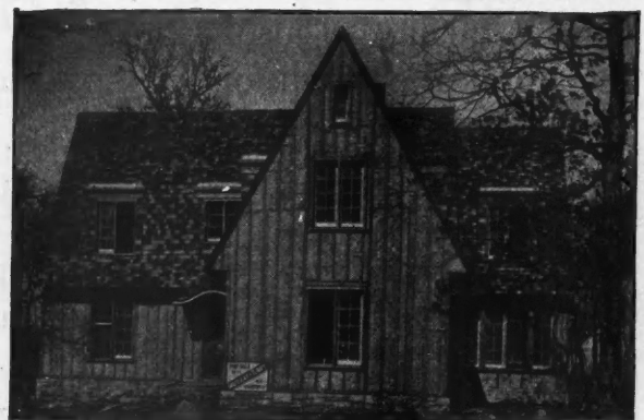
House near Chicago, showing its "underclothing" of Cabot's Quilt, with furring strips over the Quilt, on which the outside finish is laid. Roof also insulated. Leon E. Stanhope, Architect, Chicago
