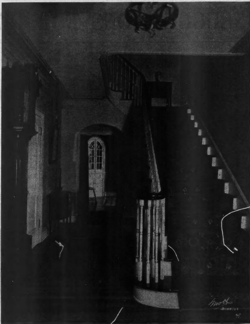
Stairways and Halls Such as the One Illustrated Here Are Charming Features of Many Modern American Homes. They originated with the builders of the American Colonies, who adapted the Georgian styles of England to the new environment.
