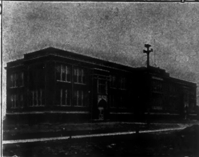
CATHERINE B. WHITE SCHOOL, Detroit, Mich. Architects, Malcomson, Higginbottom & Palmer Contractor, John Hollis Co.
