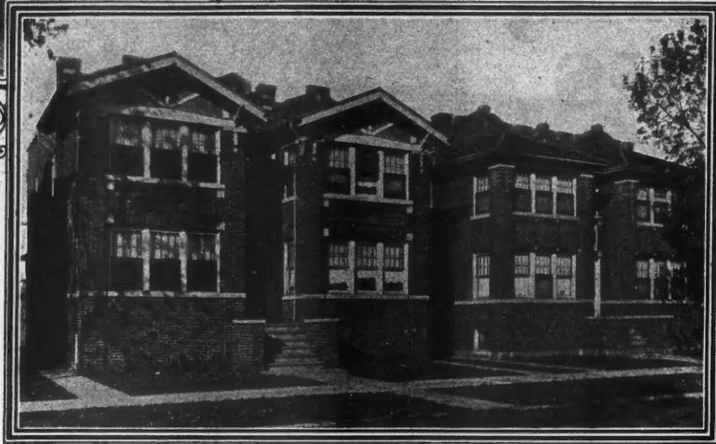
These two attractive, four-apartment, brick buildings vividly show what a little remodeling and Face Brick veneer accomplished for the two old frame buildings shown at the right, in a row, seen above, on Rhode Island Street, Gary, Indiana. Contractor and Builder, Marcello Gerometto.
