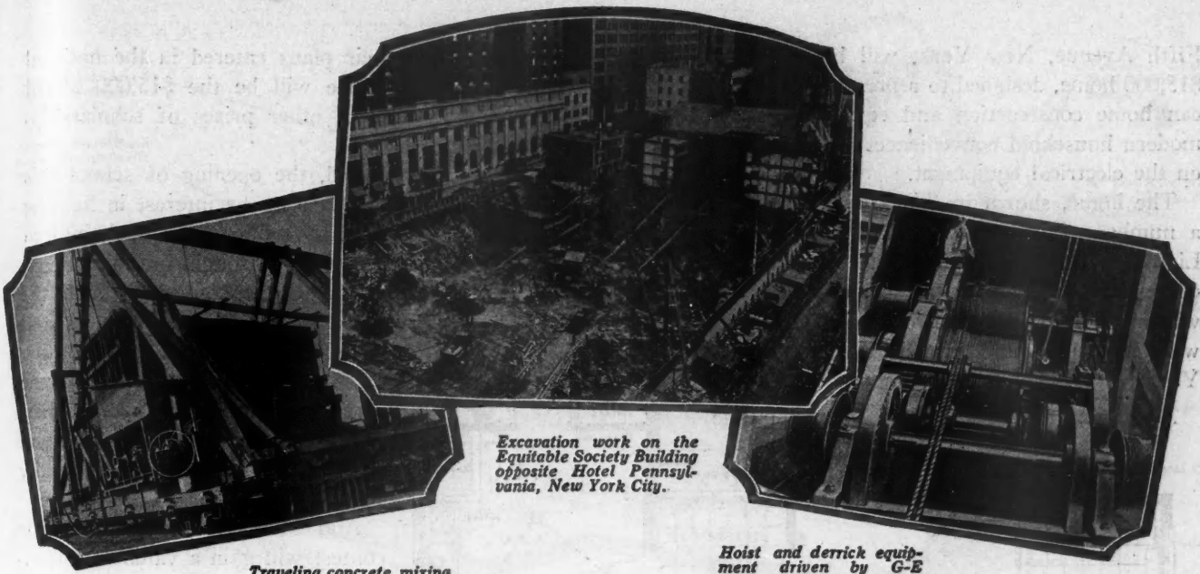
Traveling concrete mixing plant on foundation work at Valhalla, N. Y. Operated by G-E Motor.
