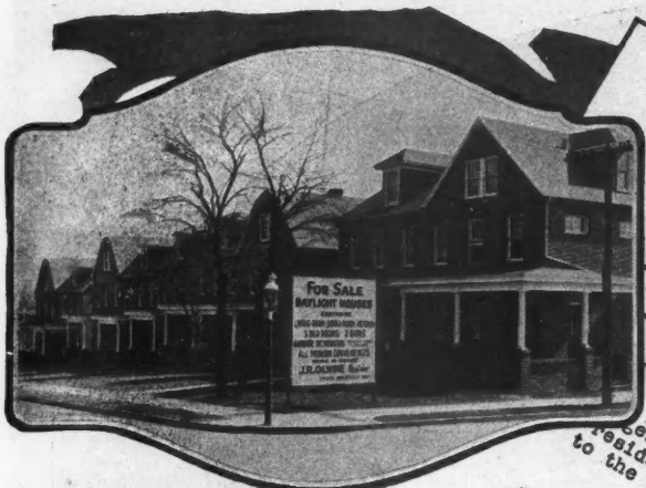
Nine Kernerator-equipped residences, constructed for Mr. W. E. Byrd, by I. R. Olivine, at Alto Avenue and Division Street, Baltimore, Maryland.
