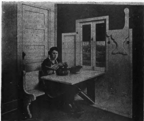
Part of the Built-In Convenience Dropped Down to Make a Work Table for the Kitchen Tasks.
