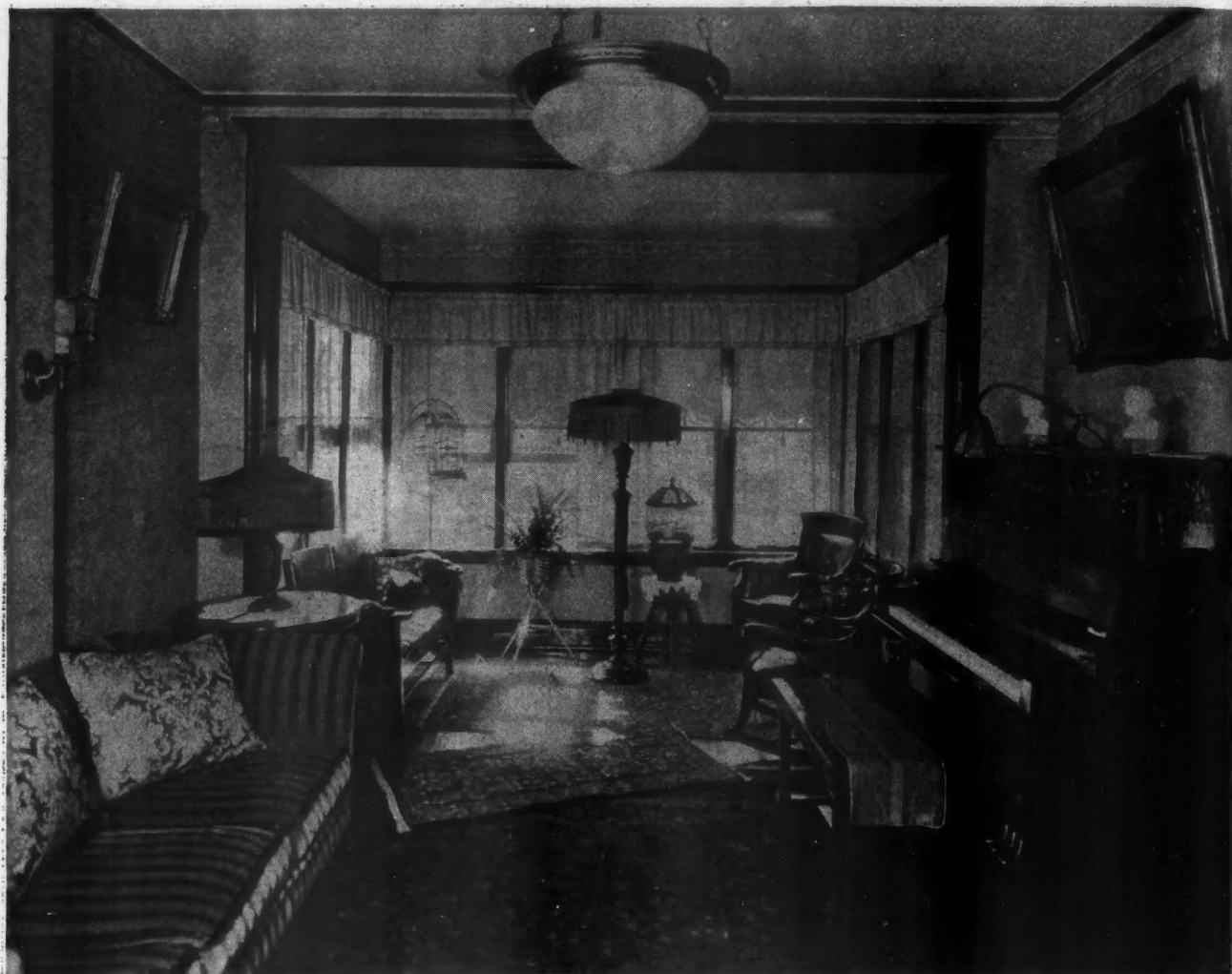
The Sun Parlor, with Narrow Mullioned Windows, Not Only Gave Much Additional Space Within the House, but Greatly Increased the Amount of Light Admitted to the Rooms Behind the Sun Room. The illustration shows the pleasing and modern room made available through remodeling the front of the home.
