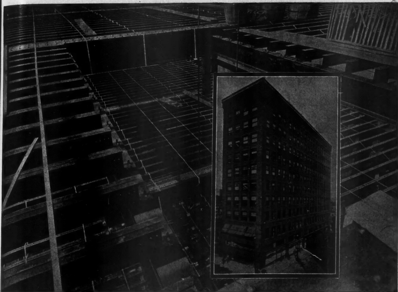
Berloy Metal Lumber in eleven floors and roof of Renkert Building, Canton, O. Architects Walker and Weeks, Cleveland, O. Contractors, Conley Construction Co.
