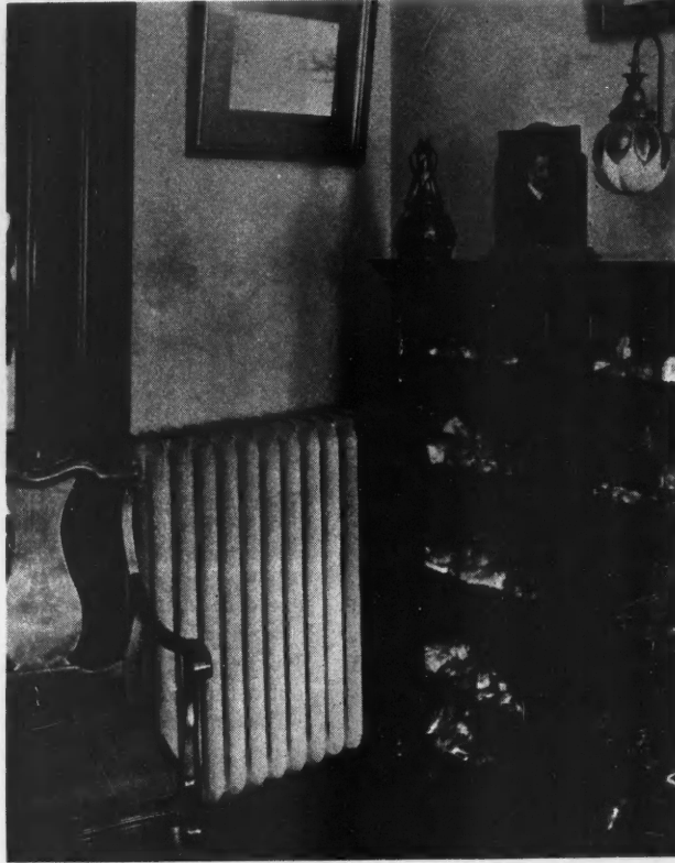
The Painting of This Radiator Made a Pleasing Variation from the Usual Bronze—Gold by the Use of the Same Color Used on the Walls. Aluminum paint, although toning in with the color scheme, was rejected because of its heat retaining property.
