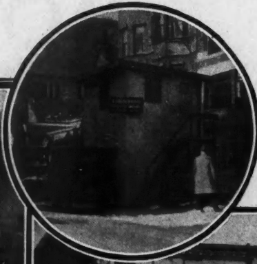
Contractors field office in Boston covered in the fall—there all winter. Note, no battens were used to hold the paper, just nails.
