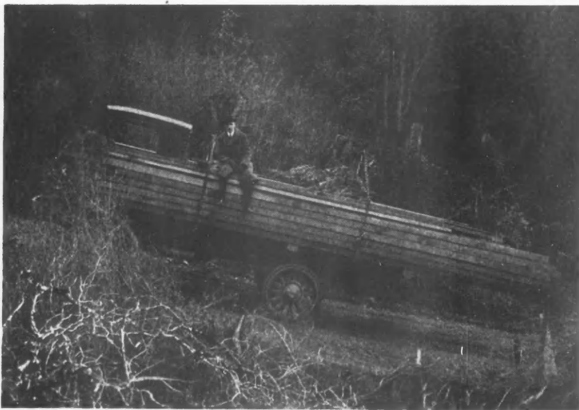
The 5-ton Autocar was stopped on this 15 per cent grade to take the picture, but pulled right away with its load of green redwood after the picture was taken
