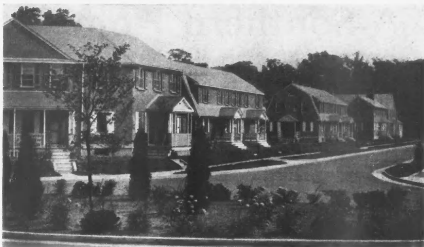
One of the Streets in the Westinghouse South Philadelphia Housing Project for Employees of the Company. It is now planned to extend this project over a tract of land large enough to accommodate 500 to 600 dwellings.
