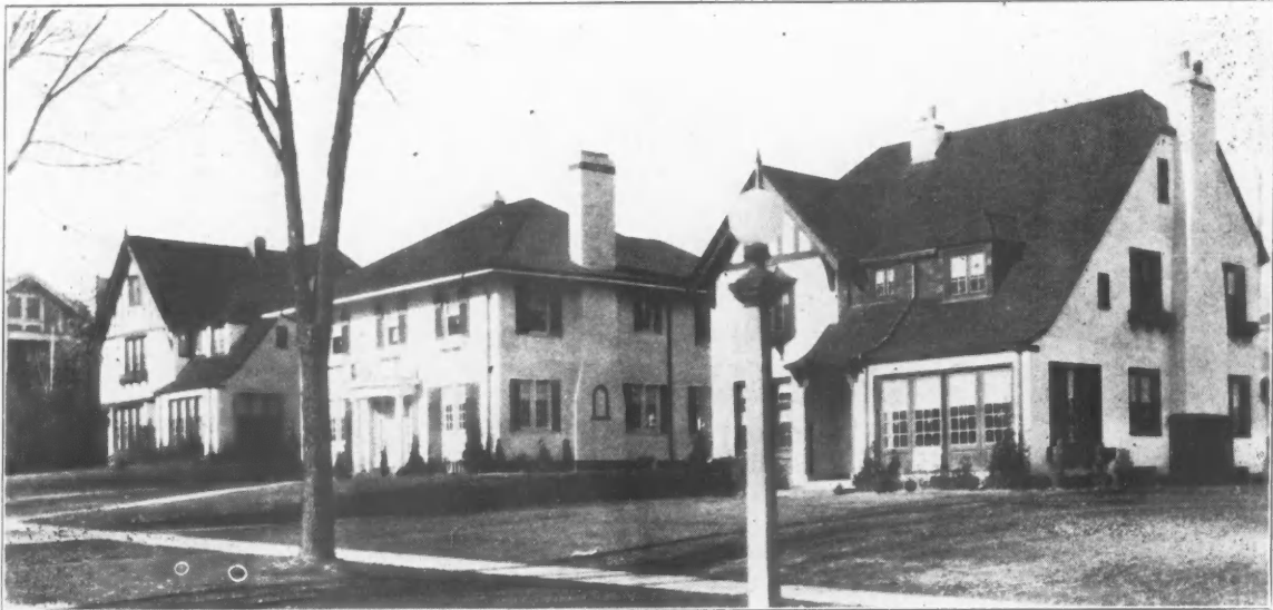
Bishopric Row—Bishopric Stucco over Bishopric Base in this row of Rochester, N. Y., houses.
