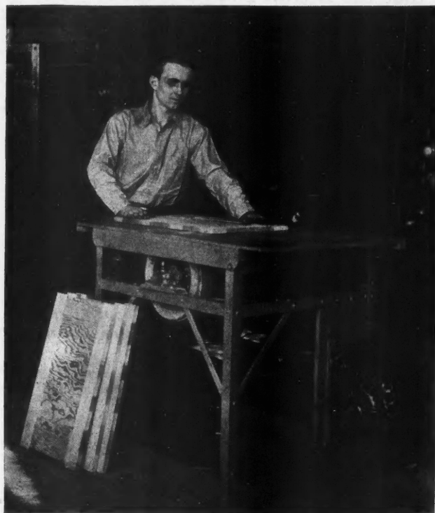
This Portable Power Operated Drum Sander Will Do the Work of Six or Eight Men with Hand Scrapers and Planes.
