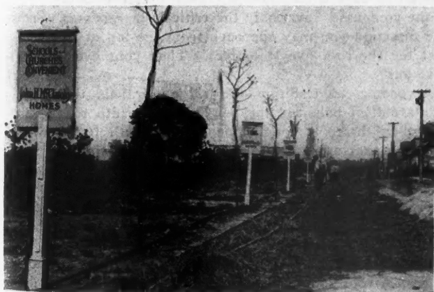
Here Is a Row of the Smaller Signs Used Along Long Lane, Which Was in Course of Construction at the Time This Picture Was Taken.
