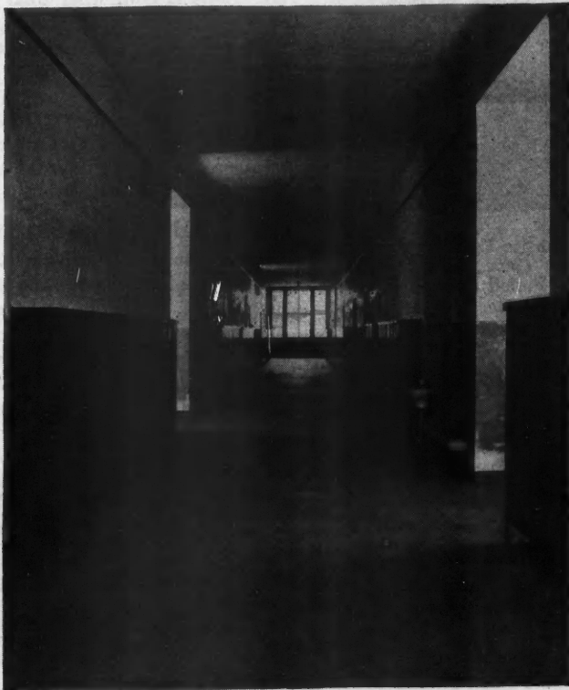
One of the Most Severe Tests to Which a Flooring Material Can Be Put Is in the Halls of a School Building Where Hundreds of Children Tramp Back and Forth Over Its Surface Every Day.
