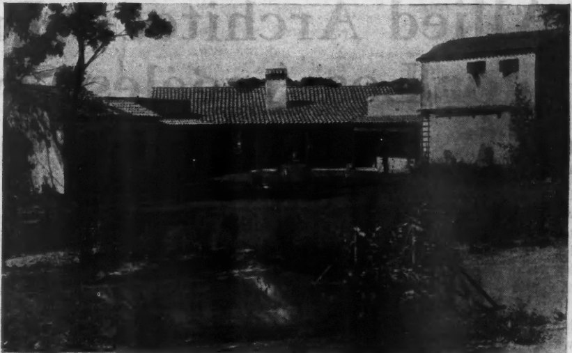
As Seen from the Patio Side the House Is Even More Individual and Inviting than from the Street. Here one might feel far removed from any suggestion of the bustling city.
