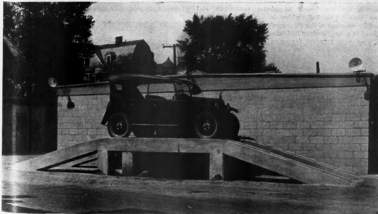
A Concrete Oiling Trestle Is Neat and Permanent. It will safely carry any weight up to 16,000 pounds, the grades are easy and protected from slipping. It is more easily kept clean than the ordinary type of trestle.
