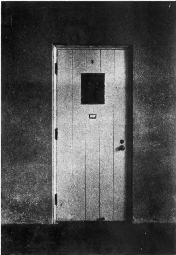
Artistic Simplicity Is the Note in the Doors of the Class Rooms Which Open Onto the Cloisters.
