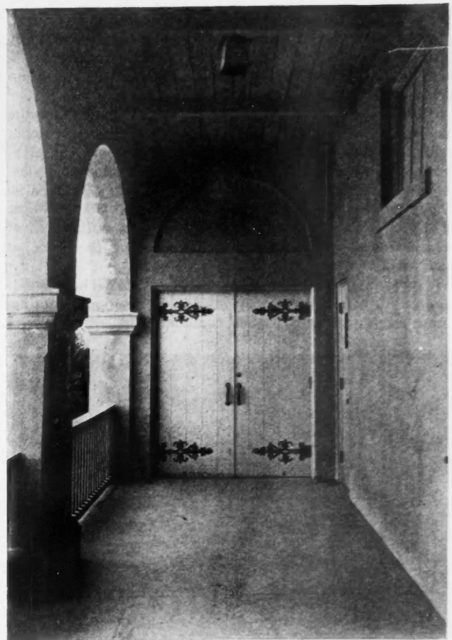
Where the Cloisters Join the Inner Corridor of the Central Portion of the Building, Rigidly Plain Doors Are Perfect Foils for Exquisite Wrought Iron Hinges.
