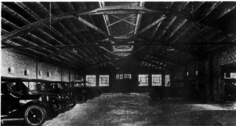
Here Is an Example of the Combination Wood and Steel Truss as Used in a Public Garage in Chicago. The span is 50 feet.
