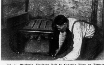
Fig. 2. Workman Fastening Bolt to Concrete Floor on Furnace Installation. The cold air duct, at the left, is ready to receive the boot connection to join at the bottom of heater casing.
