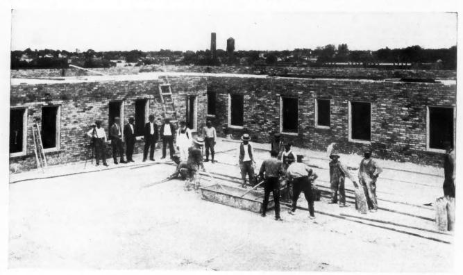
Concrete Roof Deck of the La Salle Hotel Annex, South Bend, Ind., Being Insulated with Two Inches of Cellular Gypsum. The material is mixed in the metal mortar-box, then dumped into a section formed by a two by two-inch strip on one side and a section of the poured and set gypsum on the other side. When it sets and dries out it is ready to be covered with composition roofing.
