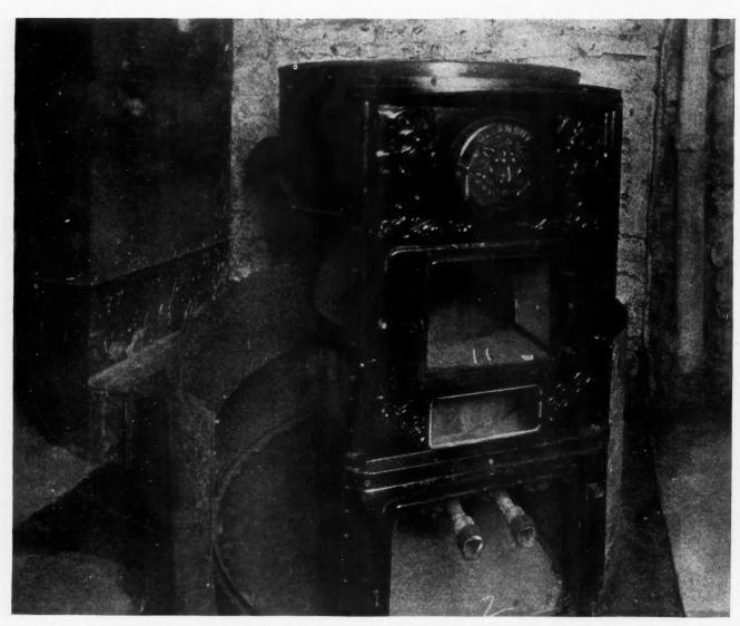
Fig. 1. Connecting the Cold Air Boot to the Bottom of the Furnace Casing. Located at the rear, a portion of air passes to the near side of the casing and the remainder to the rear and far side, assuring equal heating of the entire supply.
