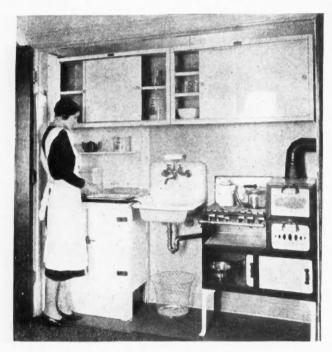
The Latest Feature of These Kitchen Wall Cabinets Is the Sliding Doors Which Are Never in the Way, and Eliminate Bumped Heads.
