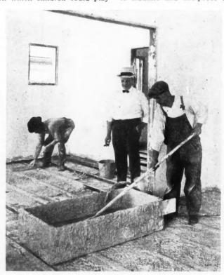
Insulating Floors in the Boswell Apartment Building with Cellular Gypsum. The material is mixed in a mortar-box and poured between the sleepers. A workman is shown leveling it to within an eighth of an inch of the upper surface of the sleepers.
