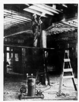
This Paint Spray Brush Can Be Obtained in Two Sizes and Either Compressed Air or Gravity Feed Types.
