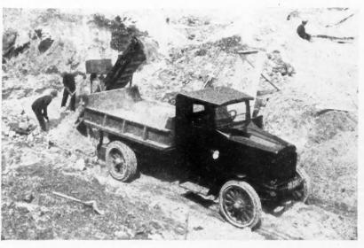
This Job Presents a Severe Test for Any Truck. Heavy loads and poor traction at the loading point put a strain on engine, running gear and tires.
