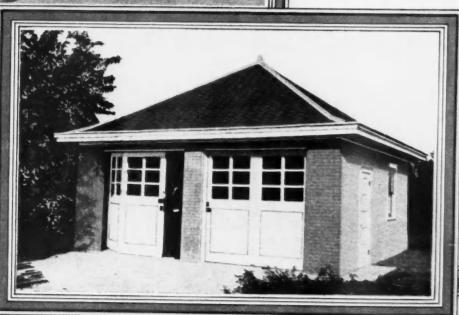
THE OSAGE GARAGE, a double garage of brick construction. Doors arranged to slide inside back around the corners.
