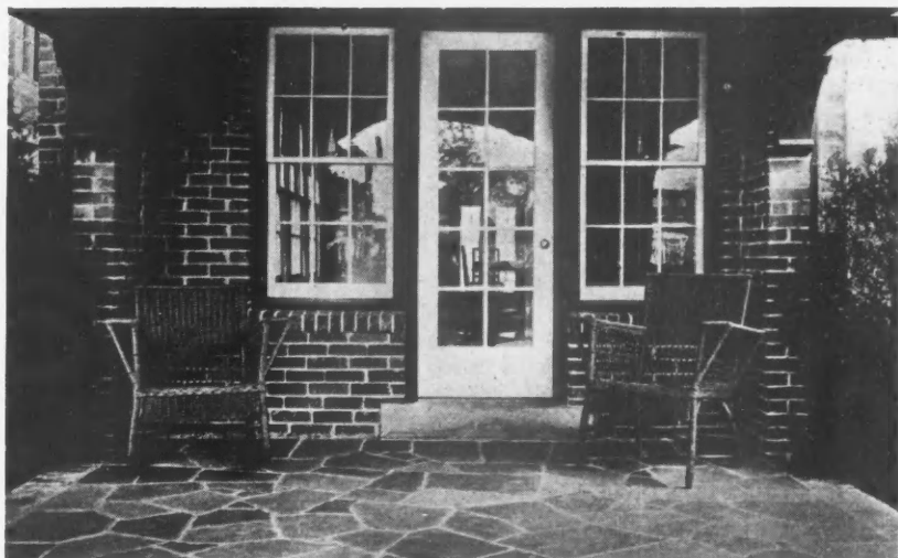
Here the Irregular Pieces of Flagging Have Been Jointed with Cement, a Slightly More Formal Treatment but Affording a Smoother and More Practical Surface for Porch Flooring.
