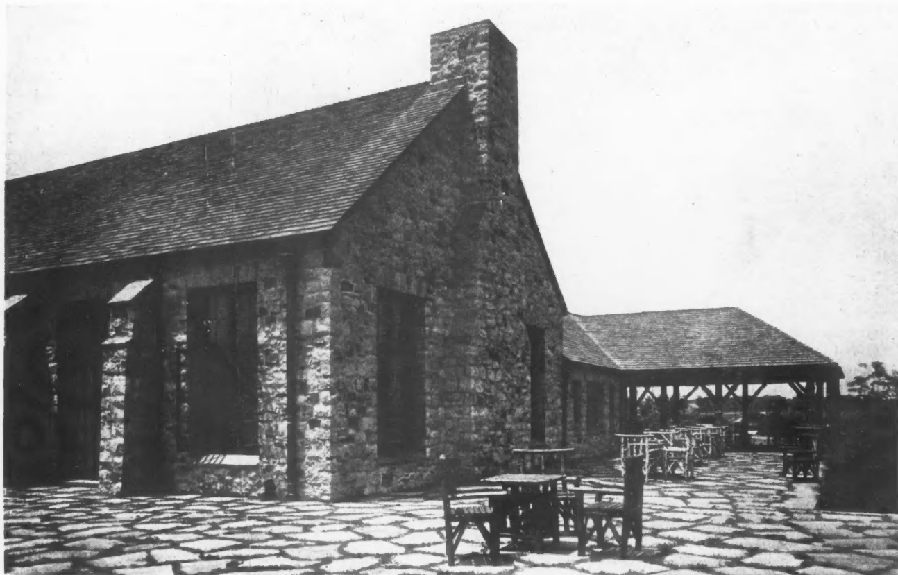
At the Norwood Club One May See This Terrace of Slate Flagging, the Irregular Pieces, Interspersed with Grass, Achieving an Effect Which Sets Off to Perfection the Rough Stone Walls of the Club House and Creates a Charming Atmosphere Which Would Be Difficult to Rival with Any Other Material.
