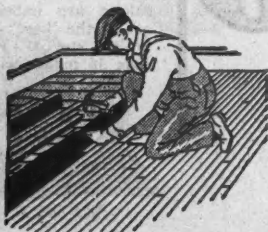
Laying an Oak Floor
