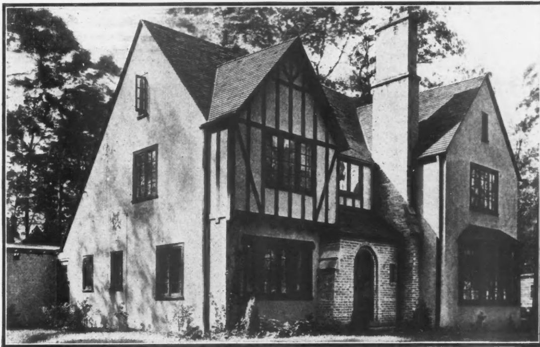
Home of C. S. Cawthorne, Lake Bluff, Illinois. T. W. Jackson, Builder. White & Weber, Architects. Celotex Insulating Lumber used for sheathing and insulation in place of wood lumber and any extra insulating material.
