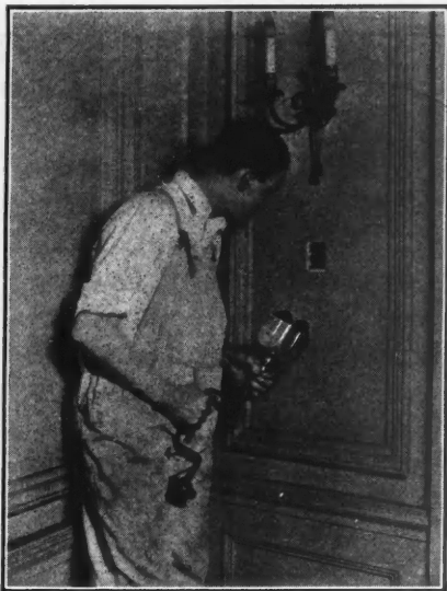
This Simple Tool Cuts an Outlet Hole for Pipes or Electrical Wiring in from One to Three Minutes.
