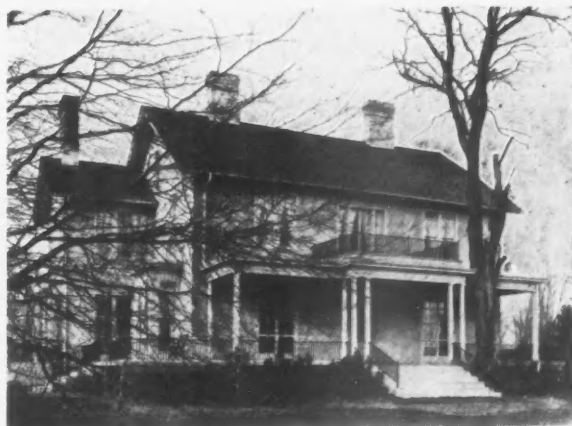
After an Overcoating Treatment the Old House Could Not Be Told from a New Stucco Home.
