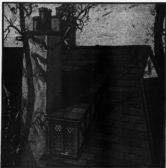
These New Asbestos Shingles Are Laid Horizontally Giving an Attractive Effect and Deep Shadows.
