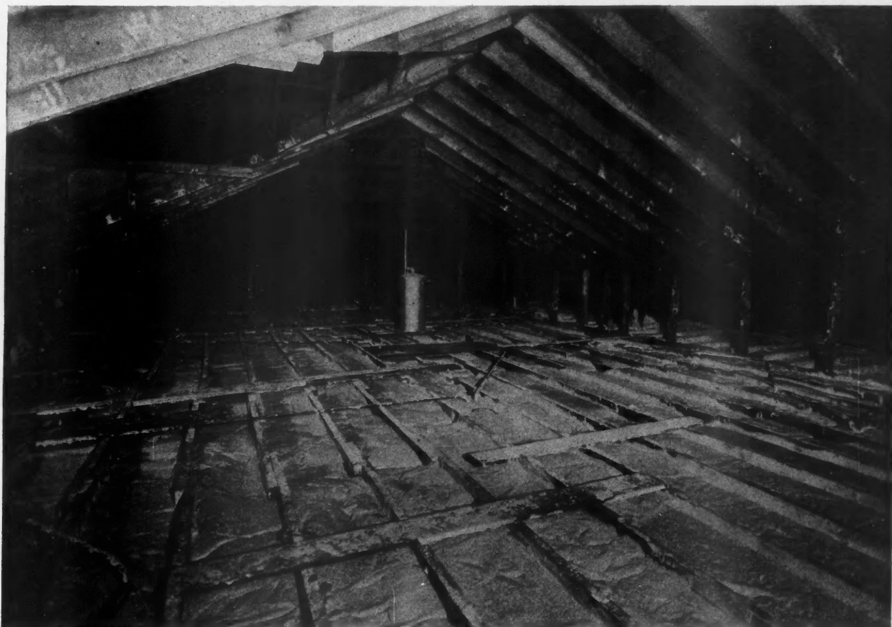
The Insulation Used in This Attic Effected Quite a Saving in the Gas Bills for the Two-Story Brick House Pictured Above. The type of insulation used is mixed with water and poured in place over the top ceiling. It adds fire resistance to the building.
