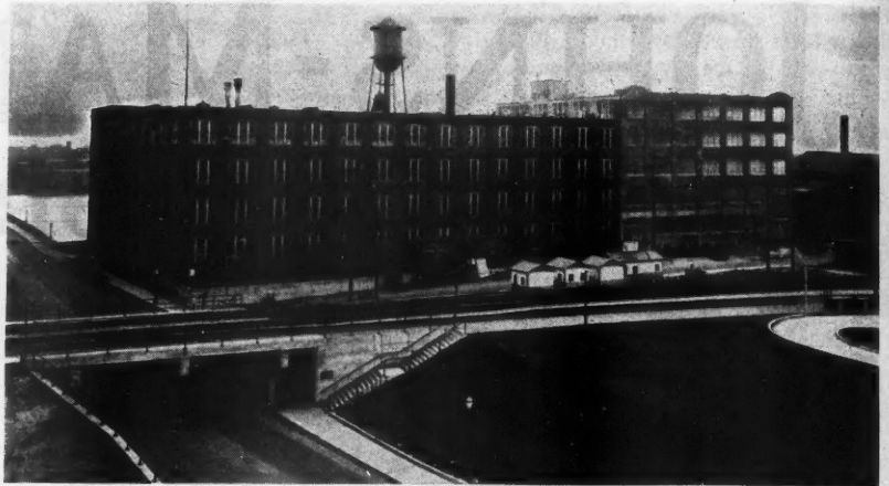
The Plant of the National Mfg. Co. at Sterling, Illinois. In the new wing at the right 6,000 of the concrete inserts described here were used.
