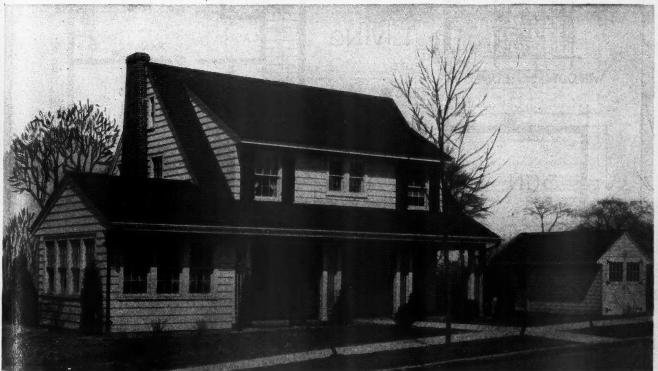
A Charming Suburban Home, Complete Even to the Garage Which Harmonizes with the House Design, Has Been Selected for Our Front Cover Home. It is shown in full colors on page one while on the next four pages floor plans, elevations and details will be found. Oscar G. Nordstrom, Ridgefield Park, N. J., Architect.
