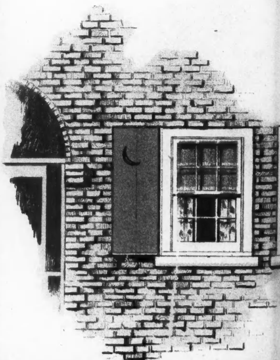
Detail of Skintled or Irregular Laid Brick Work Near Entrance.
