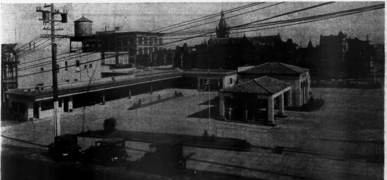
A Bird's-Eye View of the Calpet Service Station Shows the Ample Room Available for All Kinds of Service, Washing, Battery Service, Tire Changing, Gas and Oil, with Wide Approaches to Each.
