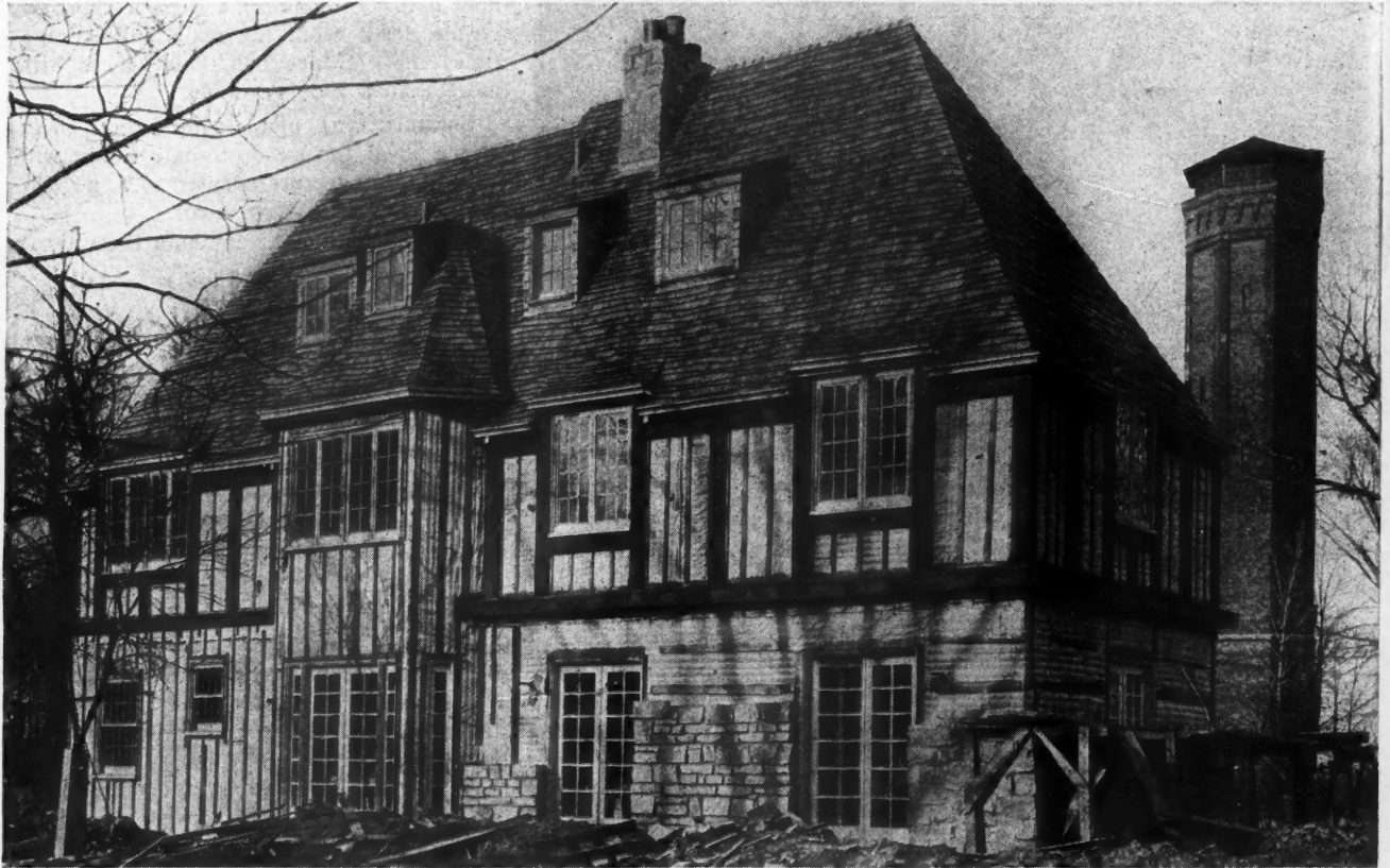
One of Chicago's Fine North Shore Homes as It Appeared During Construction. The stone veneer is just being applied and the complete wall insulation is still to be seen as applied over the sheathing. The same insulation has been used in the roof as well.
