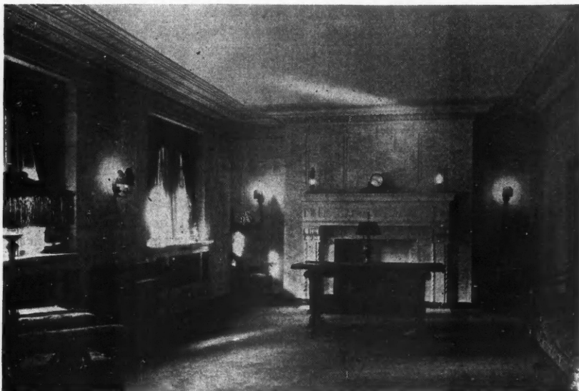
Fig. 2. A More Elaborate Plaster Cornice, a Combination of Run-In and Pre-Cast, in the Lounge of the James Apartments, Designed and Built by T. H. McHale & Son, Syracuse, N. Y.
