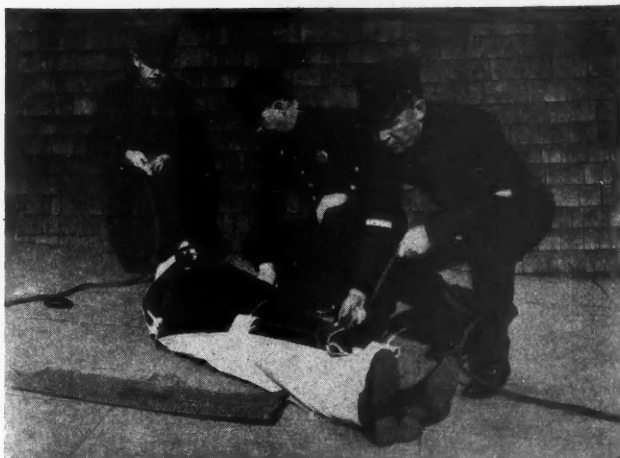
Here Is the Method of Fastening an Accident Victim into the Stretcher for Lowering from a Building. This can be done by a single rescuer where required.
