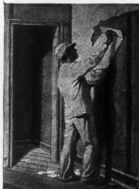
UNDER PLASTER. On inside walls and ceilings Celotex replaces lath—forming insulated walls that are stronger, less apt to crack and forever free from ugly lath marks.
