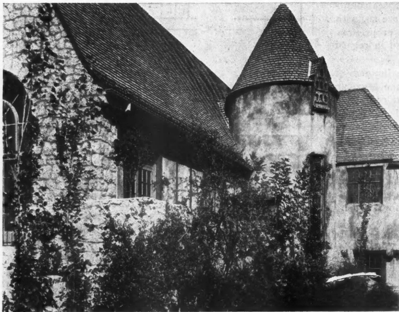
A Close-up Reveals the Charm of Texture in Building Materials and How Cleverly the Substantial Masonry of the Normans Has Been Simulated in Stucco and Rock. The mullioned windows also emphasize the period effect.
