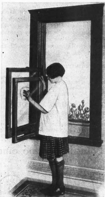
Here Is a System of Window Installation Which Permits the Window to Either Slide or Swing.
