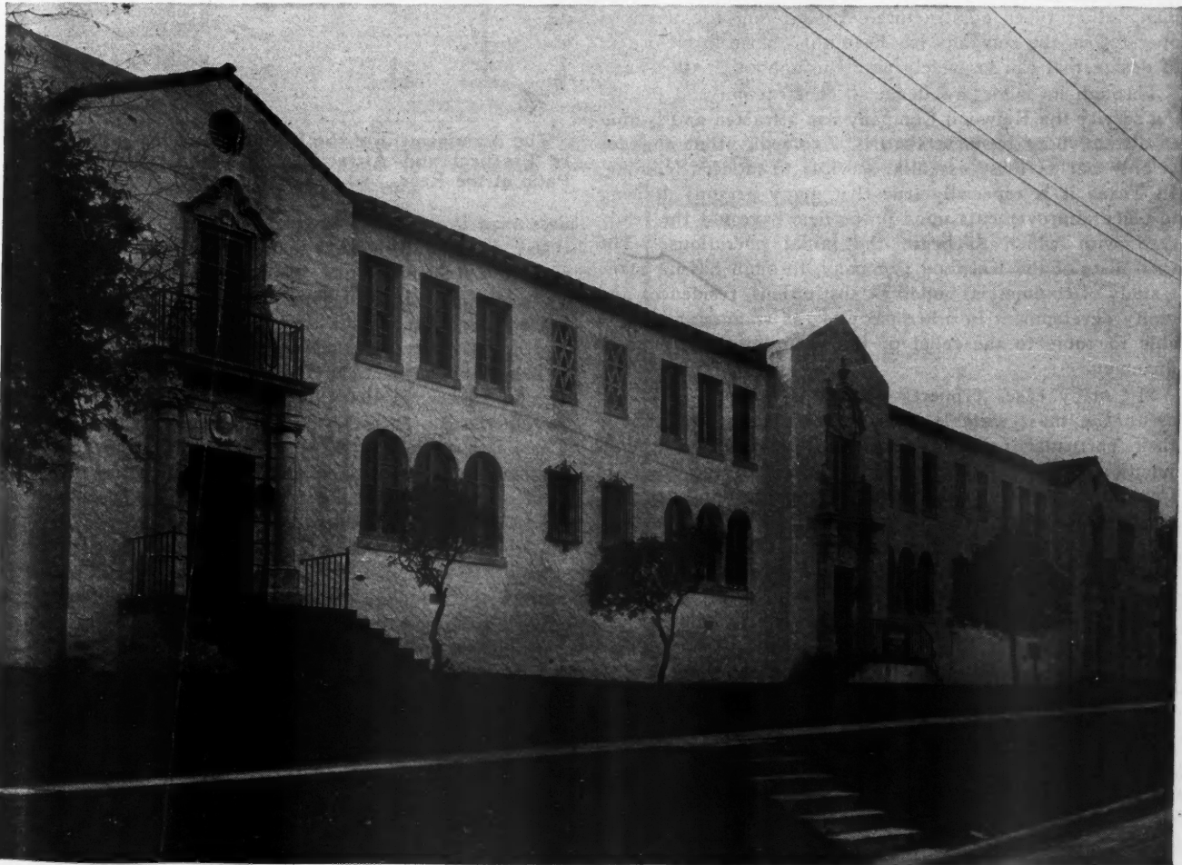
The Operations of the Kelwood Company Are Not Confined to Single Houses. The San Gabriel Apartments, in San Antonio, contain twelve four-room apartments, and a ten-car garage, all handled in the Spanish style, at a cost of $75,000.
