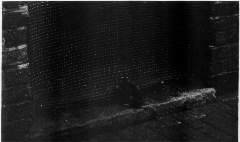
Screened Basement Windows Are a Necessary Part of Rat-Proofing Any Building. Every means of entrance must be closed.
