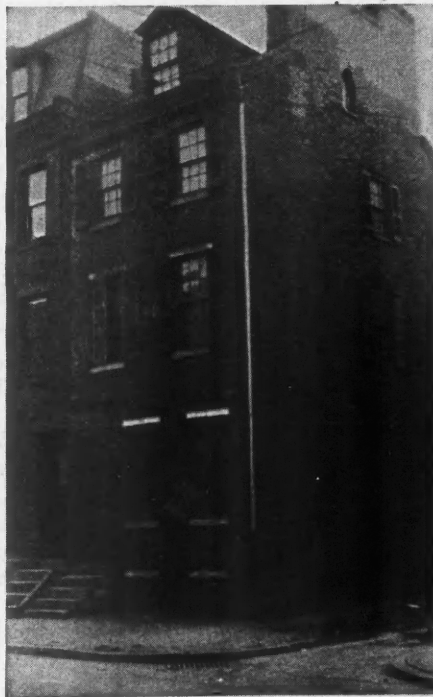
The Two Old Houses Shown Above as They Appeared Before the Improvement Work Was Undertaken.
