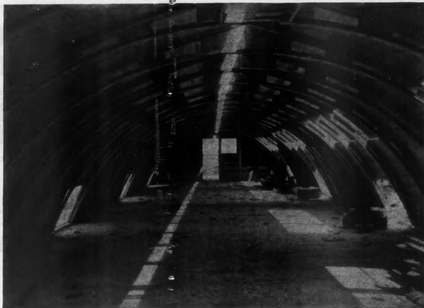
Close-Up View of Roof Trusses.
