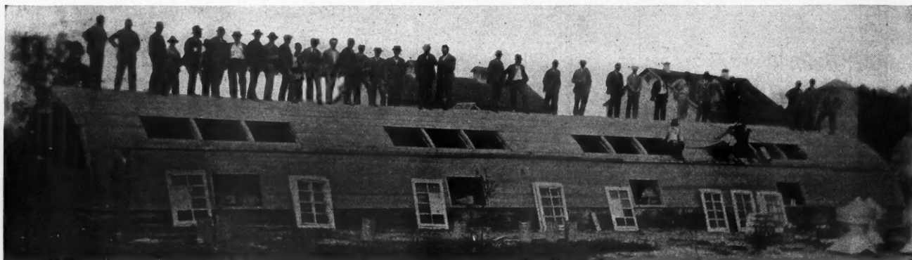
The Poultry House on the Jefferson County (Wis.) Farm, Designed by the James Mfg. Co. More than two tons of weight on the roof trusses are represented by the men standing.
