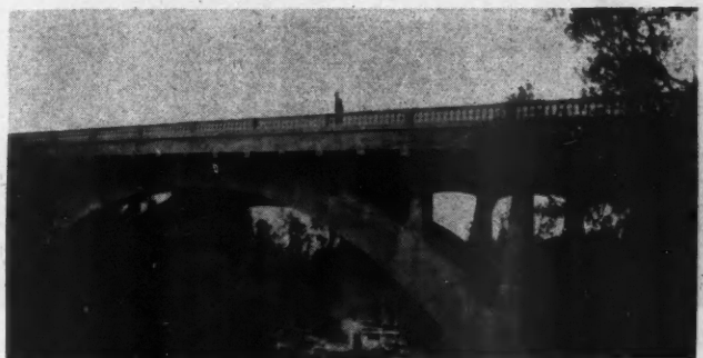
The "Arroyo Seco" Bridge, a Single Concrete Arch.
