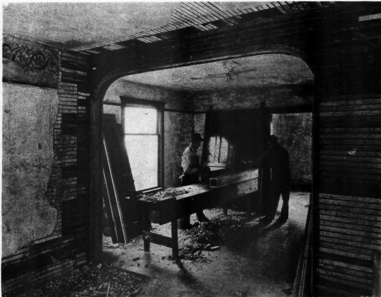
Making a Living Room of the Old "Front Parlor" and "Back Parlor" by Substituting an Arched Opening for the Old Sliding Doors Was One Step in the Rehabilitation of This Old House in Dixon, Illinois.
