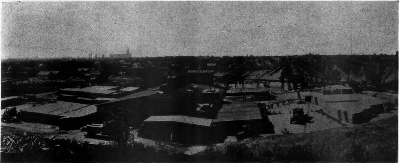
A Self-Contained Concrete Products Factory. A gravel pit, at the right, supplies much of the raw material needed, which is carried directly into the production system, where it is cleaned and scientifically mixed with portland cement to produce high-strength masonry units, stocks of which are seen in the left and right foreground.
