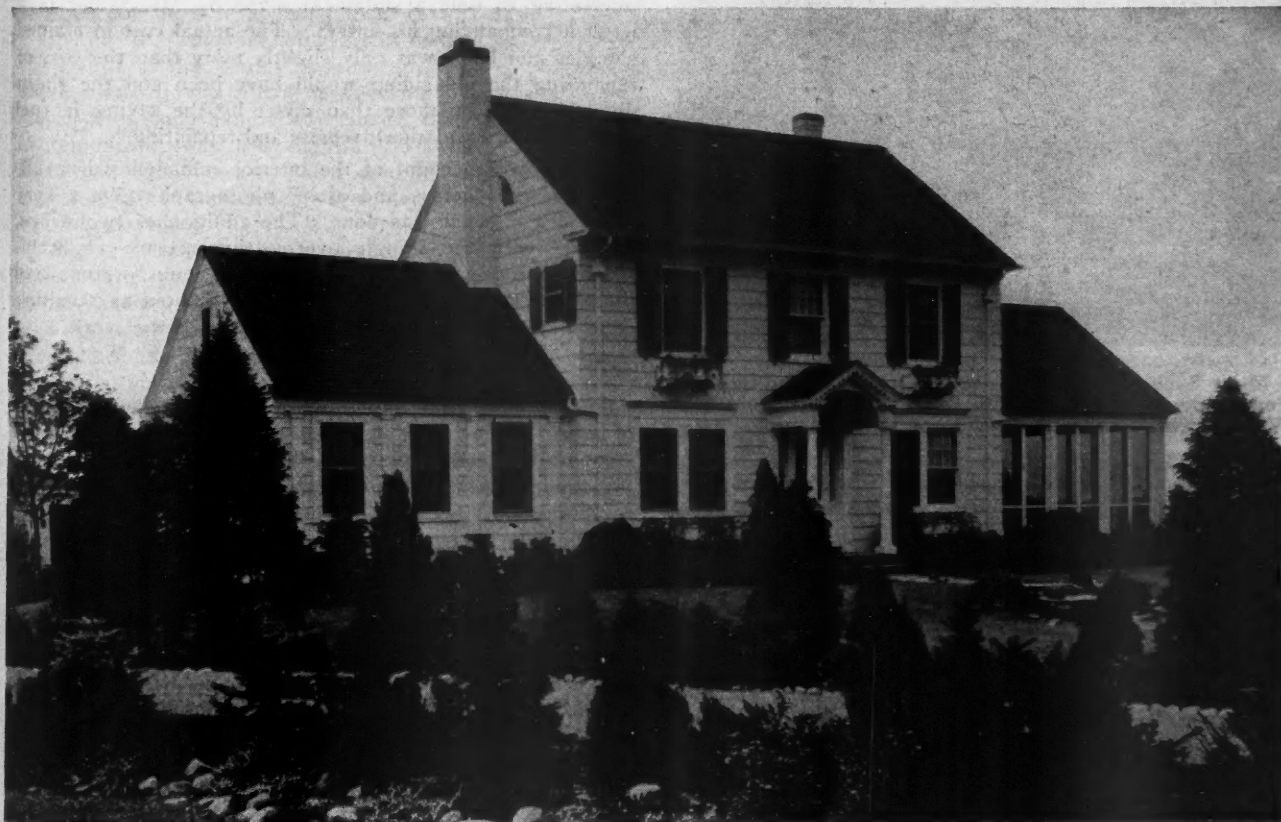
From a Crude, Inhospitable Structure, as Seen in the Small Illustration Above, This Architecturally Beautiful Country Home Was Created by the Addition of Two Wings and the Application of Wide Colonial White Shingles Over the Original Narrow Siding.
