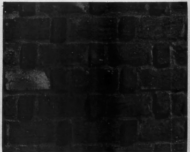
Mixed Clinkers and Swelled Brick, Laid All-Rolok, Headers Projecting. Mrs. M. G. Thompson, owner; Van Belt, Thompson & Churchill, architects, New York.
