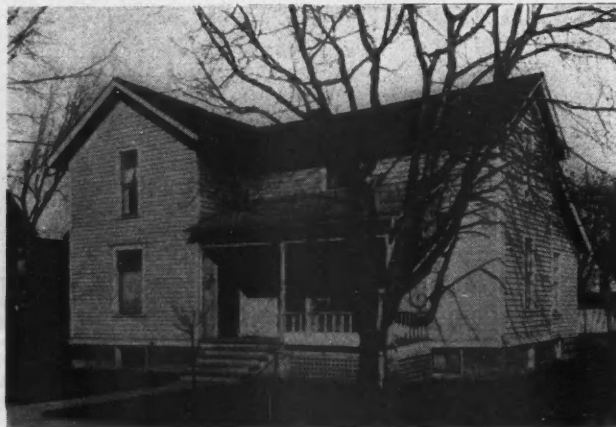
Many Such "L" Type Houses Are to Be Found in Every Community and Afford a Profitable Field for the Contractor Who Appreciates the Possibilities of Remodeling.
