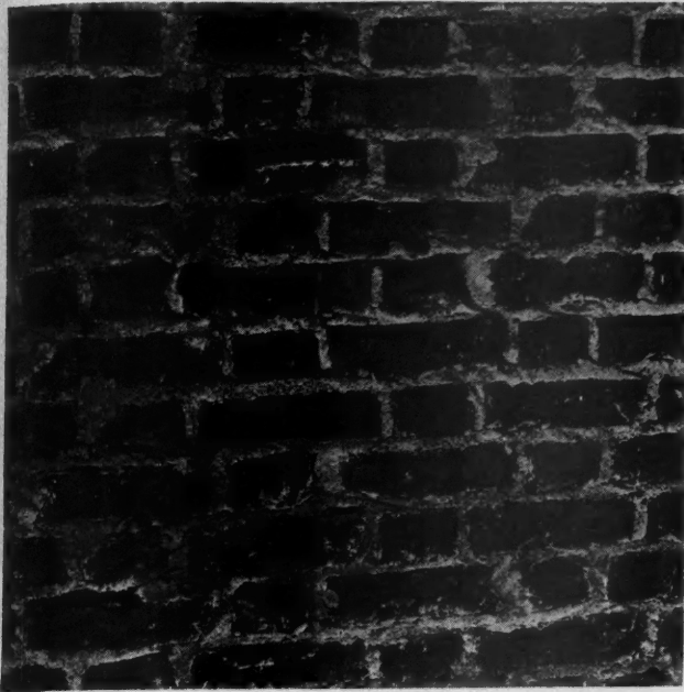
An Over-Burned Brick Laid in Flemish Bond and a Natural Mortar. J. M. Haynes, owner; Parks & Baxter, architects, Washington, D. C.
