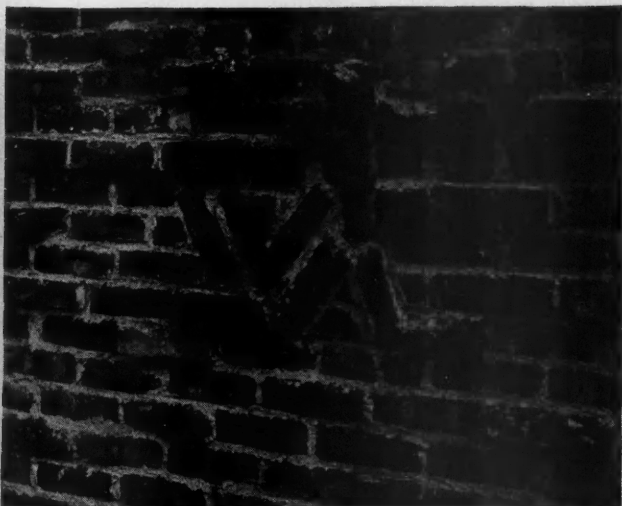
Dark Reds and Browns, Semi-Skintled, with Unusual Fireflashings. Dr. J. A. Fordyce, owner; R. G. Dixon, architect, Pittsburgh.
