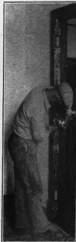
Hinge Butt Router and Templet on Jamb
