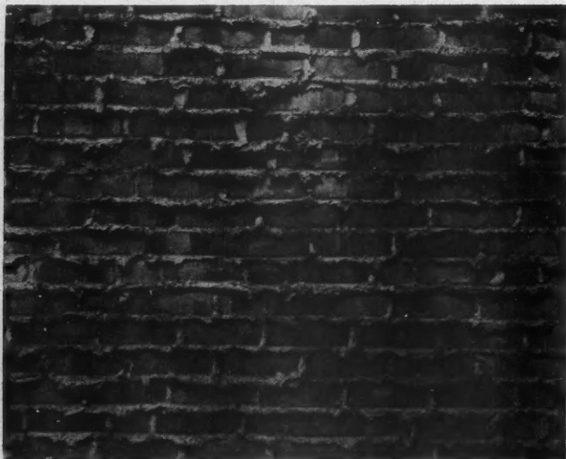
Another Type of Skintling, Pressed Joint with Mortar Overhang. J. E. Plant, owner; Bohnard & Parsson, architects, Cleveland.
