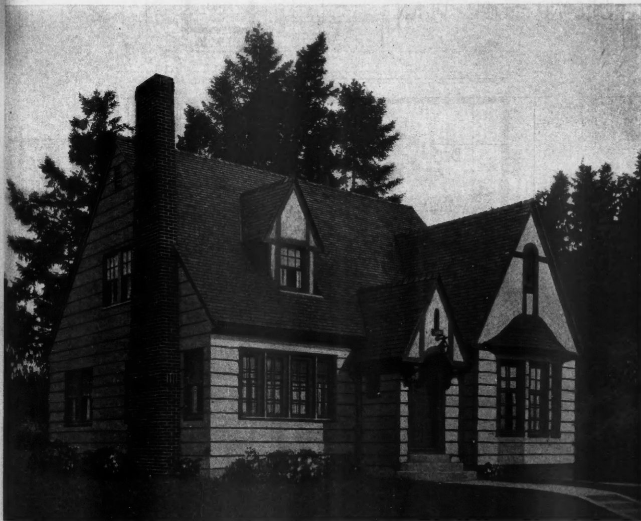
An English Cottage Type of Home Incorporating Every Modern Convenience. The compact arrangement of rooms may be seen by referring to the plans, drawn to scale, which are shown on the pages following this.
