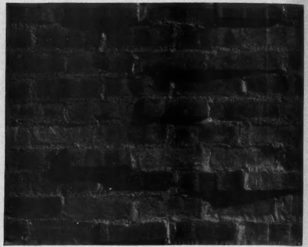
Projected Stretchers Which Furnish an Interesting Play of Shadow. T. S. Etheridge, Jr., owner; Louise M. Gilleo, architect.
