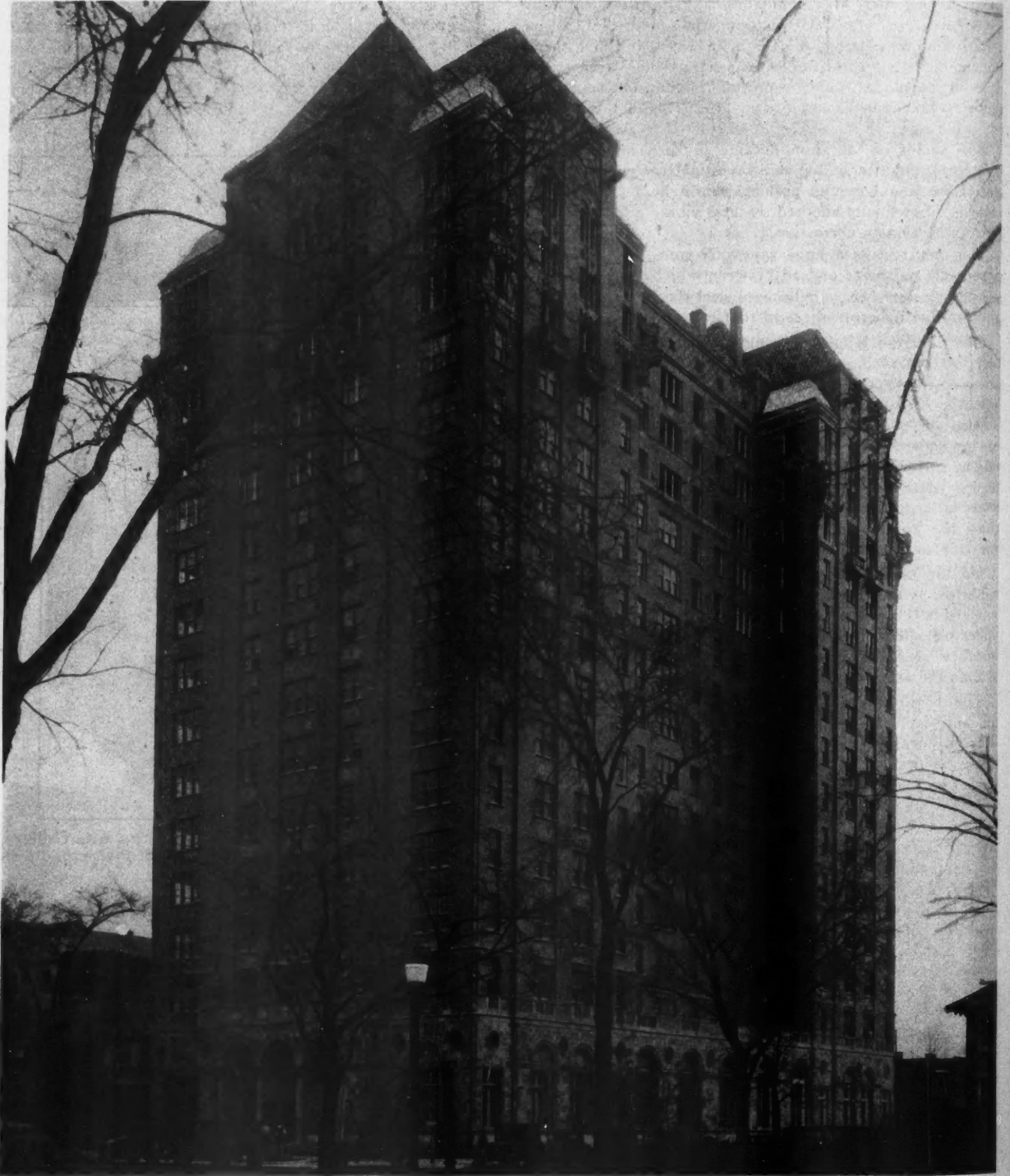
The Lee Plaza Apartment Hotel, Detroit, Owned and Built by an American Builder Subscriber, Mr. Ralph T. Lee, Is Said To Be Detroit's Finest Building of This Type. Among other innovations, it has an airplane beacon on the roof which throws a nine million candle power light into the sky and has been recognized by the government as Detroit's official airline beacon.
