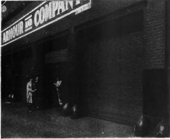
Strong Steel Doors that Roll Up Out of the Way Overhead and Are Furnished in All Sizes.
