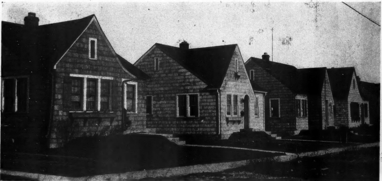
These English Shingle Type of Houses Have Met with Great Favor Among the Modern Housing Corporation's Customers in Flint. They may be bought with a down payment of $300 and upward.
