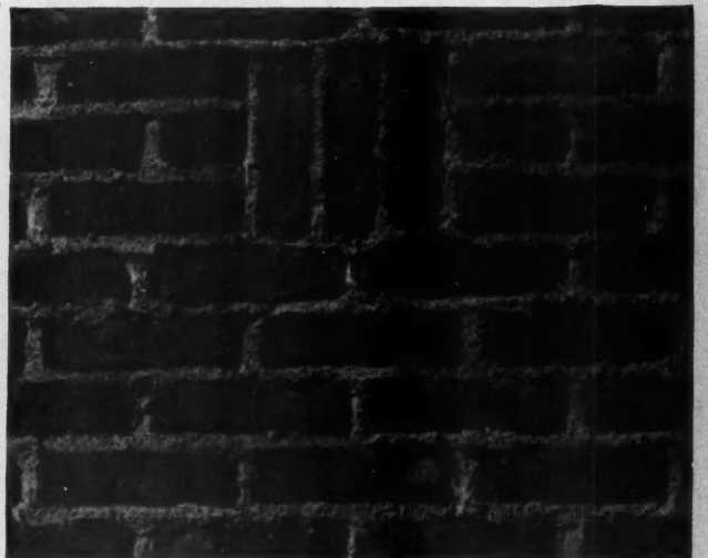
A Variety of Reds in a Pressed Joint with Natural Mortar. J. J. Cromwell, architect and owner, Woodmere, L. I.
