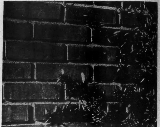
Note the Play of Shadows in This Deeply Raked Joint. Darrah Corbet, owner; A. L. Loveless, architect, Seattle.
