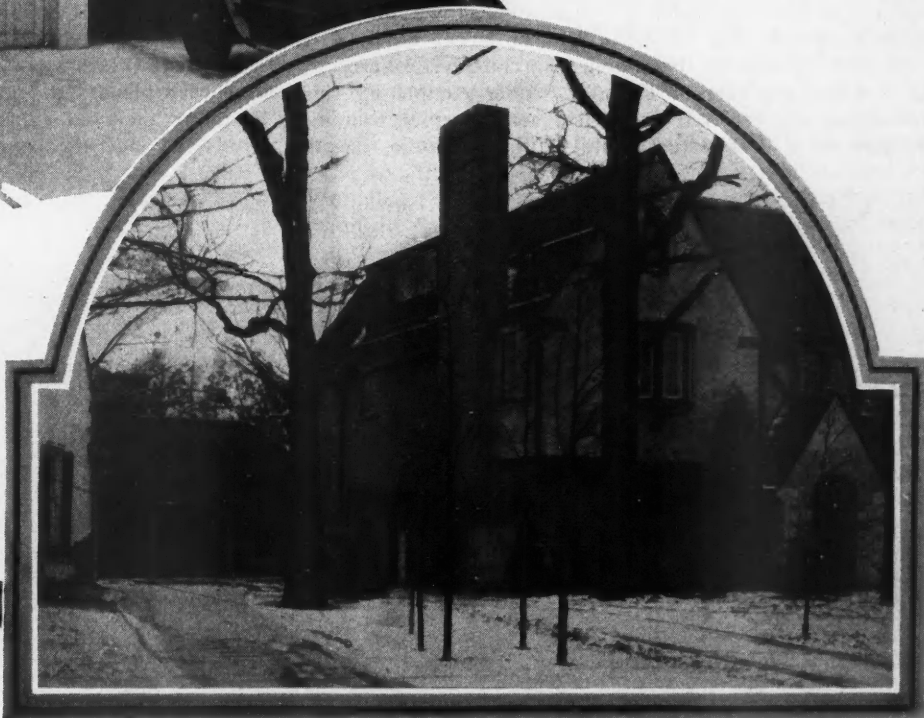
Home with Garage in Harmony in Palmer Woods, Detroit; Frazier Couzens Building Co., Builders.
