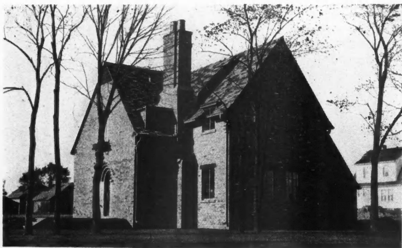
One of the Higher Priced Homes of the Modern Housing Corporation Development Located on Nolen Drive. On this street, restricted to the more expensive type of homes, the company plans to concentrate a large share of its building program in 1928.
