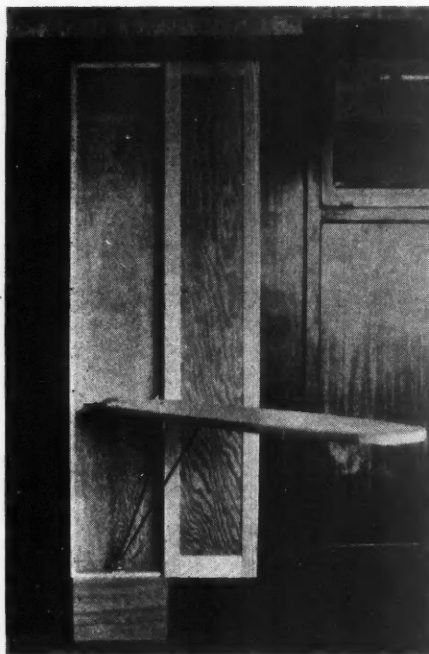
A Built-In Ironing Board Which Takes Very Little Space Because of Being Pivoted.
