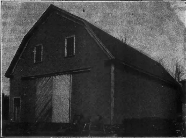
Asphalt Shingles, with Locking Butts, Are Used with Much Satisfaction Both for Roofing and for Side Walls.
