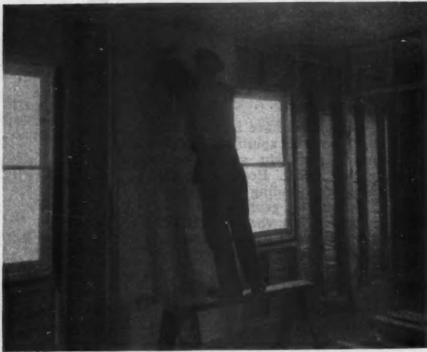
Applying a New Wood Fiber Wallboard Which Serves Both as an Insulation and as a Plaster Base.
