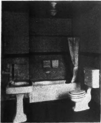
These Walls Are Covered with a Material Very Closely Resembling Marble but Available at a Much Lower Cost.
