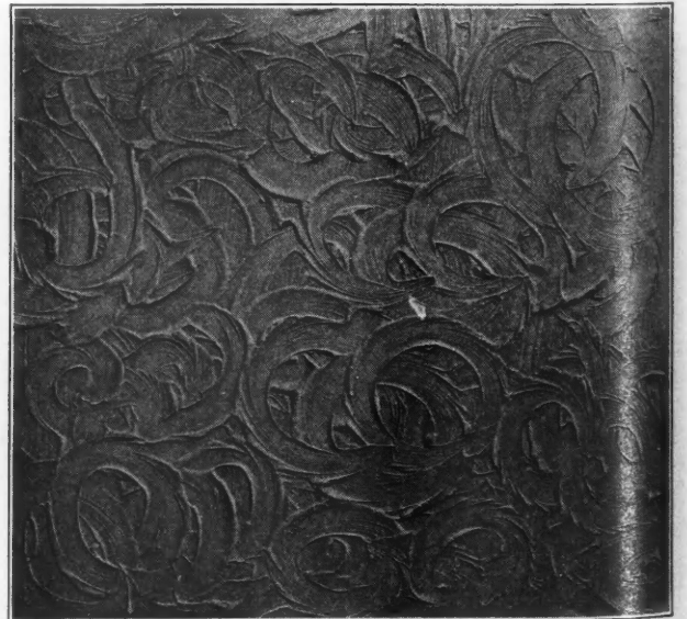
Figure 4—An Unusual Effect but Very Simple to Produce with the Curved Back of a Serving Spoon.
