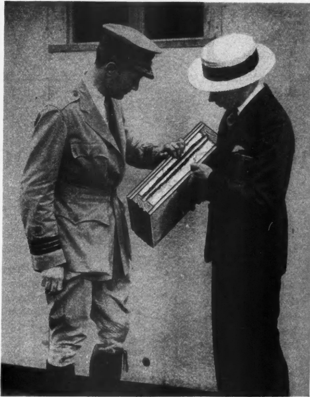
Commander Richard E. Byrd and His Architect, R. F. Barratt, Inspecting the 6-Ply Insulation in a Section of the Walls of His Antarctic Houses.
