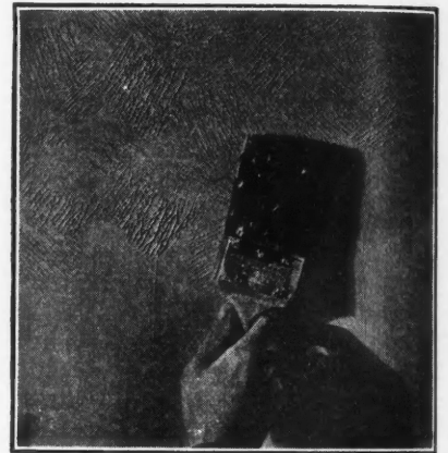
The Effect Shown Above, in Figure 9, Is Produced by Slapping the Flat Side of a Brush Against the Wet Plastic.
