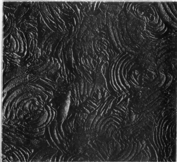
Figure 8—A Swirled Finish That Is Quite Popular and Is Made with a Dry Brush with a Circular Motion.
