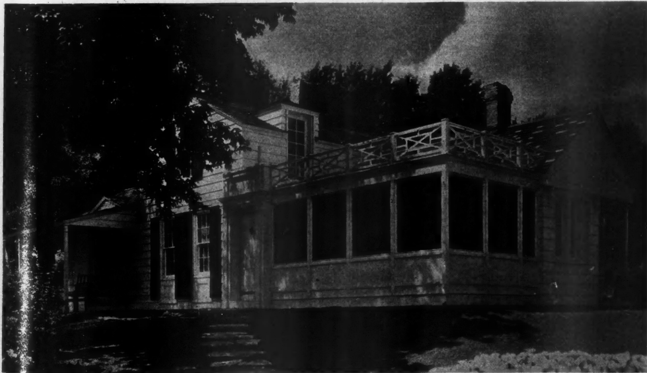
After a Thorough Dose of Modernization, with the Capable Aid of the American Farm Bureau Federation and the National Lumber Manufacturers Association, the Run-Down Farm House Was Truly Transformed Into a Thing of Modern Beauty and Comfort Which Every Member of the Family Was Proud to Call Home.
