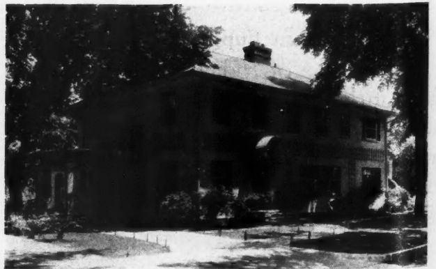
This House Has Been Painted with a New, Cold Water Paint Which Can Be Applied by Hand or Spray Gun to Any Clean Masonry Surface.
