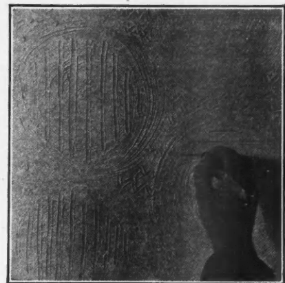
The Novel Finish Illustrated Above, Figure 6, Is Accomplished by Means of a Wad of Cloth and a Blunt Stick or Other Tool.
