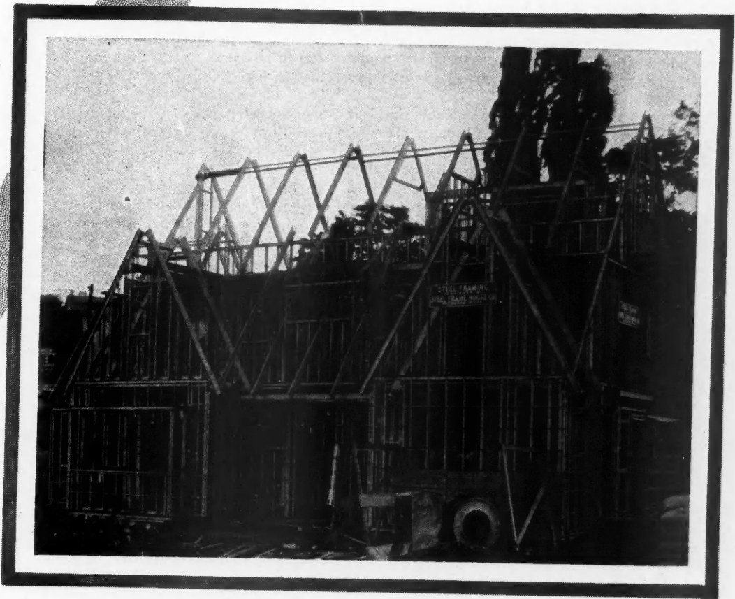
This is the Steel Frame for the Shaffer House—pictured in colors on the Cover of this month's issue of the American Builder
