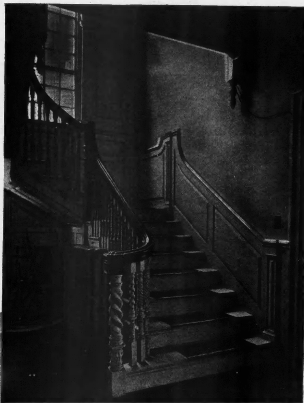
Stair hall in the Vernon House, Newport, Rhode Island. This home, built in 1758, is an interesting example of the use of Pine woodwork in one of the nation's early homes.
