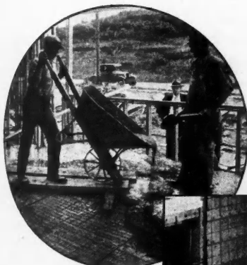
STEELTEX for interior Plaster, attached to the steel framing, gives automatic back-plastered, reinforced construction, plus insulation and sound-deadening.
