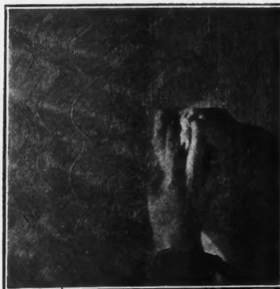
Showing How the Interesting Texture Shown at the Left, Figure 1, Is Worked by Means of a Wad of Cloth.
