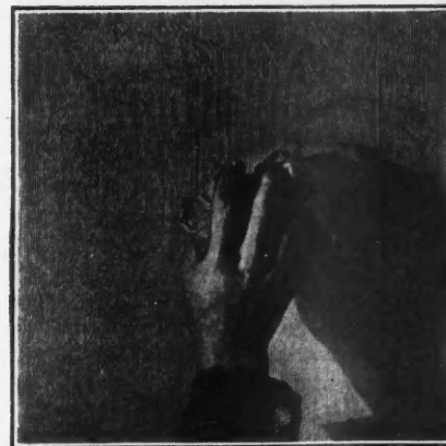
Producing the Crumpled Roll Effect Shown Above, Figure 2, in Plastic Paint with a Wad of Crumpled Newspaper.
