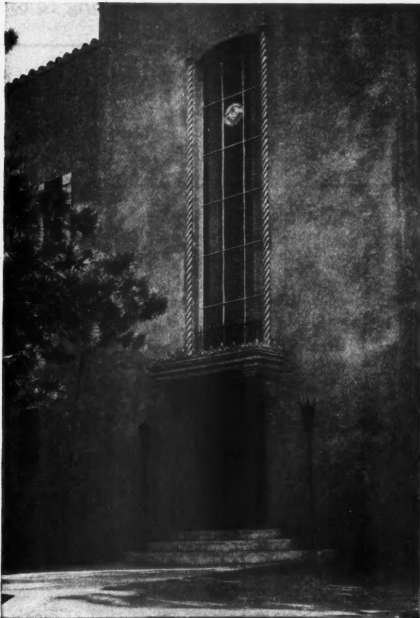
Close-Up Photo of the Entrance of the Eagle Rock Masonic Temple. Notice how closely the finished building follows the architect's preliminary sketch.
