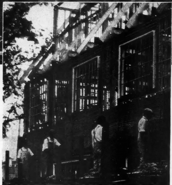
Showing Fenestra Steel Casements in the Steel Frame House Company's demonstration house now under construction at Mission Hills, Mt. Lebanon, Pittsburgh. Architects: Lyon & Taylor, New York City. Housing Engineer: Louis Brandt, Pittsburgh, Pa. Contractor: L. O. Maines Construction Company, Pittsburgh, Pa. Owner: W. H. Shaffer, Jr., Pittsburgh, Pa.
