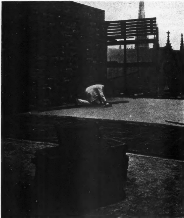
Insulation Board of Specially Treated Pressed Peat Used on Roof of the Patriotic Building, Hamburg, Germany. This material also selected to insulate roof of Steel Frame Model Home, Pittsburgh.
