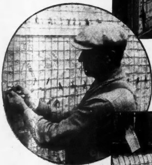
STEELTEX for Brick Facing provides a 1-inch reinforced cement slab, cast in place as the bricks are laid, forming a monolithic, moisture-proof wall of brick, steel and cement. Wall ties, hooked to the STEELTEX, are embedded in mortar.
