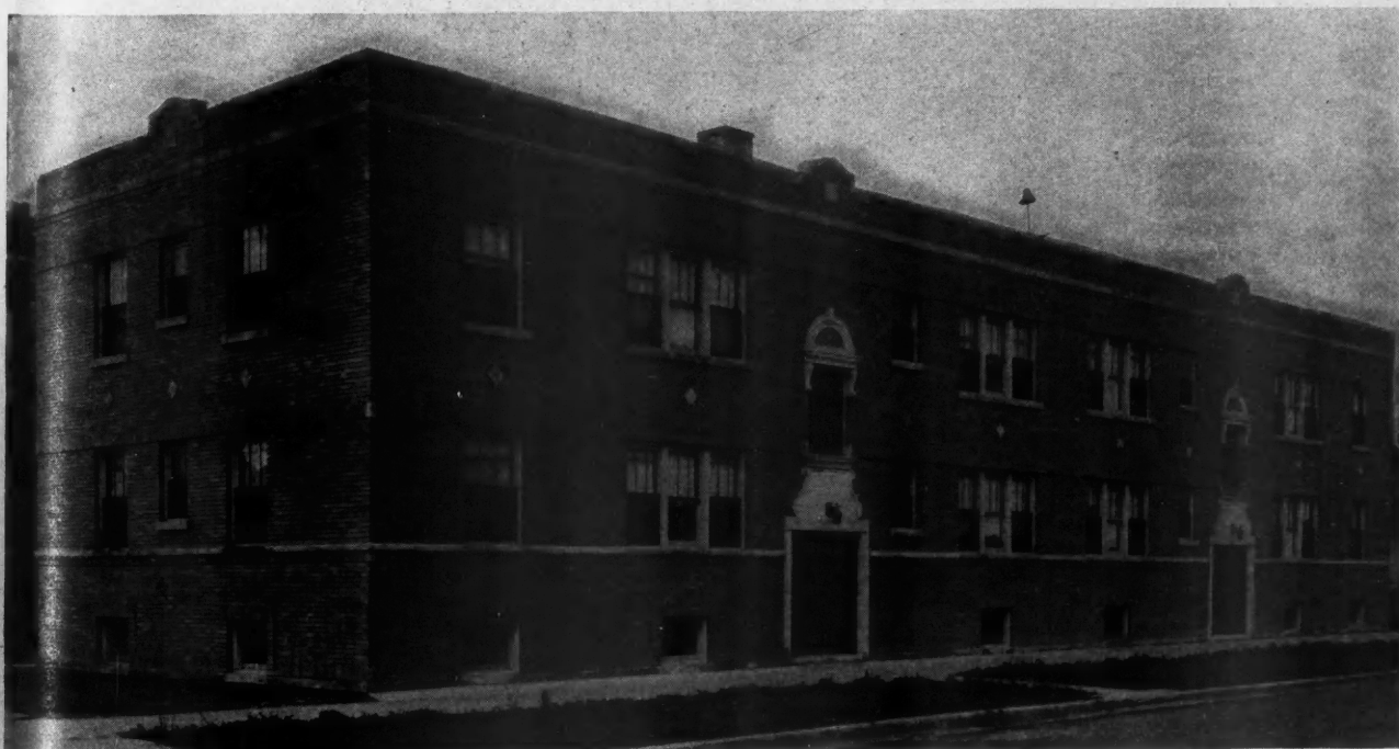
Photograph and Floor Plan of Inexpensive Yet Good Income Building on North Lockwood St., Chicago. Bernard L. Roos, Architect.
