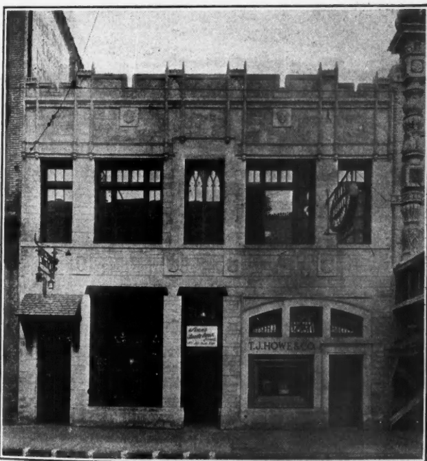
Store front, Louisville, Ky. Faced with Sawn Indiana Limestone Random Ashlar in combination with decorative cut-stone trim. C. J. Stinson, Architect.
