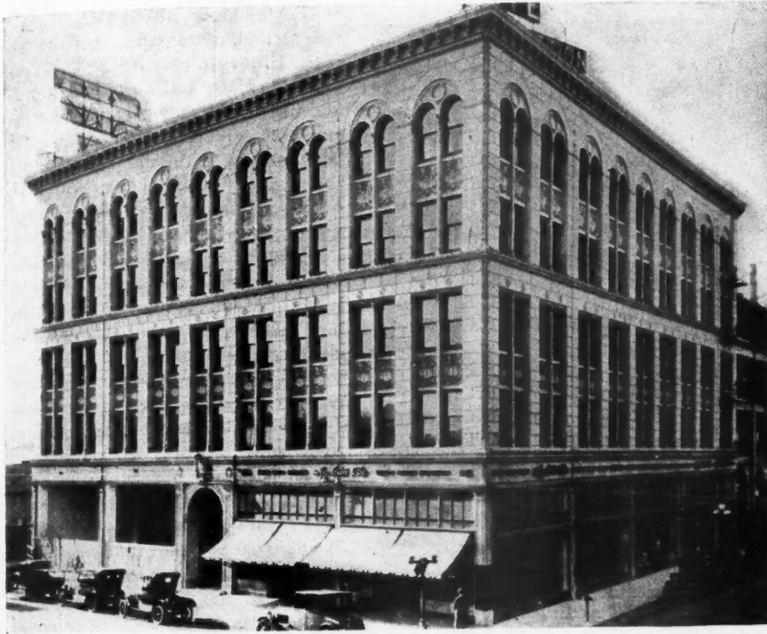
In Buildings of This Sort the Water-Cement Ratio Method of Mixing Concrete Has Superseded the Less Scientific Methods of a Few Years Ago with the Result of Stronger, More Uniform Concrete.
