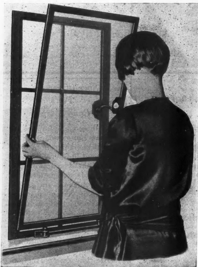
The Screen Is Held in Place by Clips Which Permit It to Be Quickly and Easily Removed When Desired.
