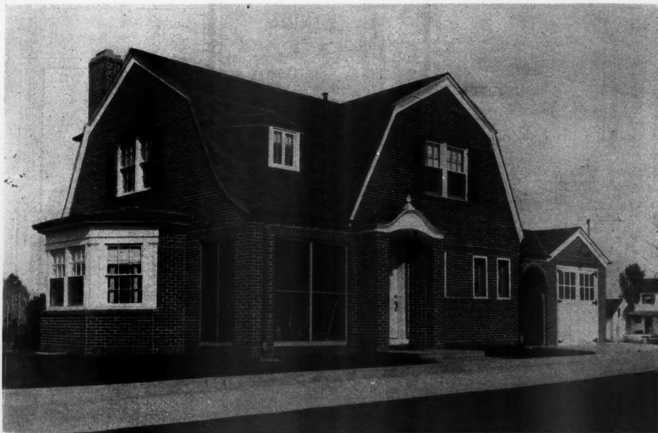
This Attractive All-Feature Home if Built from Plans as Shown on the Next Four Pages Will Provide for All Those Specialties Which Are Today Considered an Essential Part of Any Really Desirable Home.
