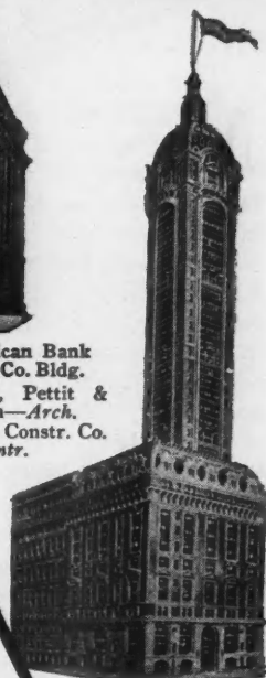
Singer Sewing Machine Co. Building Ernest Flagg— Arch. A. C. Holm & Co. —Contr.
