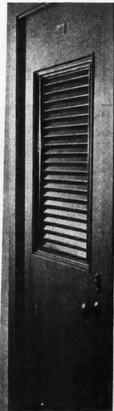
Ventilating Panels in Doors Eliminate Transoms and Permit the Economy of Lower Ceilings as Well as Other Advantages.
