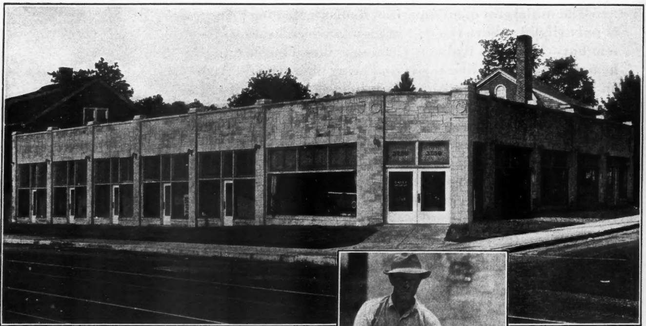
Group of stores, Indianapolis, Indiana. Faced with Sawed Variegated Indiana Limestone Random Ashlar. E. H. Dalby, Designer and Contractor.
