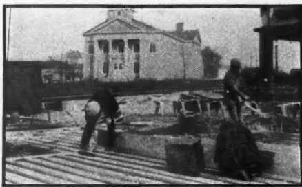
Laying sleepers over concrete first floor.
