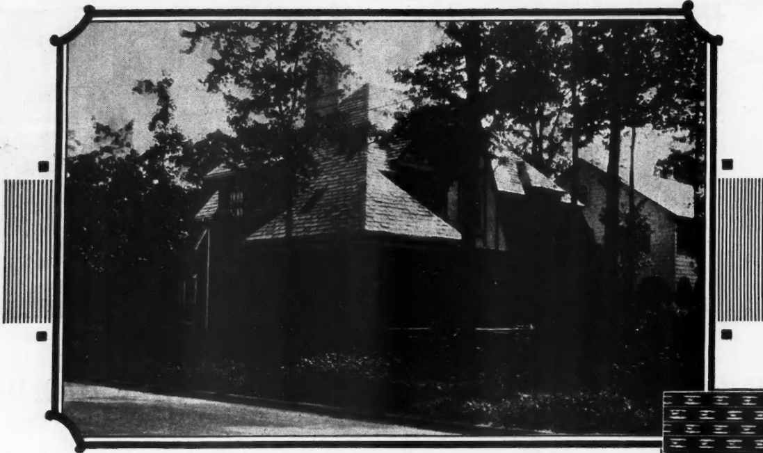
Residence, Winston Salem, N. C.—H. W. Nash, Contractor & Designer
