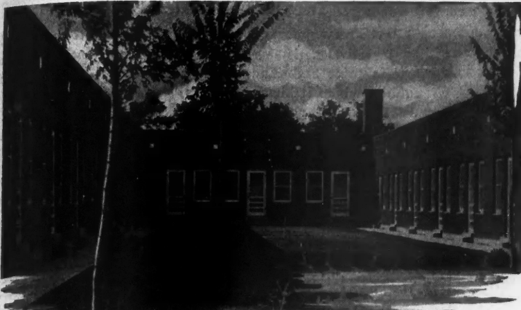
250 Andersen Frames used in this apartment building at Albuquerque, New Mexico, built by T. W. Plunkett.
