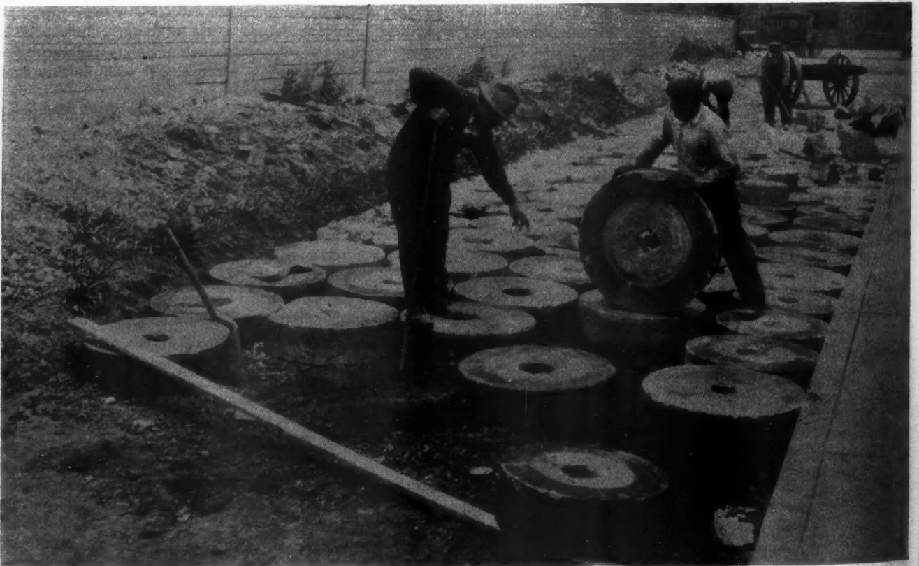
A GRINDSTONE ROAD Built of Stones Worn Down Making Hand Saws. The spaces between stones are filled with concrete. The road is standing up well under heavy truck traffic.
