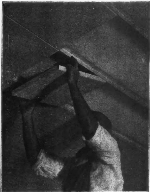
METAL TILE, Filled with Sound-Absorbing Material Have a High Acoustical Rating.
