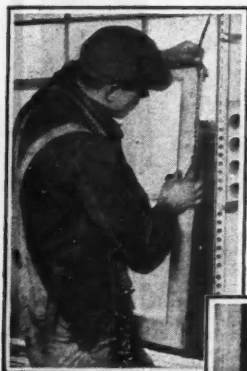
Sash is anchored with simple coil
