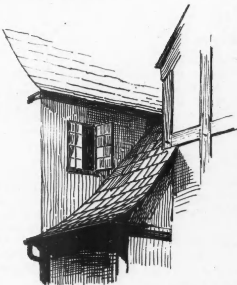
FIG. 1 CURVED PORCH ROOF
