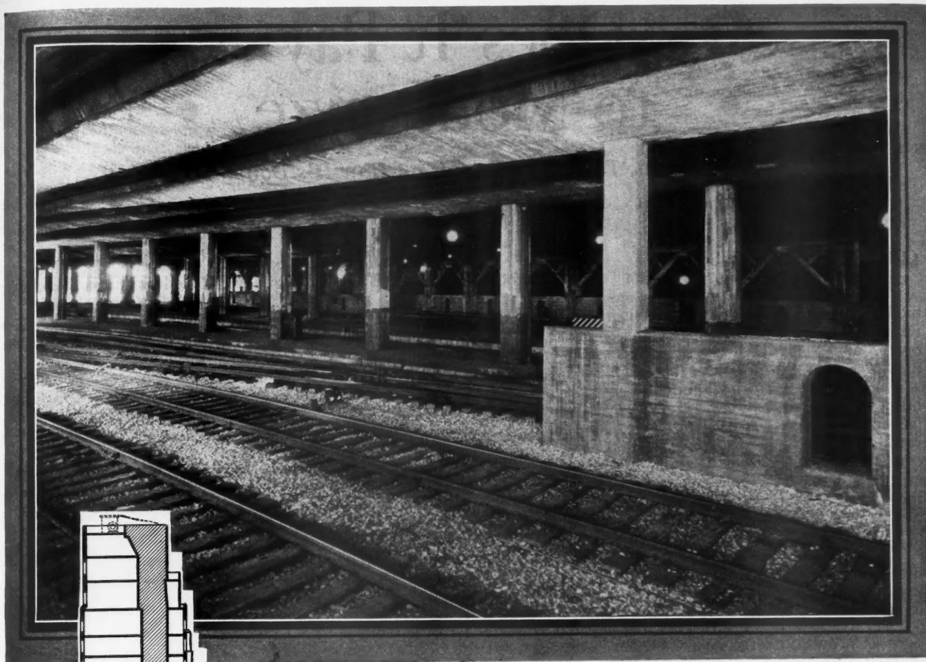
Photo of Track Area Under the Daily News Building. Note exit for smoke above each track.
