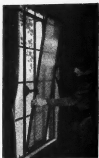
Screens easily and quickly removed or replaced from the inside.
