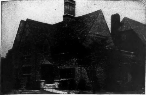
This charmingly designed home at 11 Cranford St., Forest Hills, L. I. is the tenth STEELTEX-reinforced job built—and sold as fast as completed—by Guyon L. C. Earle, Inc., Forest Hills. The NEW RIBBED STEELTEX reinforces its interior plaster with a welded fabric of rustproofed steel, on guard against all strains.
