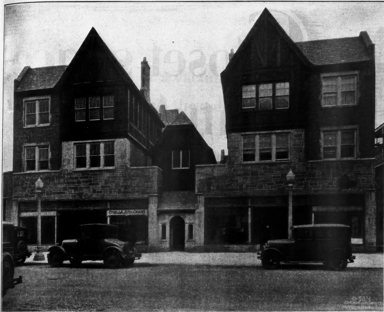
Stores and Apartments, Chicago. A. G. Lund, Architect. Old Gothic Indiana Limestone Random Ashlar.
