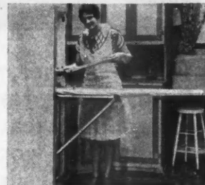
The door to the broom closet serves a double purpose. Just release a catch, and down comes a sturdy ironing board adjustable to the proper height.
