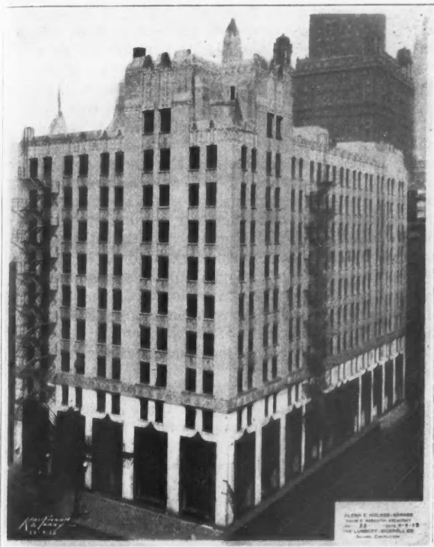
The Glenn E. Holmes Garage, Chicago; Davis D. Meredith, Architect.
