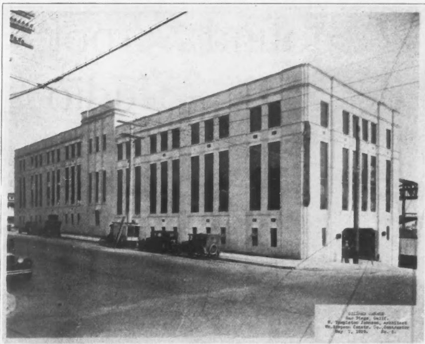
The Gildred Garage, San Diego, Cal., W. Templeton Johnson, Architect; Wm. Simpson Construction Co., Builders.
