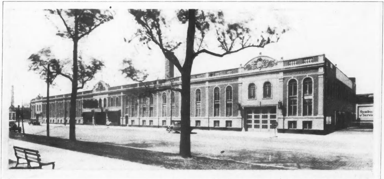
The Gateway Garage, 56th St. and Stony Island Ave., Chicago; John Hocke, Architect.
