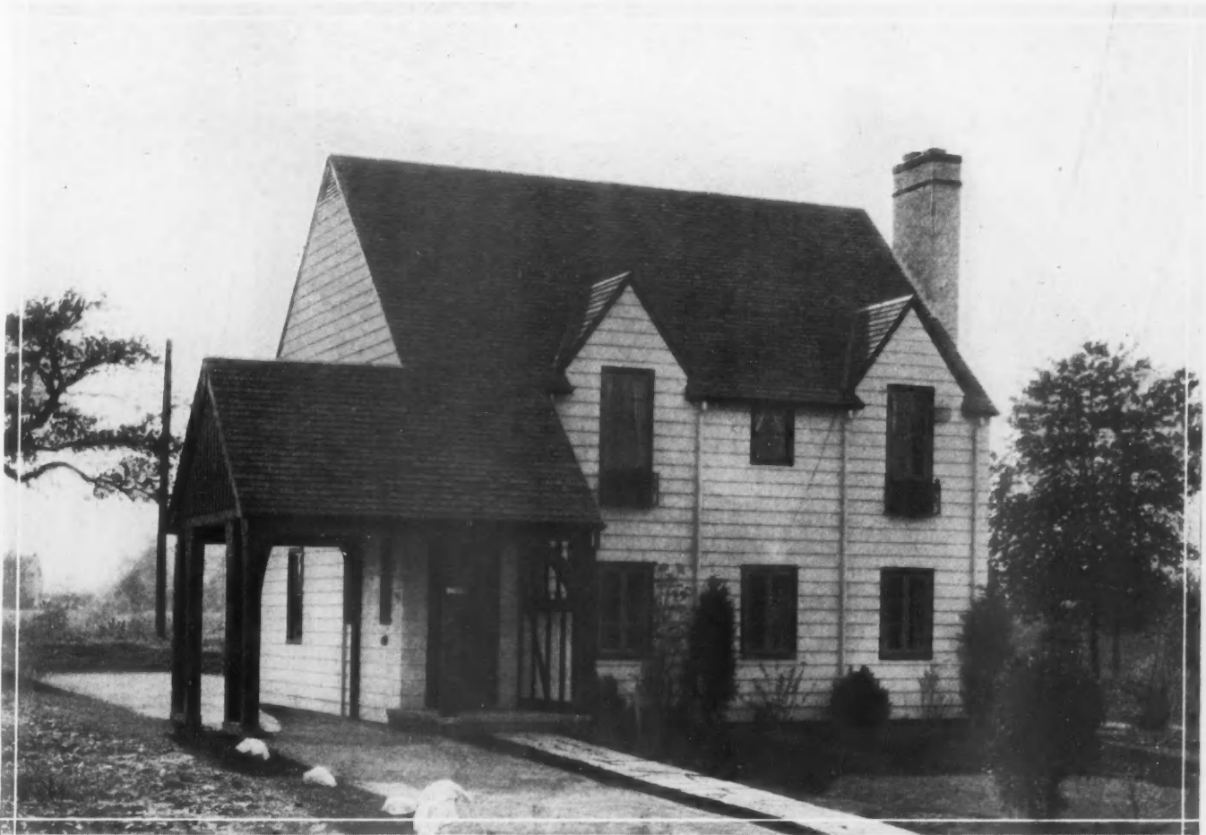
A. R. PHILLIPS COMPANY, Builders
