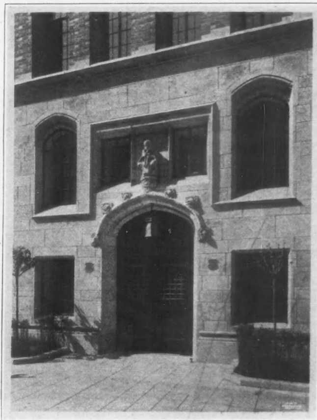
Detail of Entrance, Sherman Square Studios, W. 73rd St., New York.
