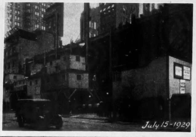
Below: View of Wall Street End July 15th. Opening between the two sections of sidewalk sheds is to provide space for material trucks to go through; all material had to be deposited within confines of plot.
