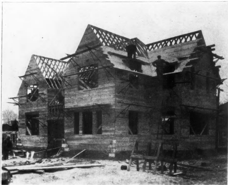
Scaffold Brackets of Steel Are Handy, Light and Safe.
