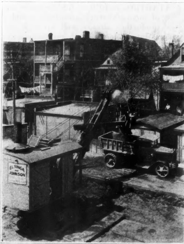
The Power Shovel and the Motor Truck Are Indispensable in Excavating.
