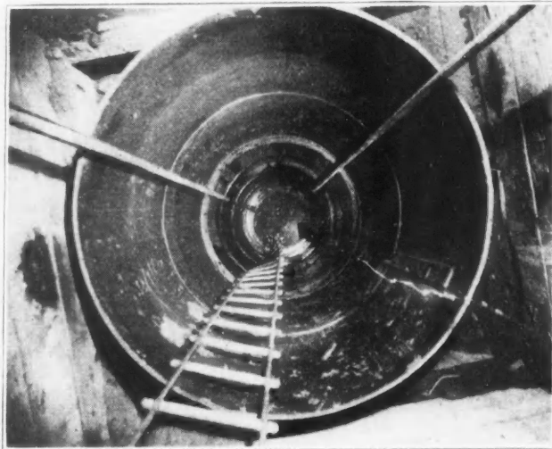
Looking Down Cylinder Caisson 80 Feet Deep Under Old Bank of Manhattan.
