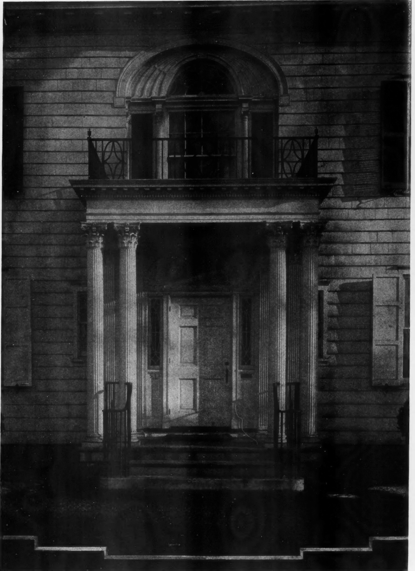
P URE Colonial Styles Still Appeal to the Discriminating. This stately entrance with its Corinthian columns and wrought iron work is a model.
