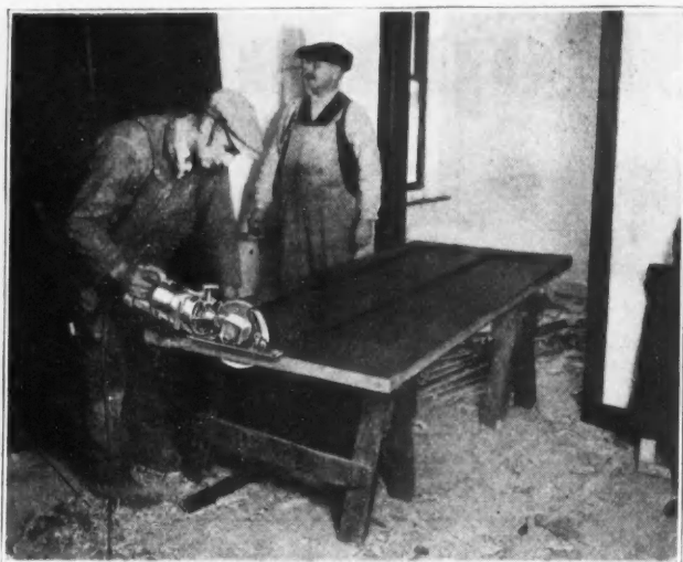
Power Hand Saw Does Fast Work Fitting Doors.
