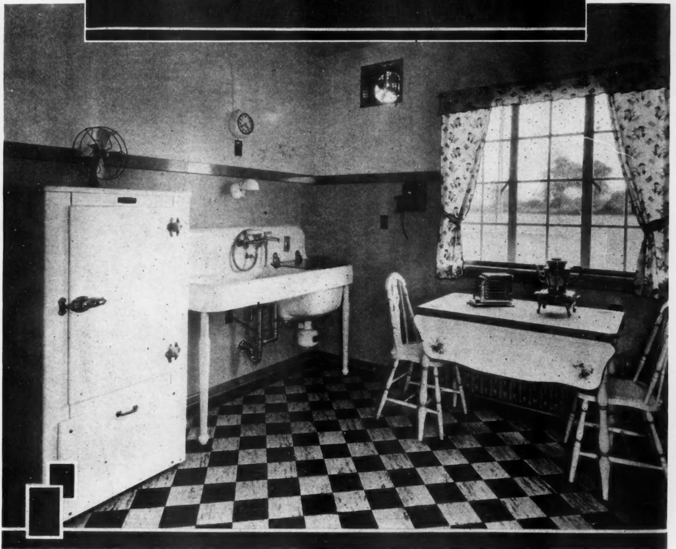
Color, Electrical Labor Savers, and Built-in Cases and Equipment Characterize the Modern Home Kitchen.
