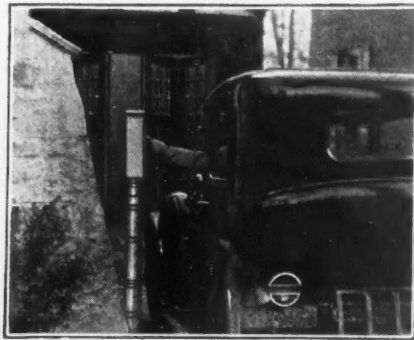
A Switch Beside the Driveway Operates the Doors Without Getting Out of the Car.
