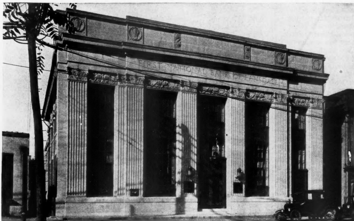
A Simple Job of Refacing with Indiana Limestone and Remodeling the Front Completely Changed the Appearance of the First National Bank, Lansdale, Pa., as May Be Seen by Comparing This View with the One at the Top of the Page. Tilghman Moyer Co., Architects & Engineers.
