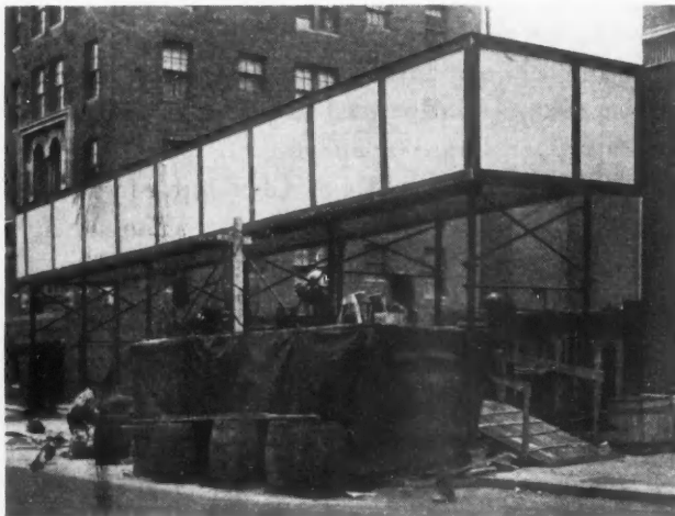
A Tubular Steel Supported Sidewalk Shed.
