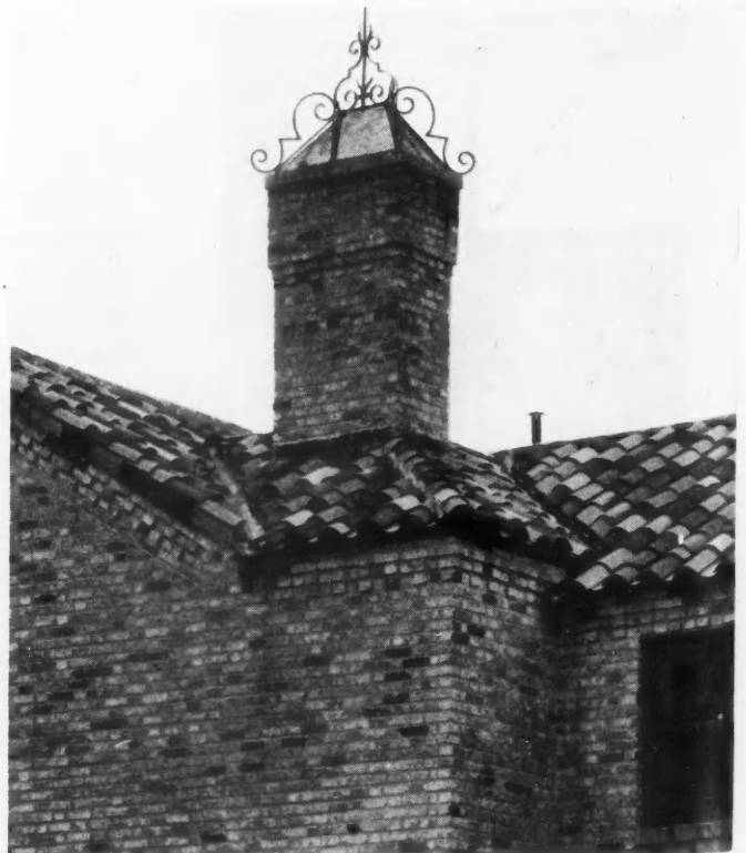
A Spark Arrester of This Sort Serves as an Artistic Finial for the Incinerator Chimney.
