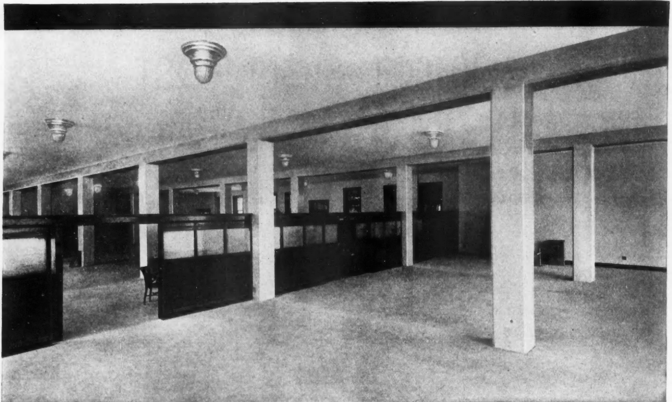
Concrete columns and floors at the newly remodeled Saddle & Sirloin Club, Chicago; high-early-strength concrete made with Universal Atlas methods and cement used in the construction. Poirot Construction Co., Chicago, contractor.
