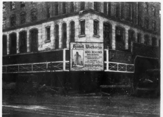
Sidewalk Shed That Presents a Neat Appearance.
