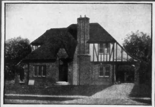
Model home at Amarillo, Texas. Architects: Berry and Hatch; Andersen Master Frames No. 604 from Amarillo Sash & Door Company
