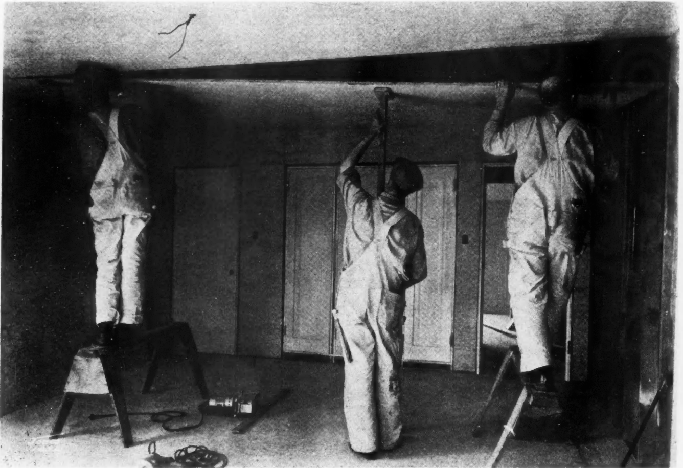
More Than 100 Square Feet of Ceiling Completed at Once! Lower costs should come when workmen become familiar with the technique of handling these big panels.
