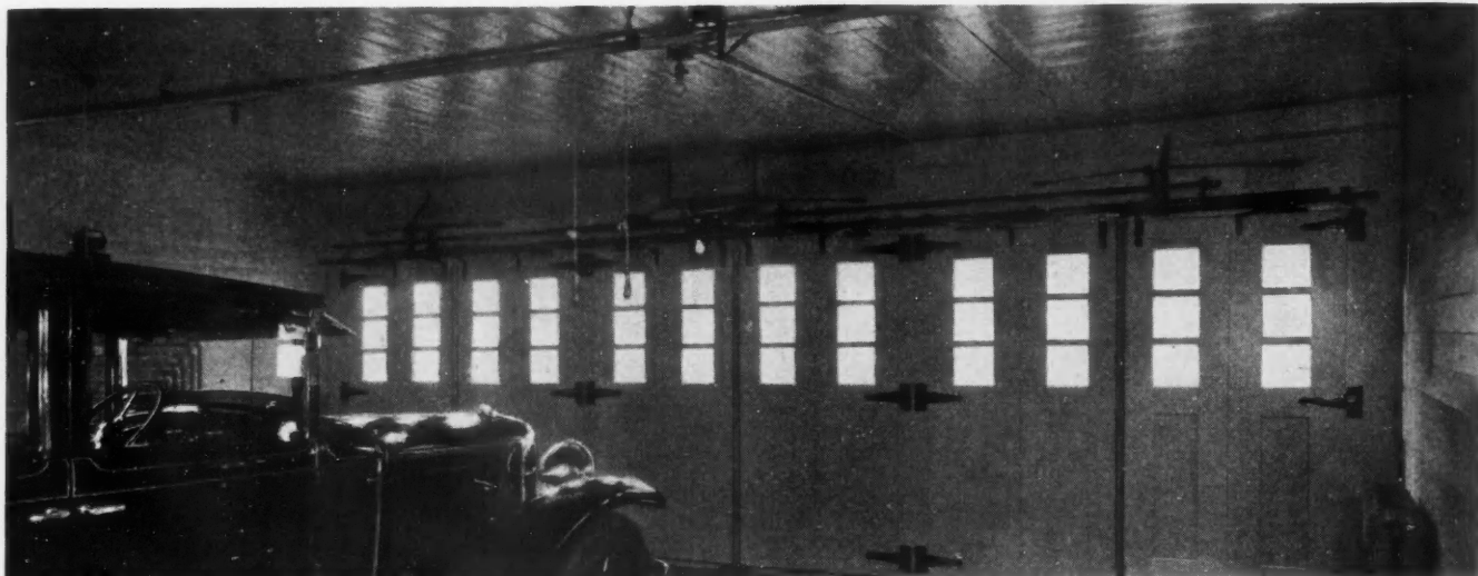
Motor Operation Can Be Applied to Almost Any Type of Door and Is Sometimes Controlled by a Convenient Pull Cord as in this Installation by the Beeman Door Control Co.
