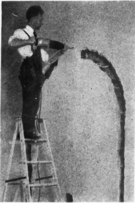
Clean Cutting Through Plas- ter and Tile.
