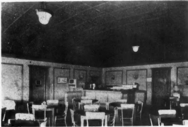
Fiber Insulating Board Applied to the Ceiling Solved the Noise Problem in This Grill Room.
