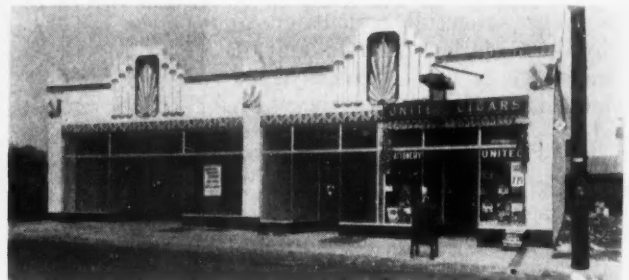
A Close-up View of the First Section of Market Street Buildings Already Erected. Note the modernistic note in these terra cotta store fronts.
