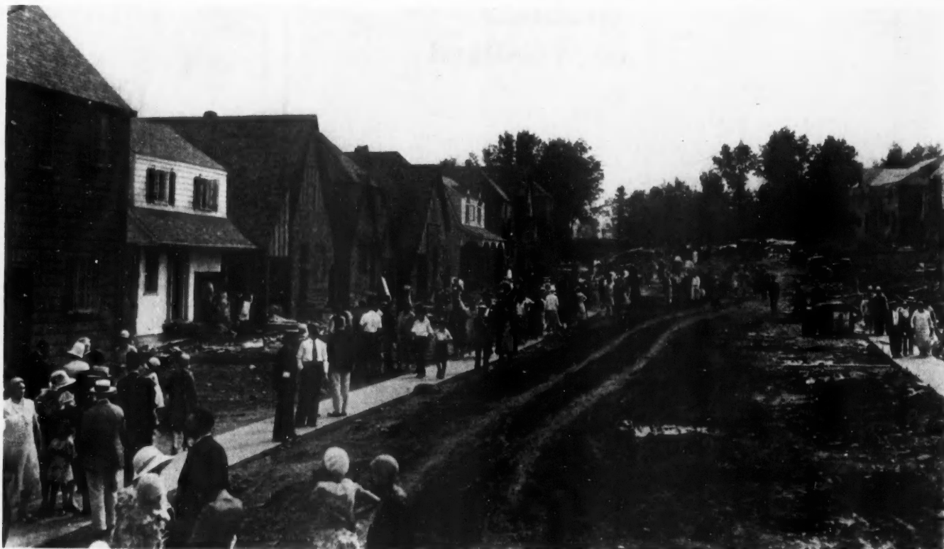
Marlboro Road While Under Construction Was a Mecca for Interested Visitors. This picture was taken before any of the "Model Home" opening days or before any advertising appeared. The reinforced concrete street and curbing have not yet been placed.
