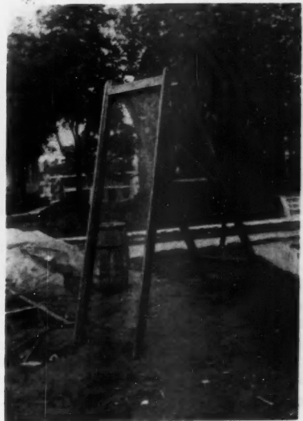
SAND SCREEN used by John Hill, Pittsburgh, Penn. Lightweight, easy.
