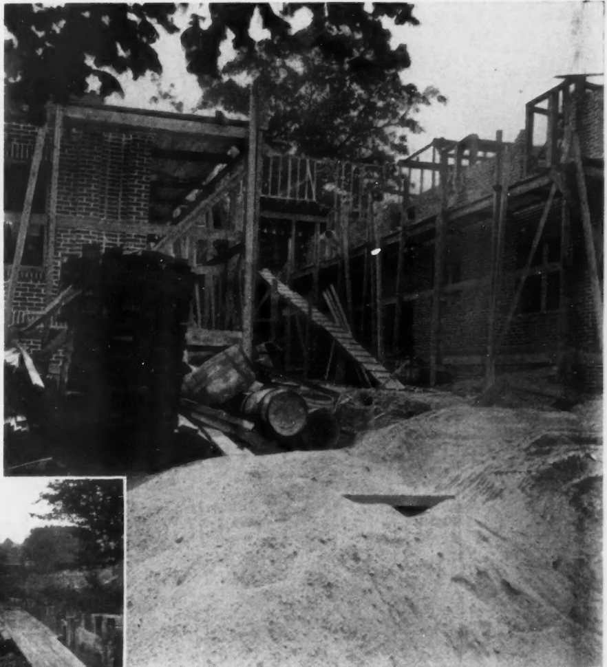
LONG RUNWAY placed for use of hod carriers instead of ladder. Enterprise Building Company, erecting apartment building in Providence, R. I.
