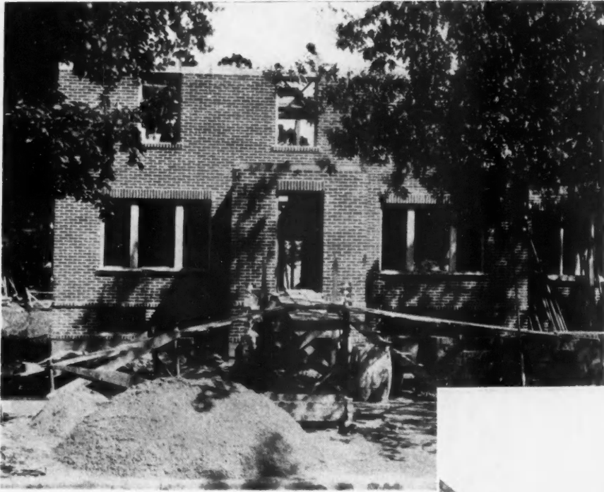
BRANCH INCLINE facilitates handling of materials on this Madison, Wisconsin, job of the Way Building Company.
