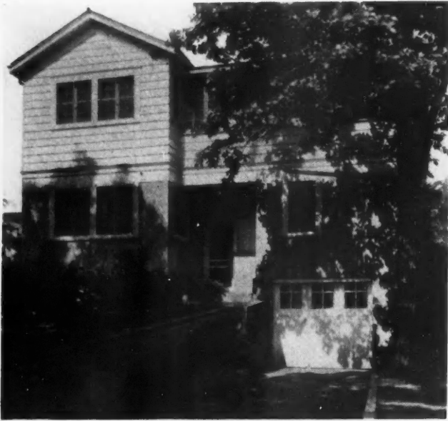
A Basement Level Garage Requires Proper Drainage to Prevent Accumulation of Water at the Entrance. A Beeman Door Control Co. installation.
