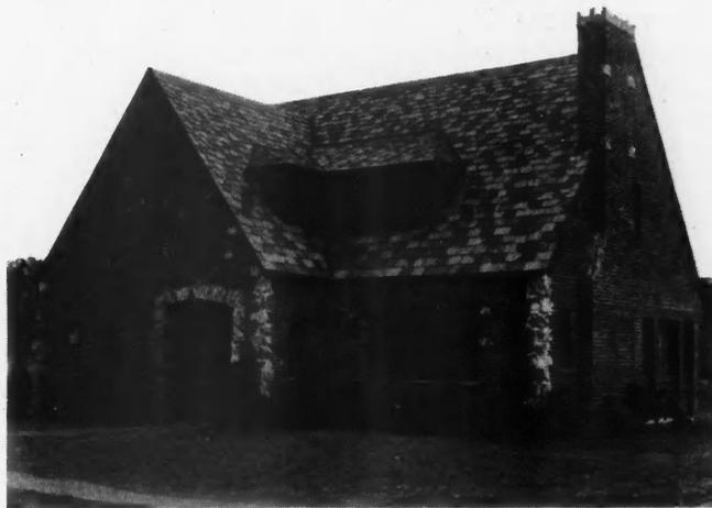
Fireproof house of special construction with walls of hollow masonry blocks and with outside wall of brick veneer. Steel joists support concrete floors. This type of house illustrates the possibility of reducing costs through the application of new materials.
