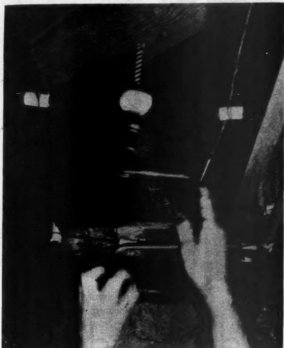
The Rubber Ball Cup Catches the Borings Instead of Letting Them Fall Into the Workman's Eyes.
