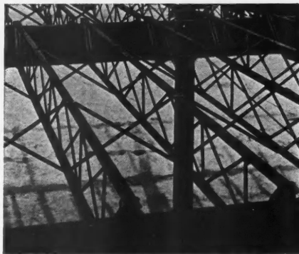
Section of typical floor in course of construction showing use of Kalmantruss Steel Joists laterally braced with Kalmantruss Rigid Bridging.
