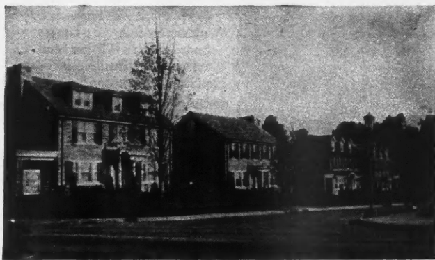
Four Houses in the Charles Armstrong Development, Philadelphia, Pa. Roofed with Cabot's Stained Shingles, Stained with Cabot's Creosote Shingle and Wood Stains and laid in variegated patterns.
