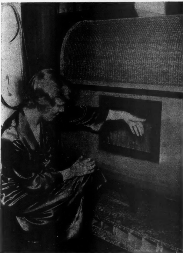
The home air is forced through a series of fine swirling water sprays which wash out practically all of the dust and impurities. The water sprays not only clean the air but are a means for winter humidification and summer cooling.
