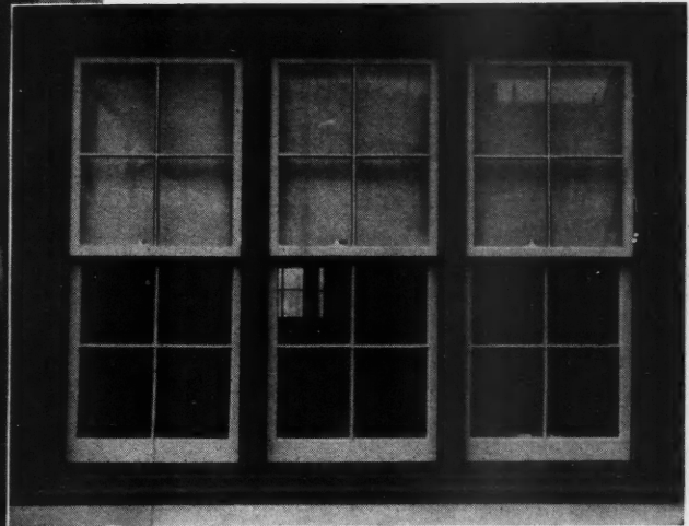
The narrow mullions give improved appearance both inside and out.
