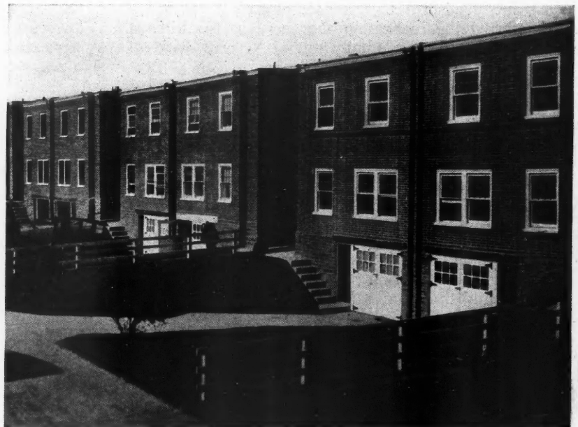
A rear yard of more than forty feet in depth is provided. The cellar garages are reached over driveways of concrete.
