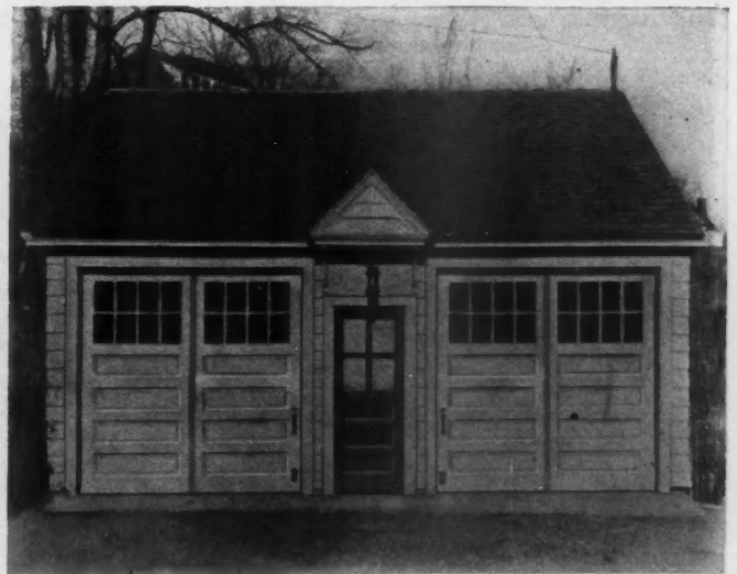
An old garage modernized and equipped with Stanley "Swing-Up" hardware. Before change doors sagged so badly they would not close.
