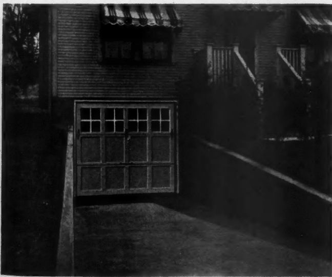
Modern upward acting garage doors by Farley and Loetscher Co. Installed in an old house. The modernized basement garage is a popular type.
