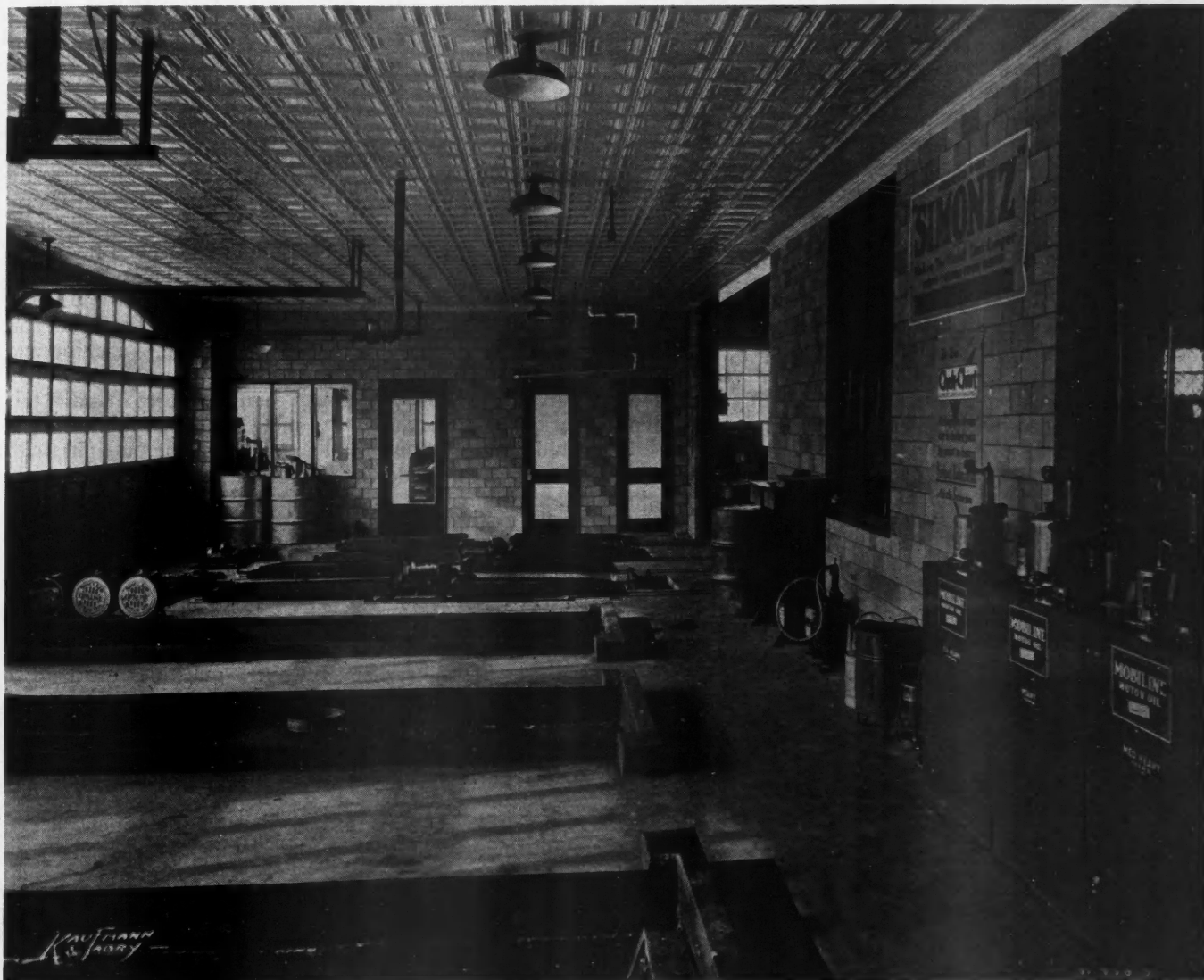
Interior view of greasing pit and brake service section at the front of old-style public garage on 79th Street, remodeled by E. J. Biggs Construction Co., Chicago.
