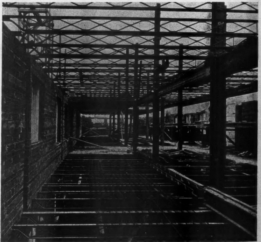
Showing the floor construction in the Lowrance Hospital. Note the use of Kalmantruss Steel Joists, Kalmanlath, and accessories.
