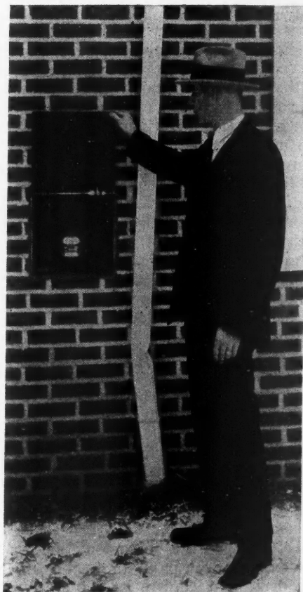
The proper place for the electric meter is outside the house.
