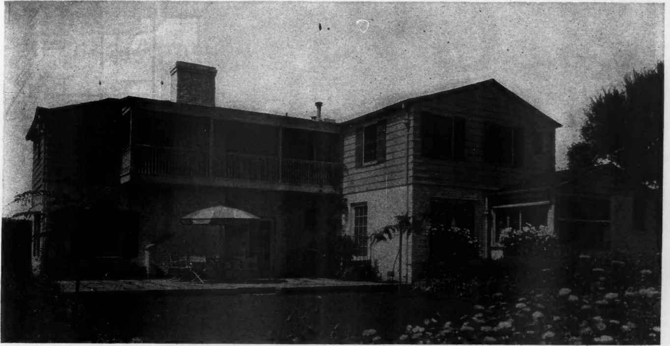
The J. B. Murray Residence in Brentwood Heights, Calif. John Byers of Santa Monica, Architect.
