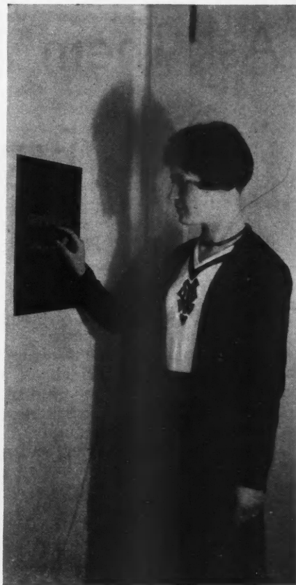
New style load center in the kitchen, very accessible.
