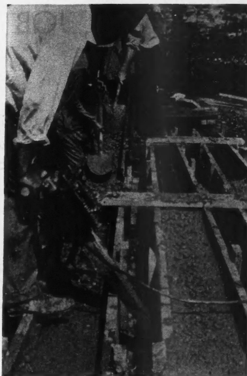
Vibrating concrete into a dense mass in forms with new electro-magnetic tool.
