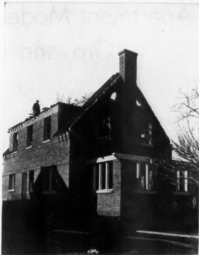
PICTURE TAKEN early in March showing face brick house in Chicago under construction. It cost 33 1/3 per cent less this spring than it did in 1925. Below is shown architect's drawing. The exterior and plan have been the most popular design of the American Face Brick Association.
