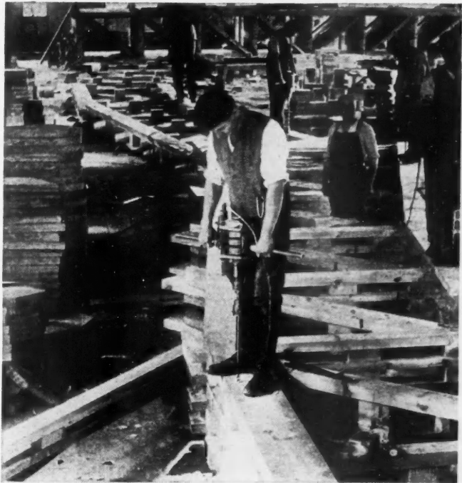
Pre-fabrication and shop assembly of trusses, paralleling steel shop practice.
