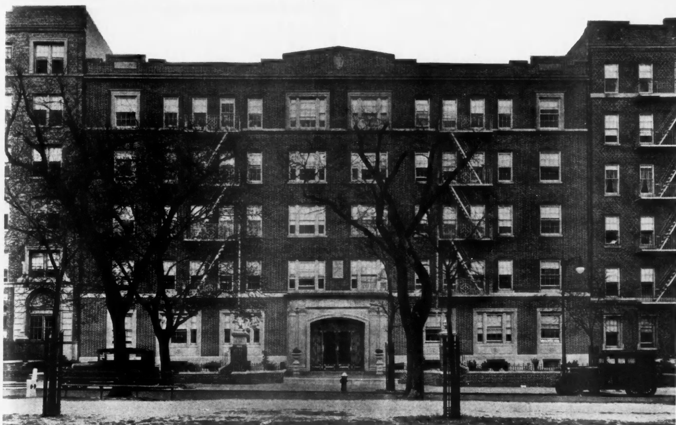
Abraham M. Kaplan, Brooklyn contractor and builder, increased the rental income of this 4-story and English basement apartment $14,000 a year by modernizing and installing two automatic push-button elevators. People would not walk up.
