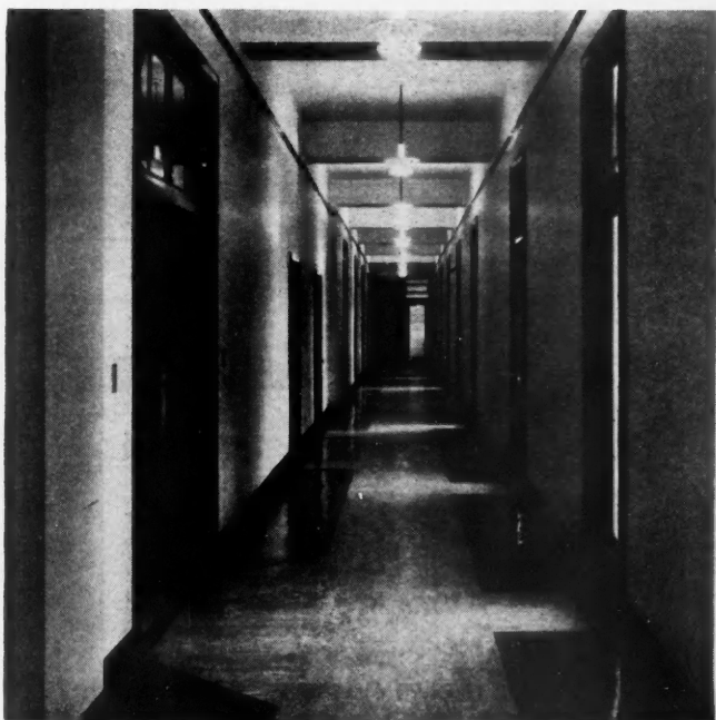
Rubber tile flooring in corridor of General Motors Building, Detroit
