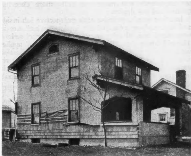
For needed repair and to improve appearance, shingles are popular. Photo above shows interesting example of wood shingles being used to over coat stucco.
