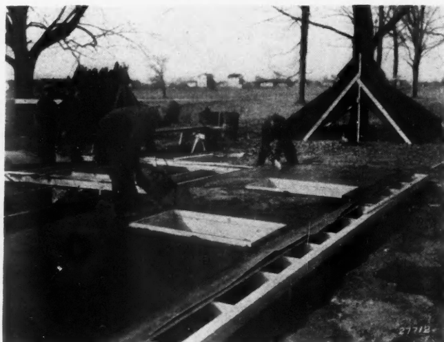
A CONTRACTOR, ARCHITECT, lumber dealer, realtor and business man of Middletown, Ohio, get together to plan an experimental house. Below is shown corrugated steel section to which stucco is applied by asphaltic binder.
