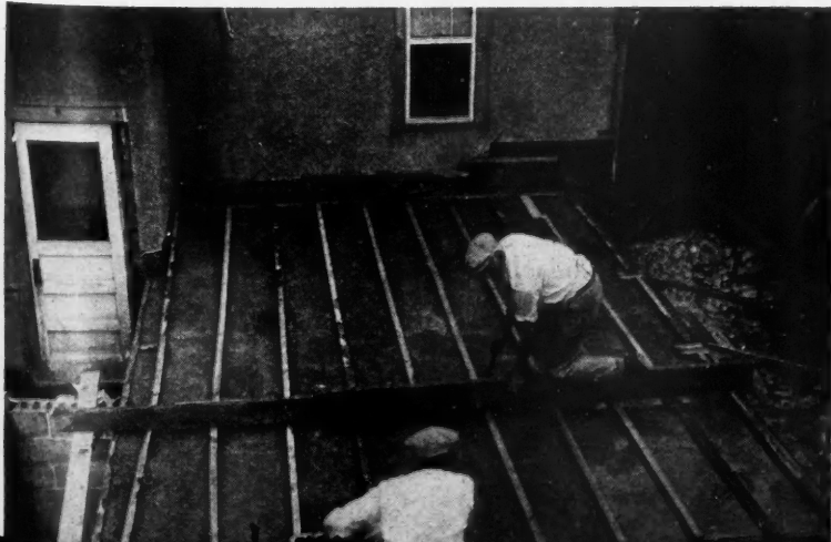
7—Sleepers placed at right angles to joists.
