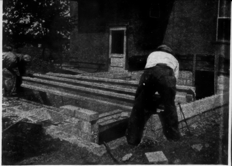
2—Placing precast concrete joists.
