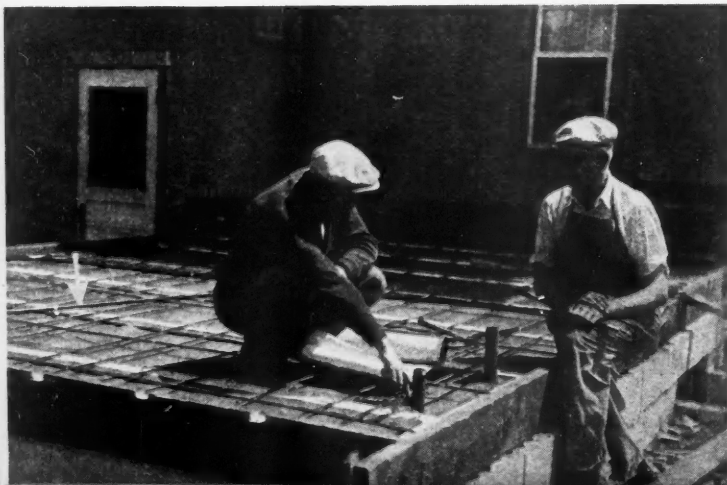
5—Completing floor forms.
