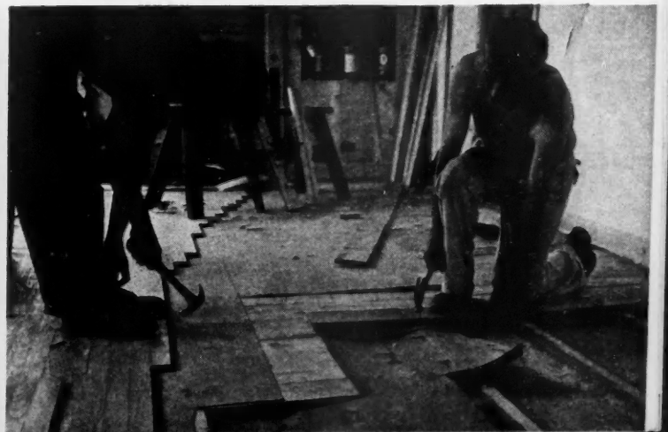
8—Laying wood floor.
