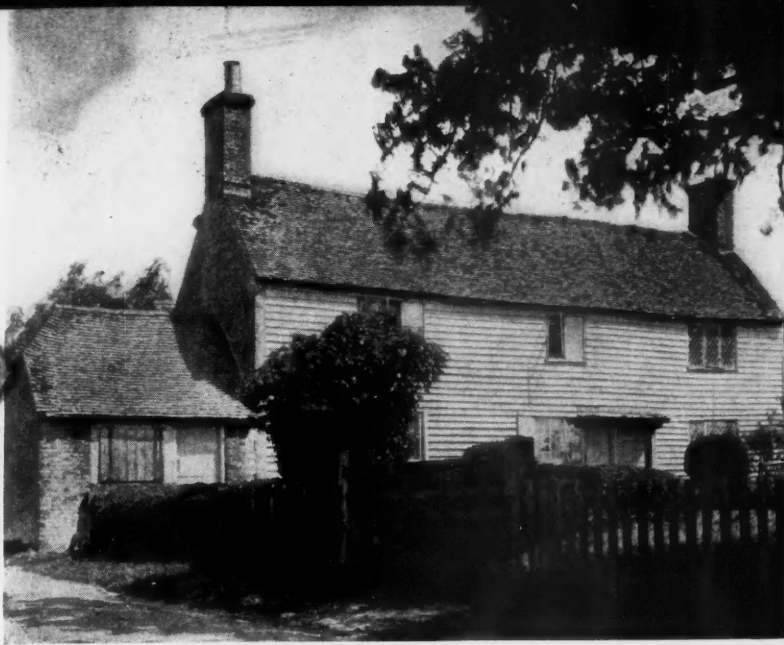
OLD FARM GROUP near Battle, England. One of the few remaining early examples of wood houses in England. Note one brick end.
