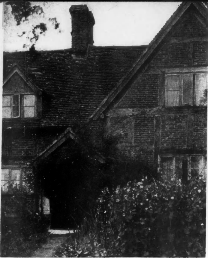
OLD HOUSE, Whiteparish, England. An interesting example of brick filled timbering; unfortunately, from an architectural viewpoint, the original leaded glass windows have been replaced by large pane sash.
