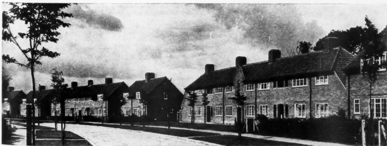
AN EXAMPLE of subsidized public housing in England built to rent, in famous Welwyn Garden City, near London. Rooms are small, with little equipment. In the foreground are flats for elderly people, consisting of bedroom, living room, kitchen and bath, which rent for approximately $1.75 per week. In center is a 2-family house with 3 bedrooms which rents for approximately $3 a week.
