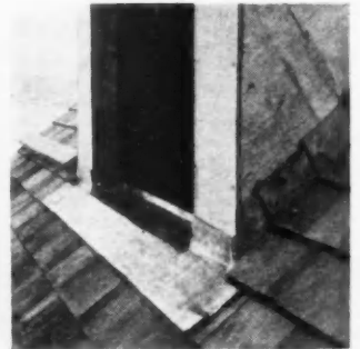
2½ LB. HARD SHEET lead flashing used at window head (left) and at dormer intersection with roof at the bottom and sides (right).
