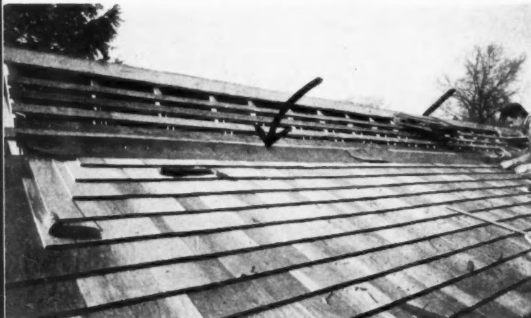
APPLYING LONG-LIFE red cedar roof. Arrow shows lead flashing installed at change of pitch above triple dormer at rear of house.
