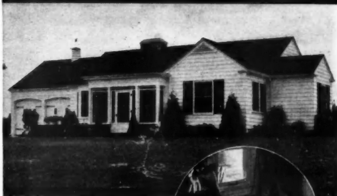
Home of Mr. and Mrs. Henry C. Forster, Jr., Bingham Road, Birmingham, Michigan, heated by U. S. Equipment.
