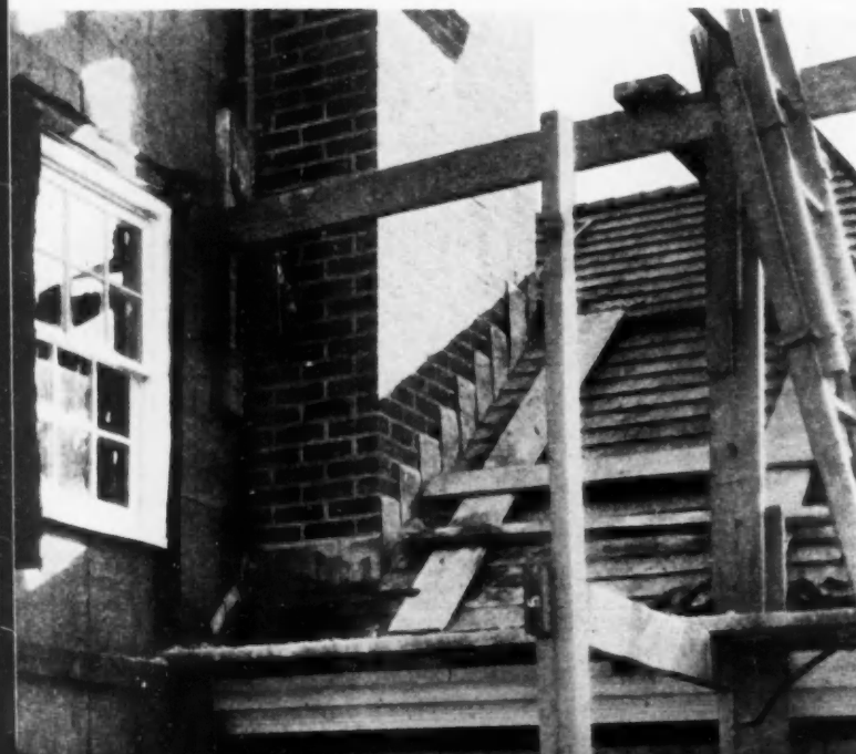
APPLYING LONG-LIFE red cedar roof. Arrow shows lead flashing installed at change of pitch above triple dormer at rear of house.
