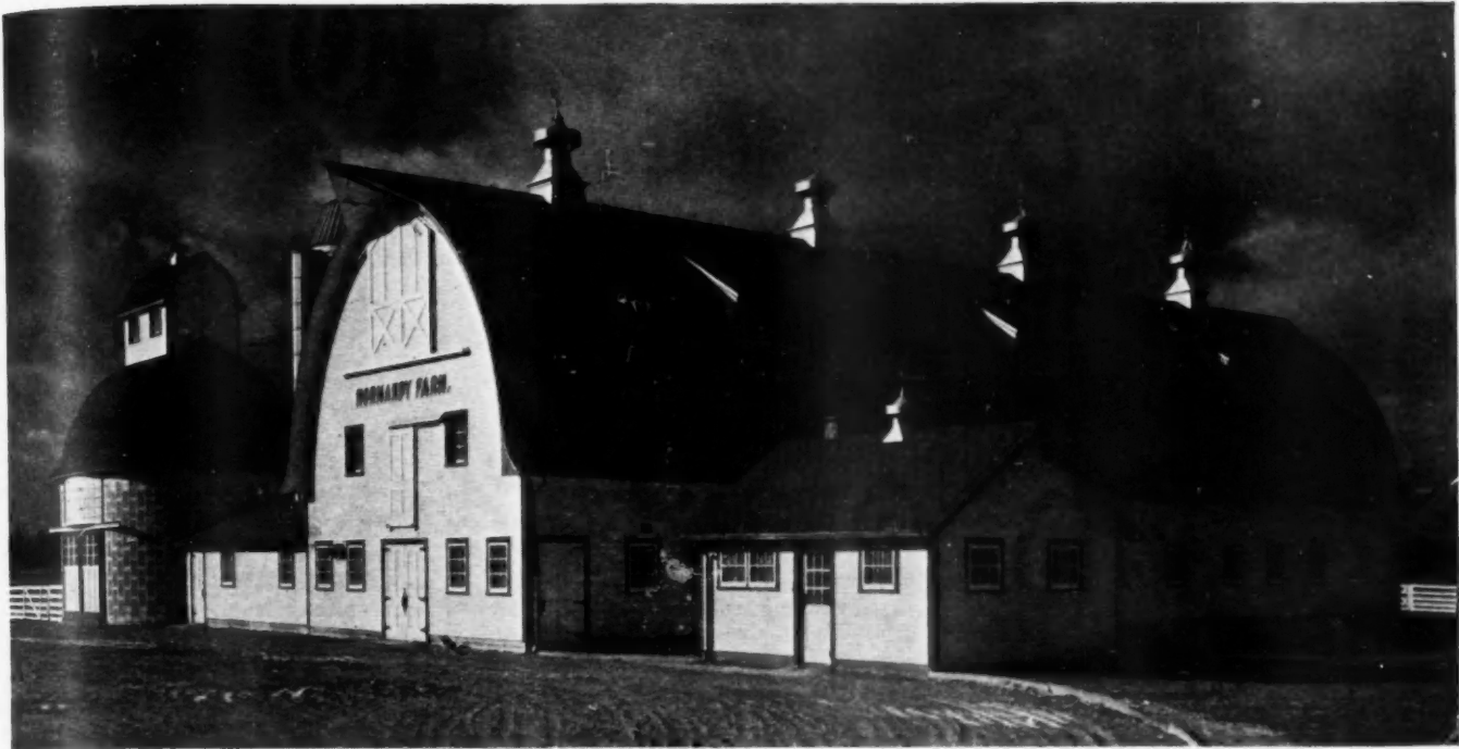
BARNs like this one near New Augusta, Ind., are the result of many hours of careful planning. Plans for barns like this are available to barn building contractor, and retail lumber dealers at no cost.
