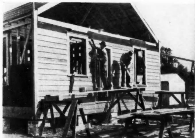
QUALITY LUMBER checked and inspected as delivered to job. National Sash and Door millwork used. AT RIGHT—CYPRESS SIDING being applied with joints and intersection painted with pure white lead and oil.
