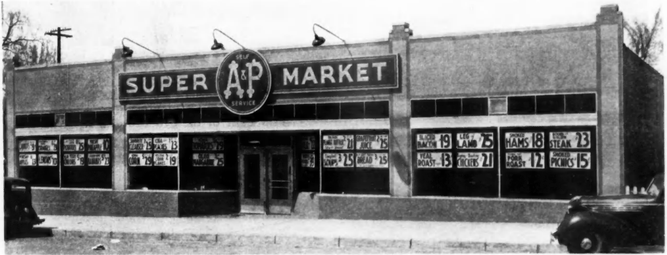
LEFT AND BELOW: Two examples of store construction using glastone units; brilliant and attractive color combinations are possible with the vitrolite facing used on this newly developed material.
