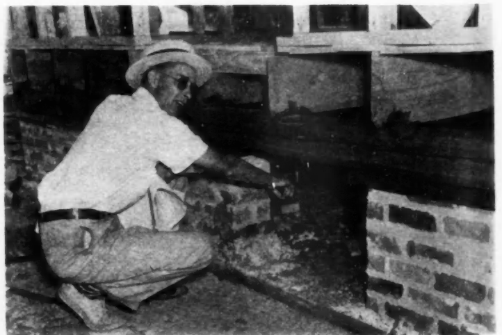
"KEY TO BETTER LIVING" is the slogan appearing on the Roger Derby direction signs above. SLATE MOISTURE-PROOF SHIELDS (at right) inserted in brick foundation wall are pointed out by the Derby sales manager. Note also the termite proofing shields below.
