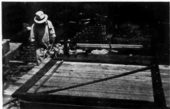
FIG. 2. Guide is turned down and electric saw cuts studs to length.
