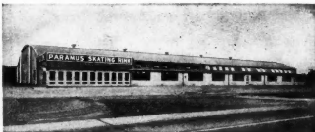
Paramus Skating Rink, Park Ridge, N. J. 220' x 120' floor area with clear span bowstring truss.
