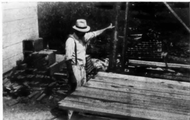
FIG. 1. Lengths of 2x4 are laid on the cutting frame.
