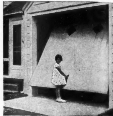
RIGHT: Hardware set easily converts swinging garage doors into upward-acting type.
