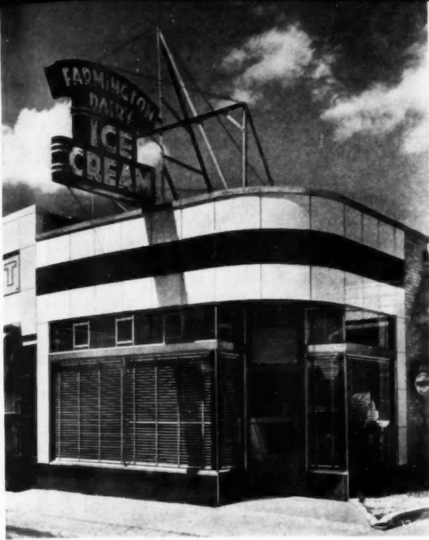
LEFT AND BELOW: Two examples of store construction using glastone units; brilliant and attractive color combinations are possible with the vitrolite facing used on this newly developed material.
