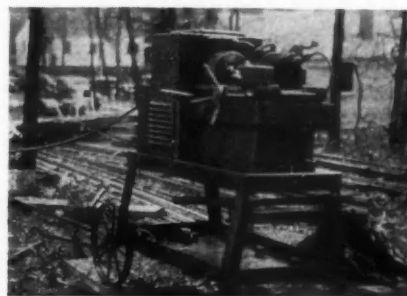
ELECTRIC pipe cutter set up on job.
