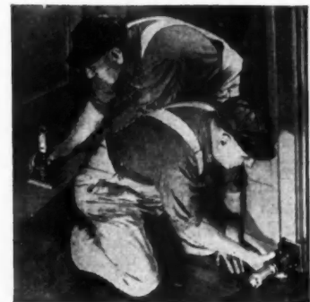
WORKMEN using new portable electric sanders on the hard-to-reach spots.
