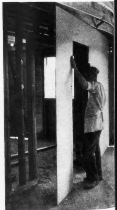
LEFT: Workman applying Upson Floating Fasteners to the studs; these anchor the panel from the back.
