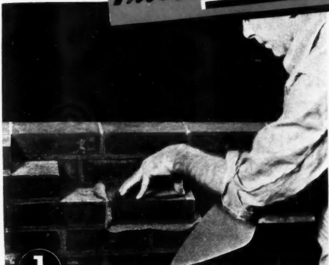
1 Take some Brixment mortar and some mortar made with lime and cement. Try shoving a full head-joint with each mortar. You'll find that with the Brixment
