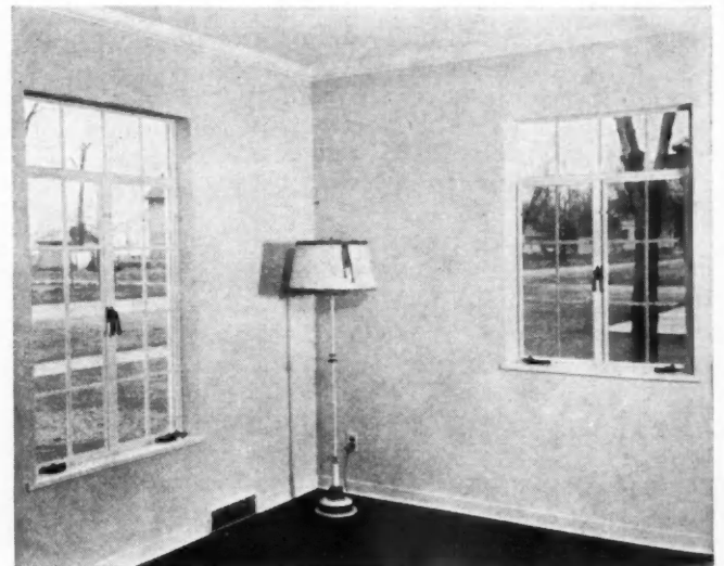
CORNER of living room shows modern, trim appearance with small size steel base and cove mouldings around steel casements.
