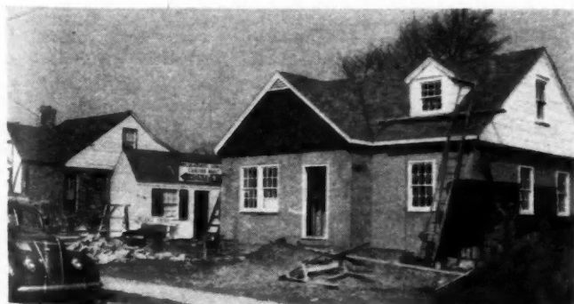
INSULATING board sheathing is used on all Bruggemann and Schafer houses, providing a warm, dry and well insulated house.
