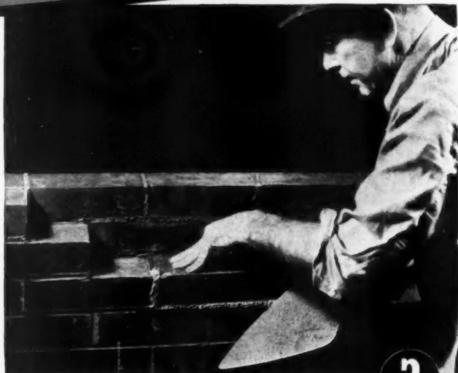
mortar (1), it is much easier to shove the brick accurately into place, with a full head-joint, than it is to do the same thing with the other mortar (2).
