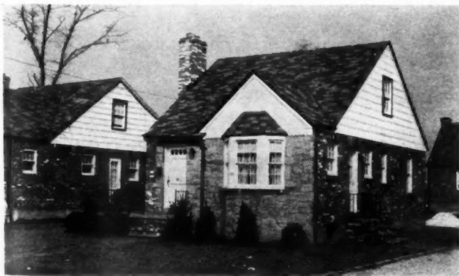
BRICK, stone and asbestos shingles are combined in this typical Bruggemann and Schafer exterior.
