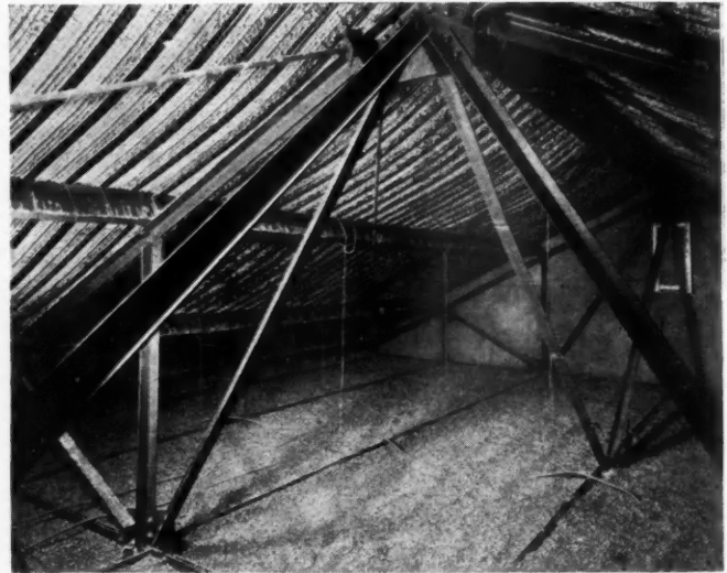
ABOVE, roof bracing and construction, concrete stucco and insulation in the E. R. Haack home, Sheboygan. BELOW, detail of framed door opening and side wall construction.
