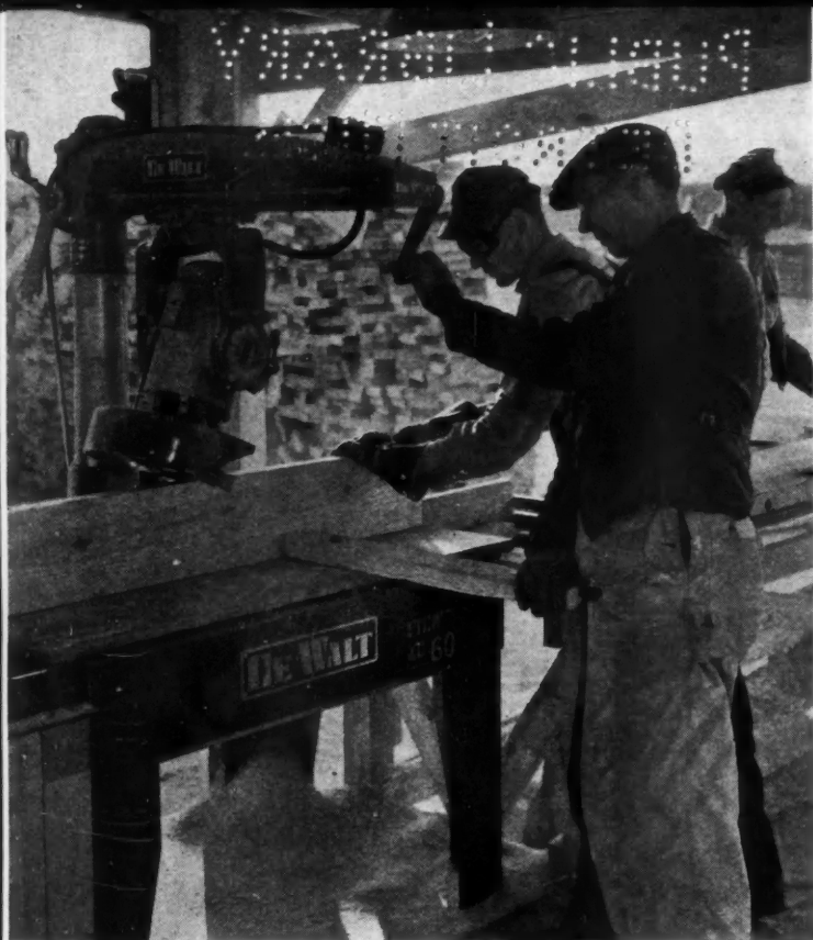
SPECIAL HEEL CUTTING HEAD on saw at Ellington Field, Texas. Multiple saw layout, arranged as in diagram below, speeds cutting.
