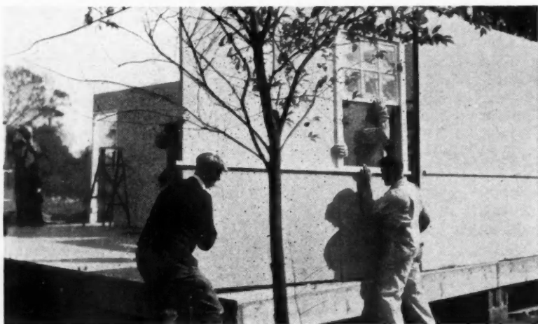
WALL SECTIONS of insulating board glued to 2-in. studs fit snugly together and are held in place by metal clips screwed to floor sections. Sections were built in nearby lumber yard.
