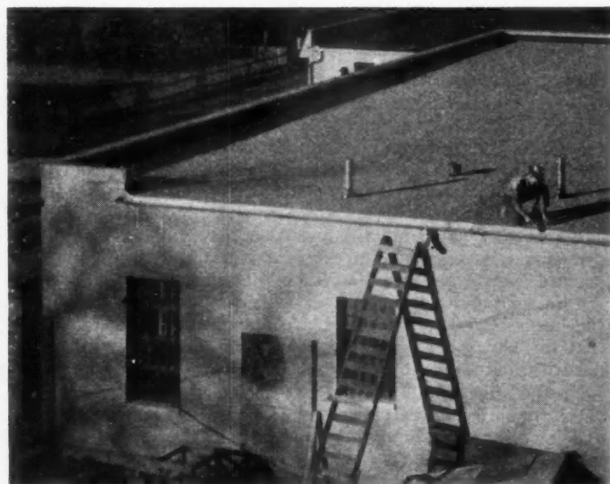
WORKMAN installing stainless steel gutters on new garage of Ohio
