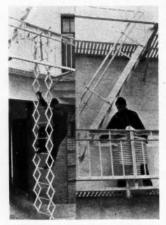
"SAFEXIT" in lowered position and (at right) retracted when not in use.
