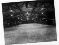
Floor designed, laid in mastic over concrete, by Cincinnati Floor Company, Flooring was lateralnailed and rolled with beavy roller before sanding. Result is a remarkably level, smooth and quiet roller rink floor.
