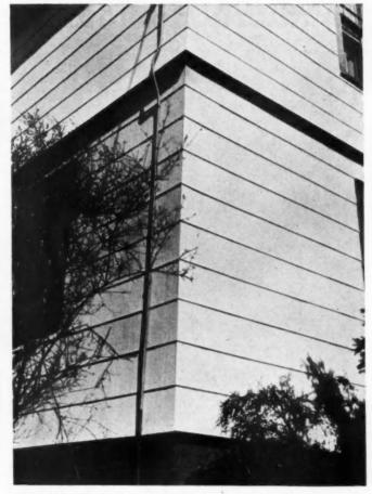
ASBESTOS sidings are lapped alternately at corners over the metal corner strip used on this job.
