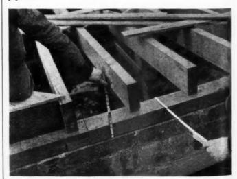
SEASONED substantial framing is used as illustrated in this photograph, showing  $4 \times 6$  notched and lapped sill and  $3 \times 8$  joists.
