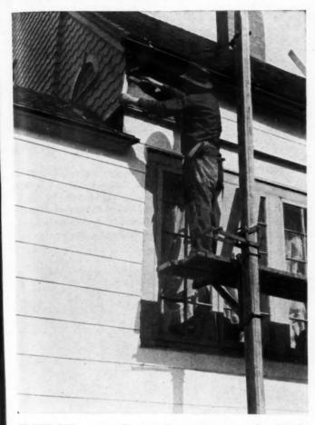
ON THIS JOB non-corroding metal corners were used under the asbestos sidings, both outside and inside corners.
