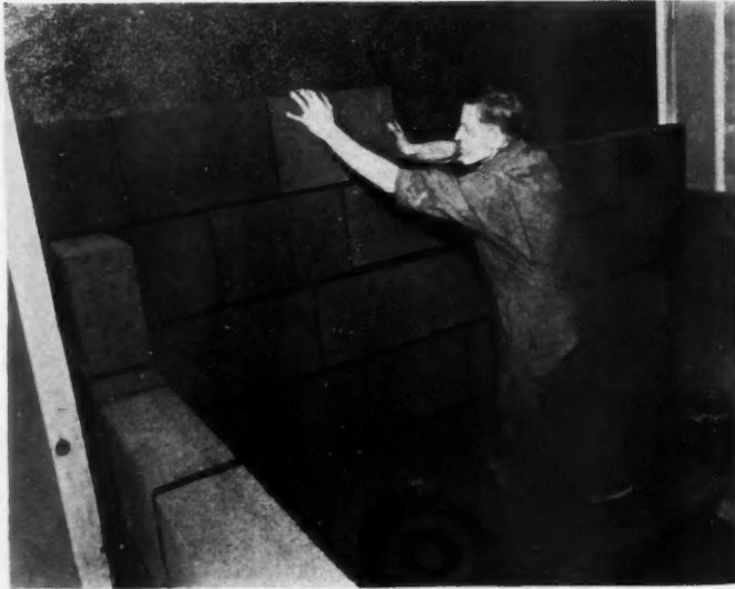
ARMSTRONG'S Foamglas insulation offers glass in a form which can be sawed and worked with ordinary tools. Shown is a worker sawing a block of Foamglas in a mitre box. ABOVE: A workman is erecting Foamglas insulation on a wall of a refrigerated room.
