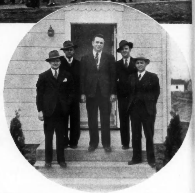
MEMBERS of Bradford organization are, left to right: William Hofar, priorities man; Ellis Ray, concrete foreman; Gale Bradford, president, Bradford Homes, Inc.; Kenneth K. Jackson, manager, Bradford Homes, Inc.; Edward Henager, carpenter contractor.
