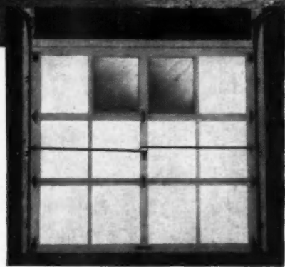
View of Door from inside of Garage
