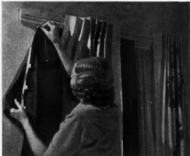
TAKING the place of metal curtain rods, Jiffy slotted wood mouldings serve both decorative and blackout purposes. First a special slider tape is sewed to the top of curtains. Then each little slider is inserted into slot through small aperture near end of moulding.
