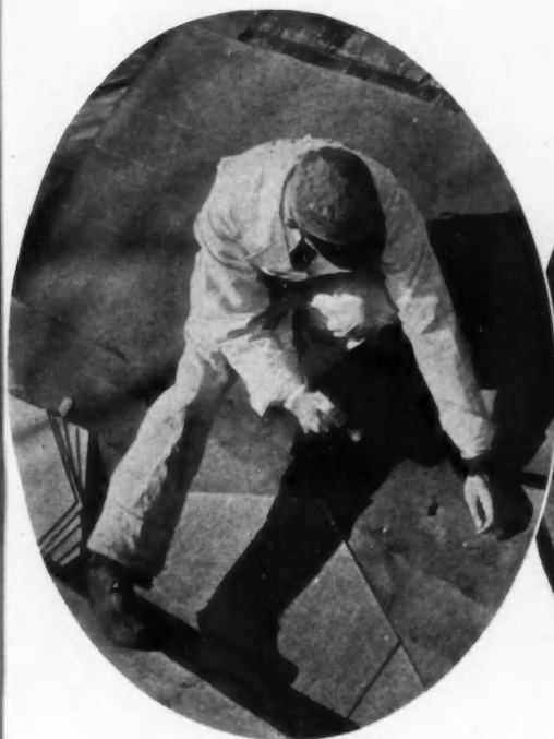
SELL reroofing jobs.
