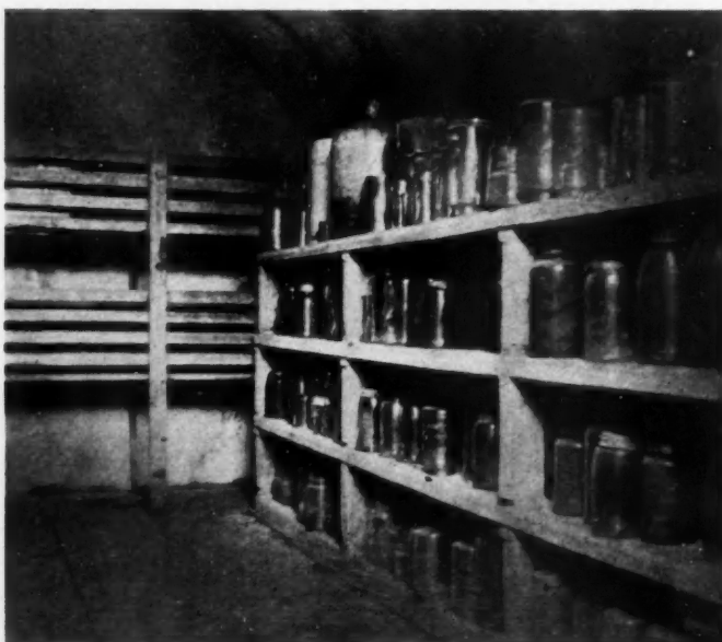
THIS concrete underground storage cellar, built near Wilmington, Ohio, has served well since 1915.
