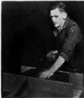
ARMSTRONG'S Foamglas insulation offers glass in a form which can be sawed and worked with ordinary tools. Shown is a worker sawing a block of Foamglas in a mitre box. ABOVE: A workman is erecting Foamglas insulation on a wall of a refrigerated room.
