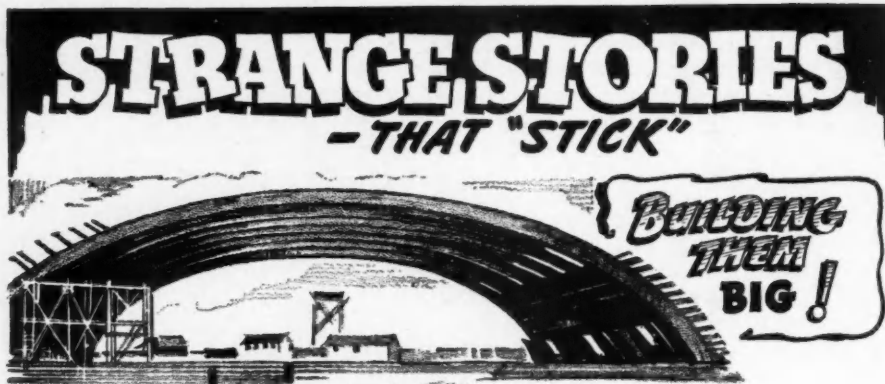
LAUCKS GLUES WERE USED IN THE CONSTRUCTION OF 152 FOOT BEAMS ON A HANGAR AT GRAND FORKS, N. D.
