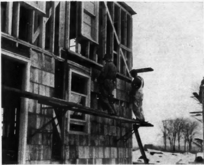
SHINGLE panels—complete with insulation board, building paper, and shingles—are applied on the job by nailing to each stud bearing. The panels are easily handled by two men.
