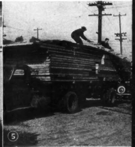
PREFABCO houses in the making: (1) Frame comes out of jig; (2) insulation in place on ceiling panel, glue being applied; (3) plywood face being put on as panel moves down production line; (4) floor sections ready for the job, finish applied; (5) loading, "a house to a truck"; (6) erecting on site; (construction details and site view on next page).
