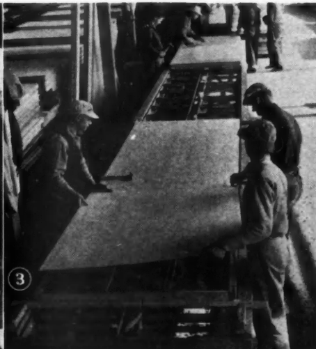
PREFABCO houses in the making: (1) Frame comes out of jig; (2) insulation in place on ceiling panel, glue being applied; (3) plywood face being put on as panel moves down production line; (4) floor sections ready for the job, finish applied; (5) loading, "a house to a truck"; (6) erecting on site; (construction details and site view on next page).
