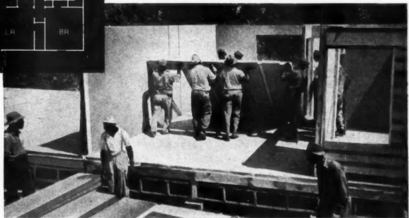
PICTURED AT TOP. Low-cost Homasote Home constructed on the Precision-Built Jr. Method . . . LEFT. Basic floor plan of low-cost, two-bedroom home . . . BELOW. Crew assembling walls and partitions at the site.
