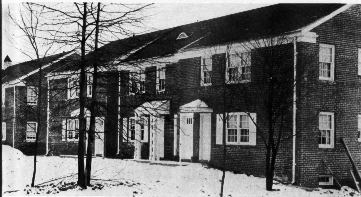
ABOVE: Construction view of some of the six-apartment units in Rahway Gardens war housing project. Typical plans of one- and two-bedroom apartments are shown at right. Notice separate entrance to both first and second floors, instead of common vestibule.
