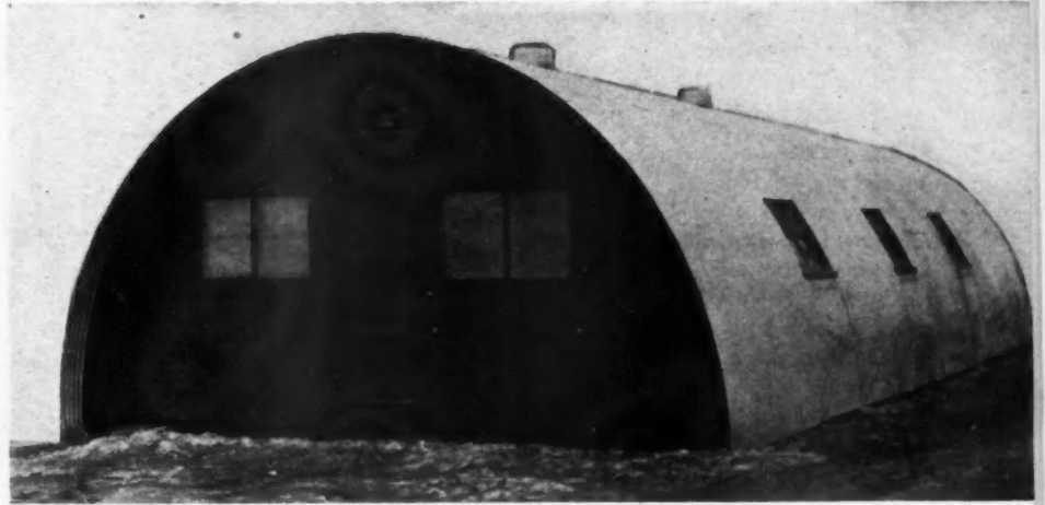
Factory-built Navy hut 20 by 48 by 10 feet in size, of type shipped all over the world to house fighting forces. Exterior is of insulated sheets on a Stran-Steel frame; ends are of double plywood wall construction with insulation placed as in drawing below.
