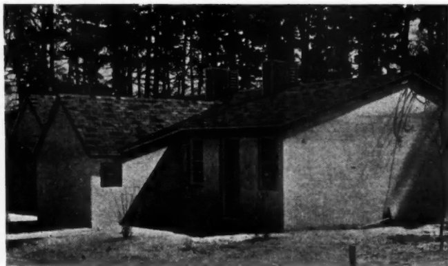
CONSTRUCTION VIEW of one end of row of Levitt's cinder block houses. Units are 21 x 30 feet; carry $2850 mortgage; rent for $33.
