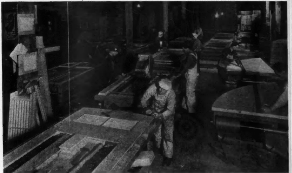
Labor-saving assembly tables, jigs and power equipment speed production of plywood end panels for Navy huts in West Coast plant. Plywood is glued and nailed to light frame of 1 1/2" stock in converted millwork plant as seen in foreground of view above.
