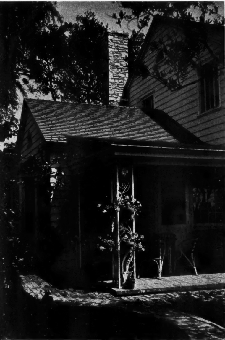
BRICK porch floors should be laid smooth and even so that furniture will be level. Notice brick walk, and portion of circular pool in lower part of the picture, which is faced with brick.
