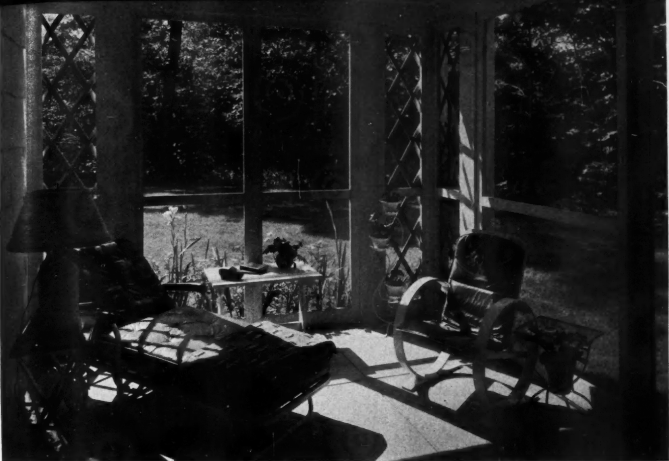
SINCE there is no shortage of concrete, an already roofed-over porch or terrace can easily be turned into an outdoor living room, usable at almost any time, by first laying a concrete floor. The areas to be screened in a porch of this type are small. Lattice work at the outside corners, later covered with climbing vines, provides shade and decoration.
