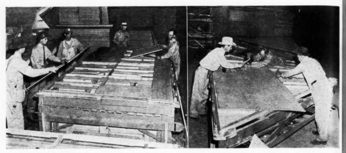
UNION CARPENTERS apply exterior grade plywood over 2" by 2" framing on standard jig tables in Texas plant.
