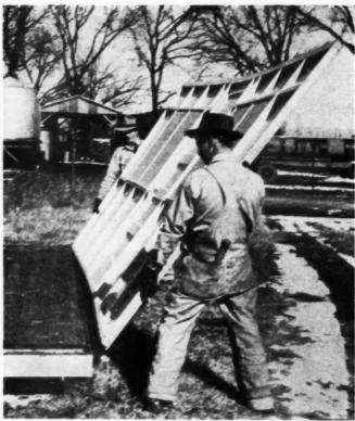
16 FT. WALL SECTION complete with door is handled by two men. Ease of erection has been tested on all war fronts.
