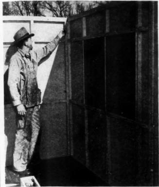
"VICTORY" units are quickly bolted together, as quickly taken apart. Crew of six can erect house in 1 hour.
