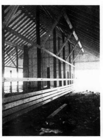
STEPS IN ERECTING a pole & rafter barn. Left, workmen set the butt-treated poles plumb, on concrete footing pads; then cut off tops to desired height, as shown above. Braces, side girts, rafters, and outside covering are added as shown in photos to right.
