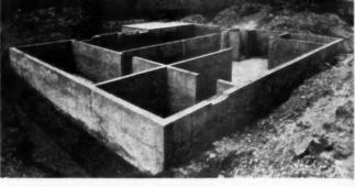
TYPICAL poured concrete basement walls during construction. Note water standing around outside; wall showed no leakage. Drain tile around footing will carry the water away from the foundation.
