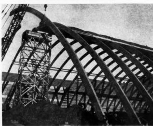
Example of Laminated Timber Arch Construction, Span 170 ft. Photo Courtesy Unit Structures, Inc., Peshtigo, Wisc.
