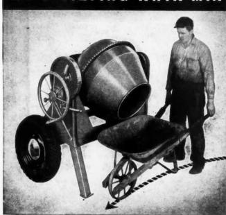
End discharge Air-cooled engine Light weight Welded construction
