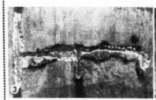
Wire mesh fastened over reinforcing.
