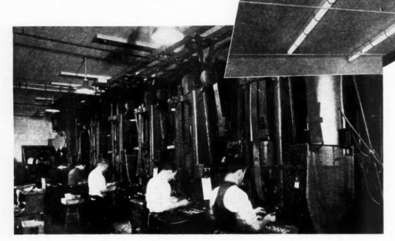
GOOD lighting and a low noise level increase war plant efficiency. Ceiling above shows proper installation to provide both items.
