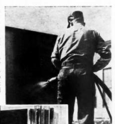
WORKMAN, above, applying pneumatically shot concrete to test panel: Colburn system model is
