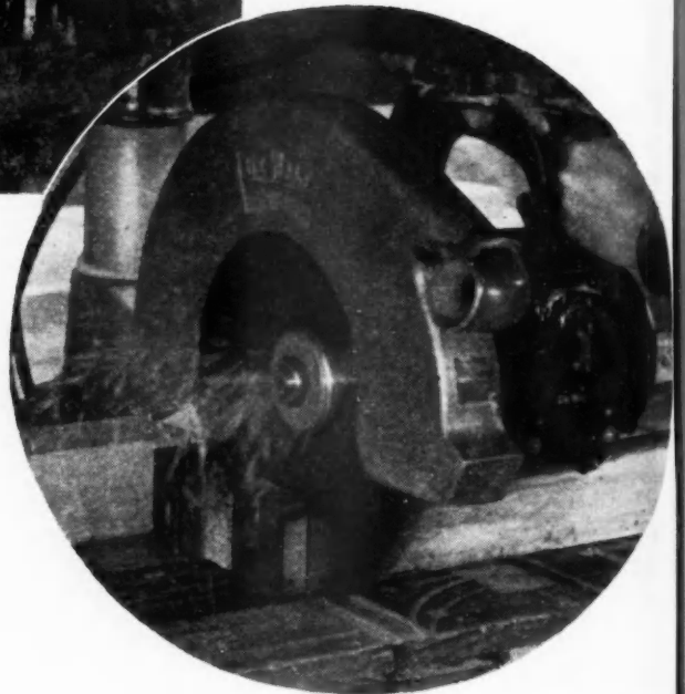
LEFT: Large military camp project under construction; pre-cutting shed and lumber stock pile in left background, pre-cut members in foreground, barracks in right background. Below, multiple squaring of studding on saw.
