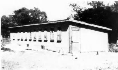
Laying house on farm in Minnesota, with walls constructed with multiple-function Celo-Siding.
