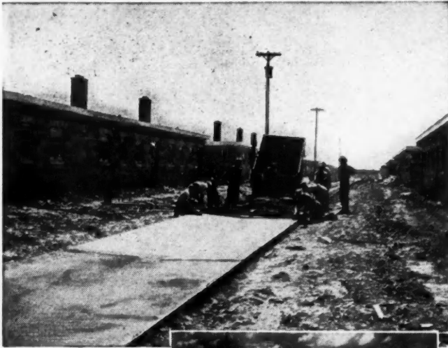
Building concrete lane at housing project for Naval Ordnance Depot workers in Nebraska.
