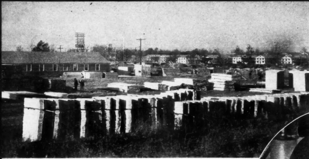
LEFT: Large military camp project under construction; pre-cutting shed and lumber stock pile in left background, pre-cut members in foreground, barracks in right background. Below, multiple squaring of studding on saw.
