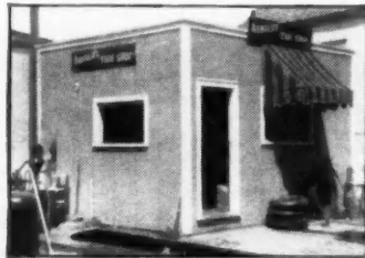
Small wartime tire shop with exterior walls of Celo-Siding.
