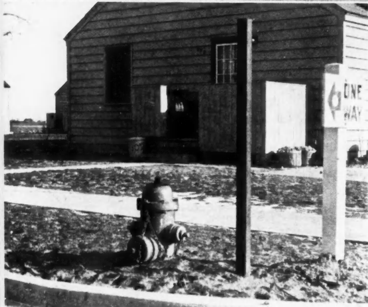
BLIGHTING beautiful Sheridan Parkside, coal bin, garbage and ash cans at front door demoralize war workers, drive them house hunting endlessly. Fire hazard protested by firemen unable to attach hose to hydrant off grade. GOVERNMENT planned to keep war workers contented are the projects pictured above.
