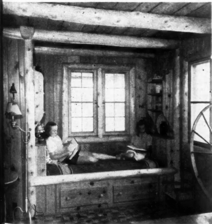
BUILT-IN bunk with rustic log trim and drawers below make pleasant corner. How to build bunk is shown in drawings on page 61.
