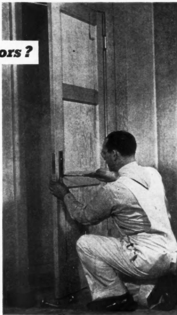
CARPENTER quickly applies hardware to factory machined door as shown here.
