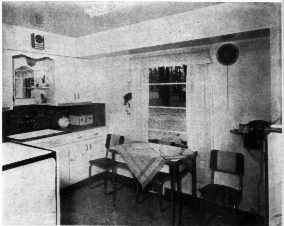
THE kitchen shown in the photograph above is typical of the houses under construction as pictured at the top of the page. Built under title VI of FHA, the kitchens of these houses are fully equipped, including ventilator, package receiver, fluorescent lighting and telephone shelf. Toe space is provided and the floor has linoleum cove base.
