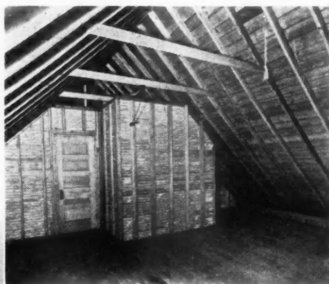
THE bare attic space before "face lifting."
