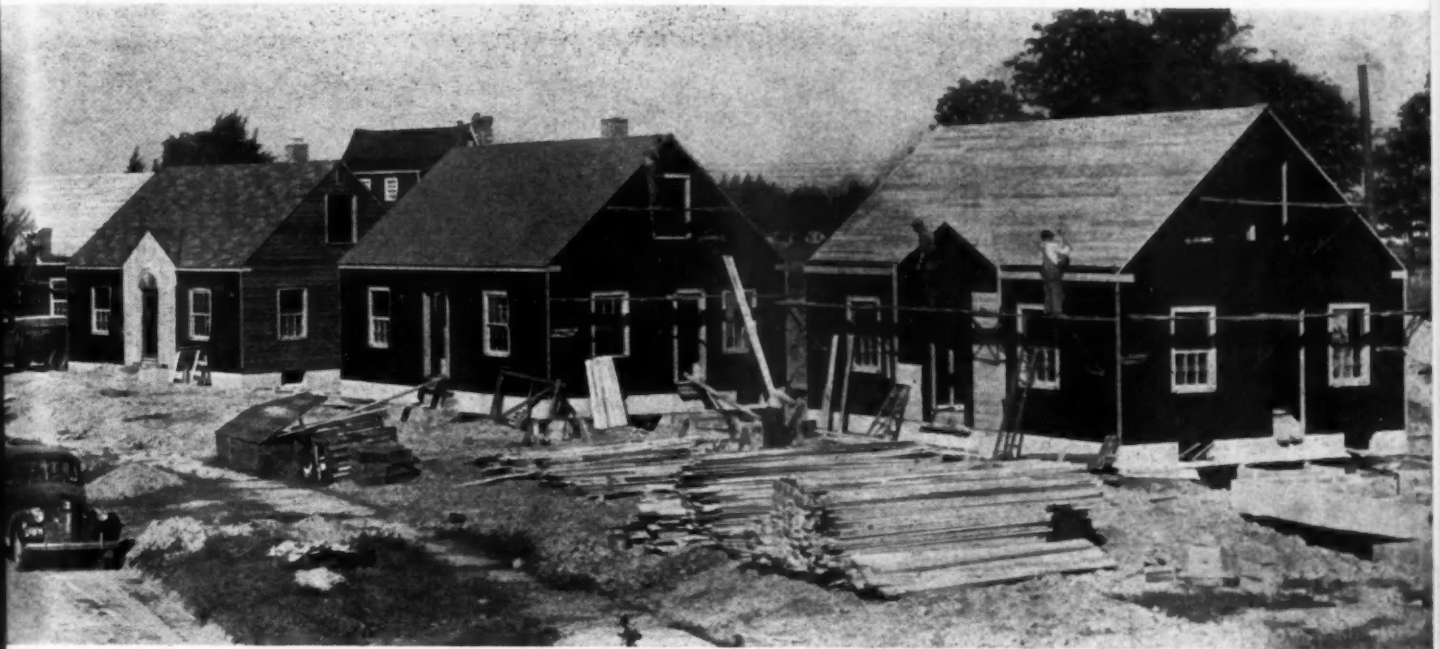
ABOVE is a view of one of the Gerholz Healy Company's war housing streets showing the desirable effect obtained with varying set-backs.
