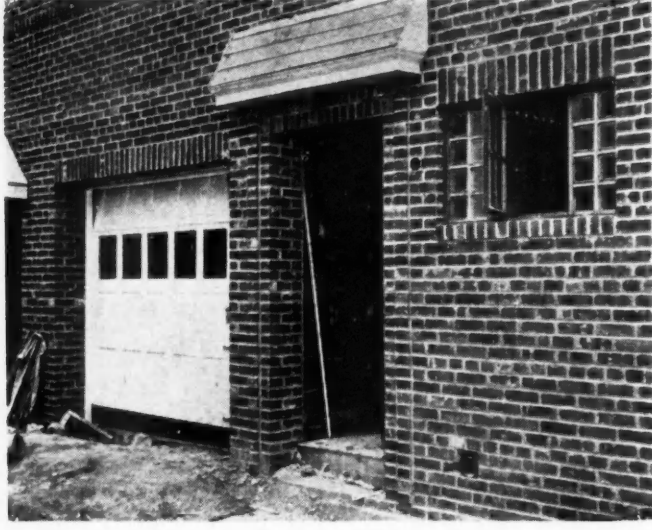
GARAGE door and main entrance dominate first-floor elevation.
