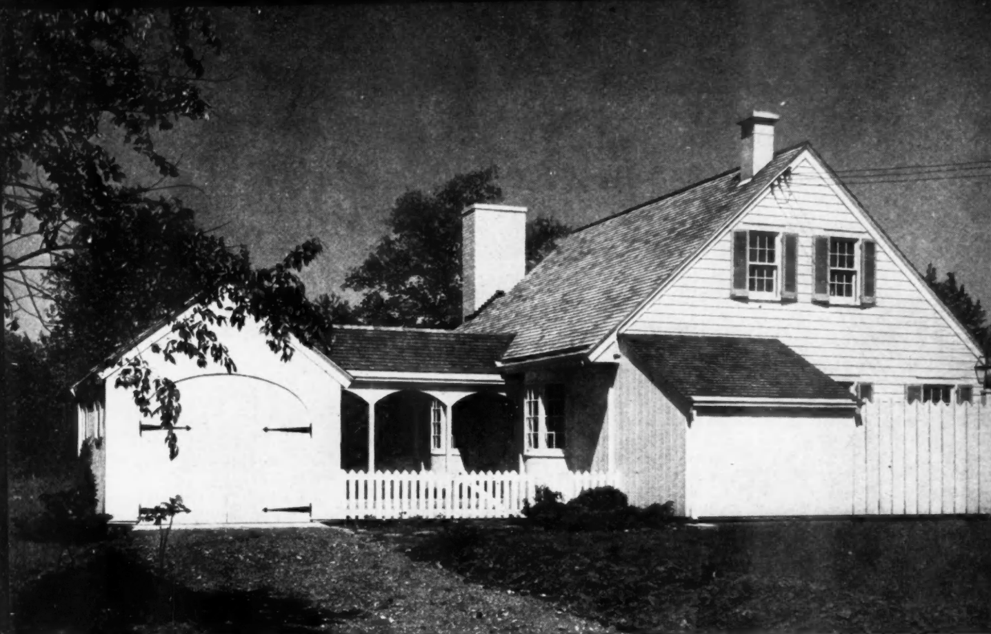
THE simplicity, charm and beauty associated with early Colonial architecture are captured in this distinctive two-story Cape Cod.
