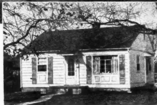
. . . NATIONAL HOMES CORPORATION, LAFAYETTE, INDIANA
