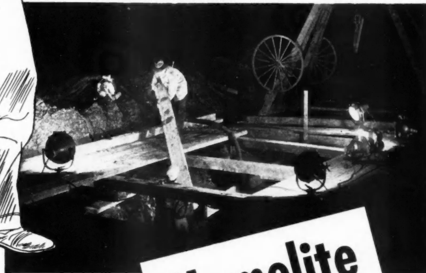
Below — A Homelite Pump and Generator make the right combination for speeding dewatering jobs at night.
