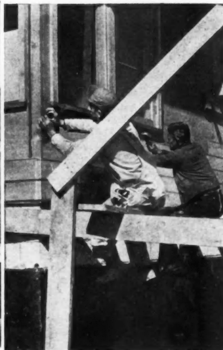
WORKMEN are applying aluminum roofing. Installation of aluminum siding is complete. ALUMINUM siding in process of application.
