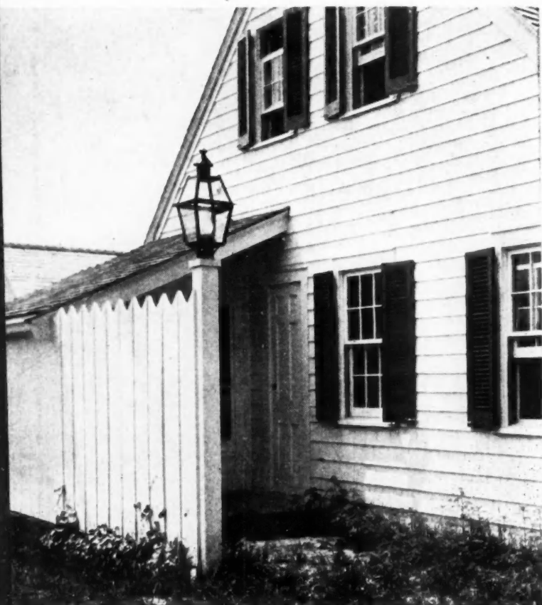
TREATMENT of the rear entry is characteristically Colonial.
