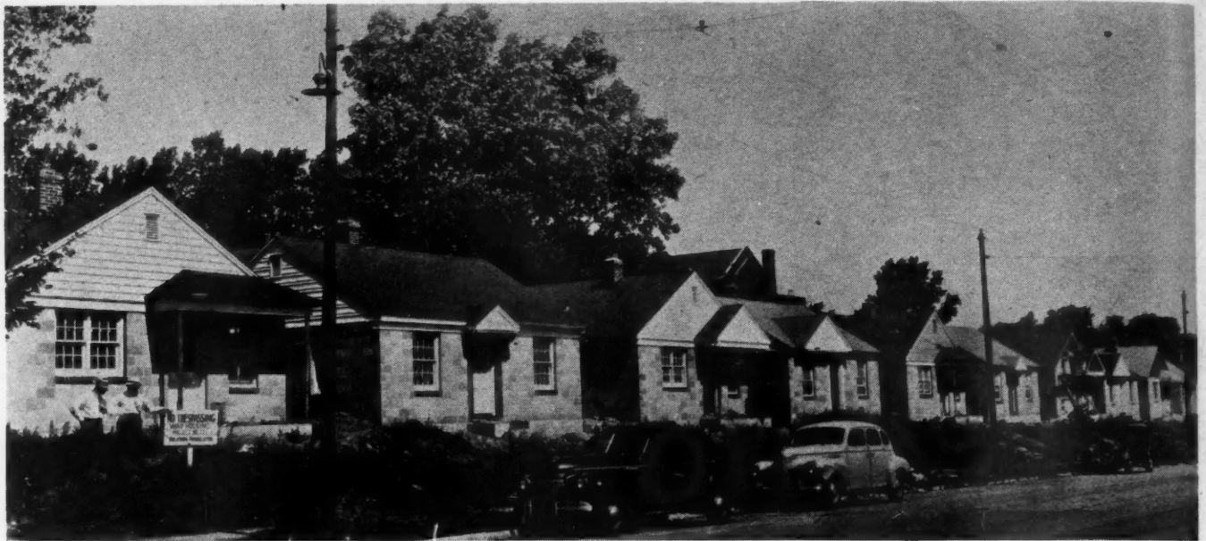
HOUSES in Kansas City, Mo., built with Haydite blocks made with Universal-Atlas Duraplastic air-entraining cement.
