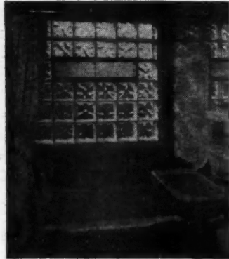
AB27109—The Winco ventilator shown here installed in glass block to provide light along with privacy and ventilation in a bathroom is designed especially for use in glass block. In addition to its adaptability for new home construction it is also fitted for hospitals, stores, offices, etc.
