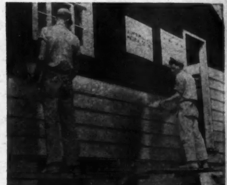
AB2741—Hoess aluminum clapboard siding is manufactured by Metal Building Products, Inc., Detroit. It consists of a section of rolled aluminum sheet, beveled like wood siding and formed to interlock with other sections. Each section is formed with a "U" shaped channel at the bottom. The top edge is rolled over so it interlocks with the "U" channel of section above it.
