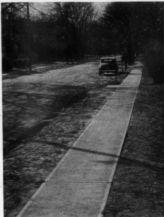
SIDEWALK made with Duraplastic air-entraining Portland cement.
