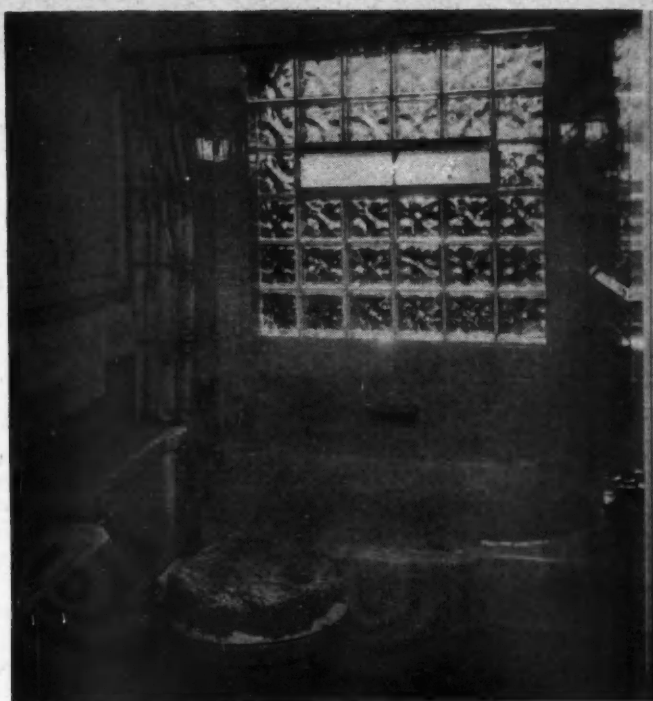
THIS bathroom treatment is standard in Gerholz houses. Glass block provides ample light and Winco ventilator fresh air.
