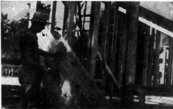
Goes on fast... end joints eliminate trimming at stud and joist centers.
