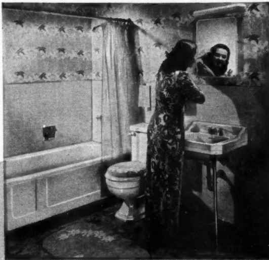
Here is the bathroom side of the Ingersoll Utility Unit installed and in use. Note also the recently installed unit at the right . . . see how neatly kitchen utilities and bath fixtures tie into the central mechanical core.
