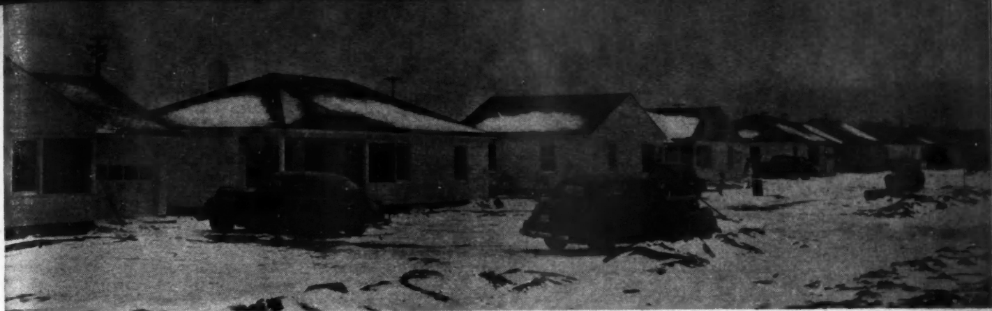
STREET scene of Bulder Payne's G.I. houses under construction showing variety gained by reversing plan and changing roof lines.
