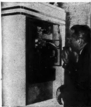
AB2771—This "brain," consisting of the Minneapolis-Honeywell Moduflow system, automatically controls the flow of heat from the Electromode electric furnace, new postwar product for home heating in the TVA area, Pacific Northwest and other regions where low power rates make electric heat practical.
