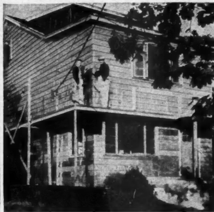
ALUMINUM is used here for re-siding job.
