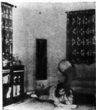
AB2765—A new principle of heating has been employed by Day and Night Mfg. Co., Monrovia, Calif., in Panelray wall heaters. The vented, gas wall heaters radiate infra-red heat. All heater parts are above floor level. They are available in three sizes and in dual models for adjacent rooms.
