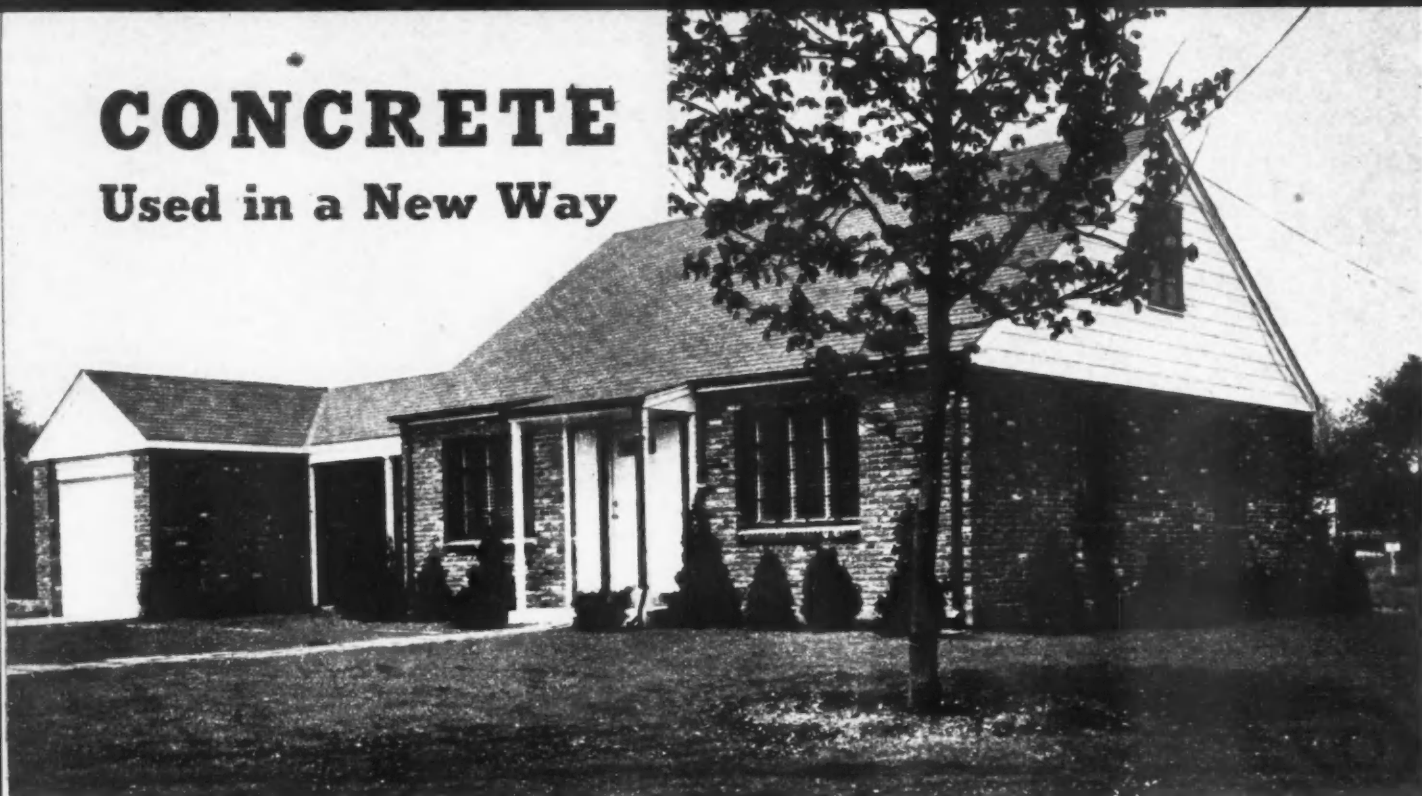
A TYPICAL HOUSE in the North Shore Acre development. Except for the roof and ceiling, the entire house is of fireproof construction.
