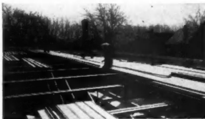
Application of "Ferrobord" Steeldeck
