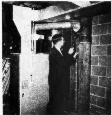
RESEARCH worker is pointing to flue of molded asbestos tile replacing conventional flue.
