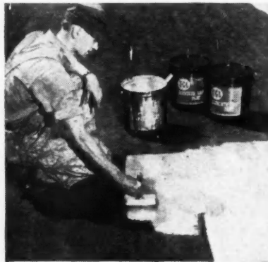
ROOF paint provides low-cost insulation, year-round weatherproofing.
