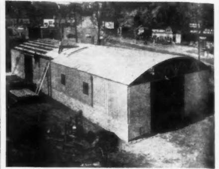
ROOF sheeting laid across faced-in channels.
