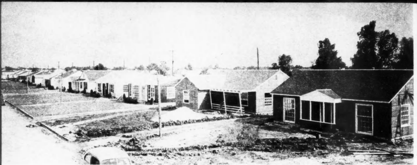
SOUTHERN BUILDERS have found that machines in the plant can do more work than ten men in a conventional on-the-job operation.
