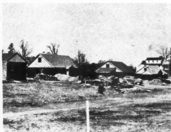
PARTIAL VIEW of the development in an incomplete state.
