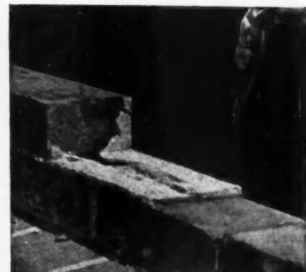
In either case there is not enough mortar in the bed joint to completely fill the furrow.
