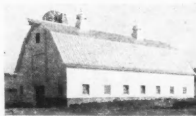
GILSALUME insulates-weatherproofs barn of A. E. Allen, Westfield, N.Y.
