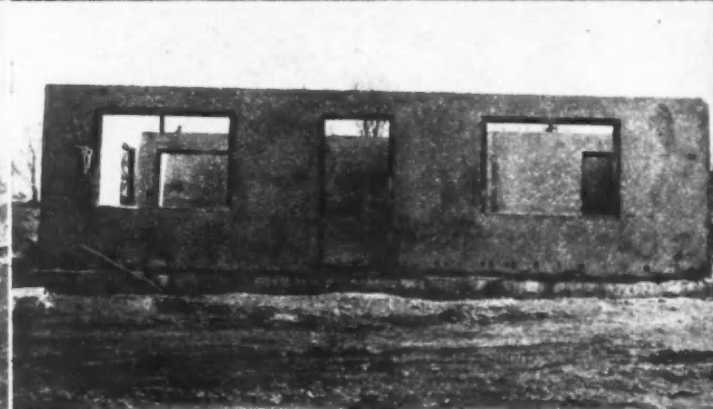
HEAVY power equipment is used to level areas and to hoist steel forms in place. Concrete floor and walls after forms have been removed.
