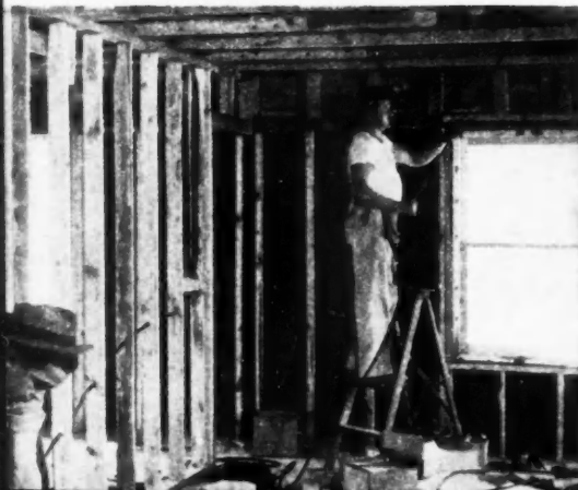
ELECTRIC wiring subcontractor times his work to coincide with interior finishing.
