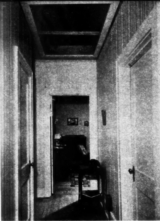
ABOVE LEFT—Opening in hallway ceiling for attic fan. RIGHT: Attic louvers permit free flow of air from attic.
