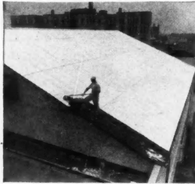
ROOF of Crest Theatre, L.I., N.Y., receives last coat of Gilsalume.
