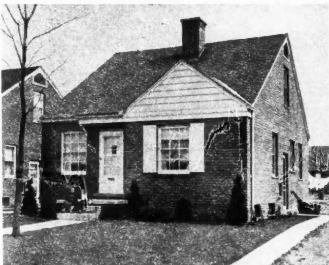
COMPLETED brick veneer house for which wall and roof sections were precut and preassembled with metal jigs in off-site workshop.
