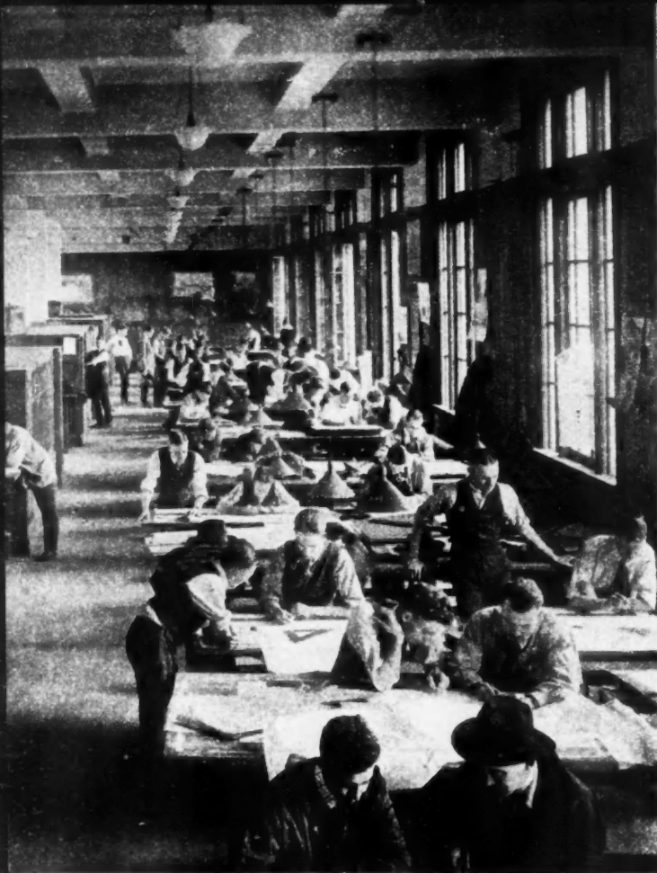
UNIVERSITY classes are making room for young men who plan on entering the building business.
