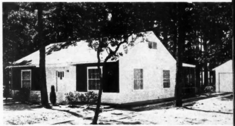
DOORS, windows, louvers, trim, etc., are fabricated, fit in plant.
