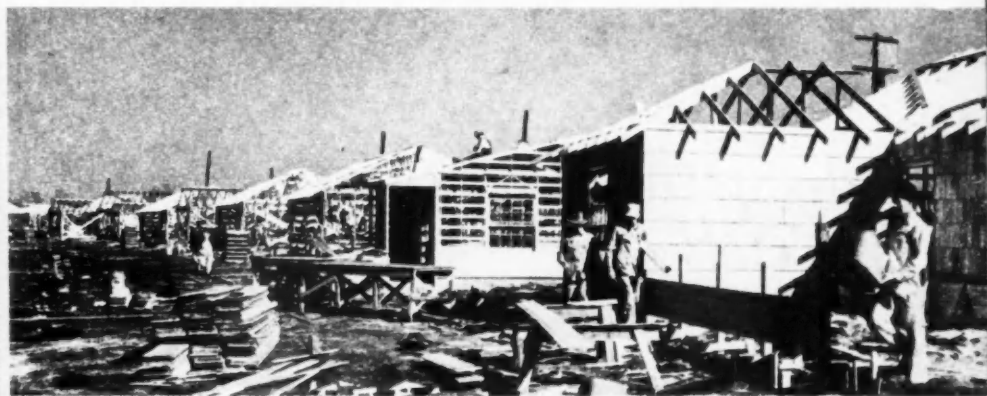
ASSEMBLY line system is used on job site with separate crews doing specialized jobs.
