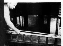
HORIZONTAL mortar joint fixture goes in place atop the first course of block; will be filled with mortar
