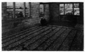
RADIANT floor panel installation going into small office area
