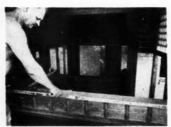
TROWELING become es a simple operation of leveling off the mortar bed. Fixture permits a relatively dry mortar mix
