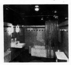
craze or buckle. To install, each individual tile is embedded in a mastic cement to provide a completely waterproof finish for the wall. This tile is produced in a variety of colors, and can be ordered for immediate delivery in small or large quantities.
