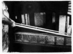
FIXTURE is removed, leaving smooth. continuous bed of mortar stiff enough to prevent "floating" of glass block
